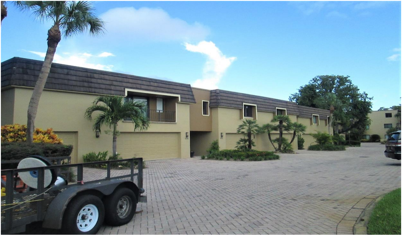
Facing northwest towards front of Condominium Building E
