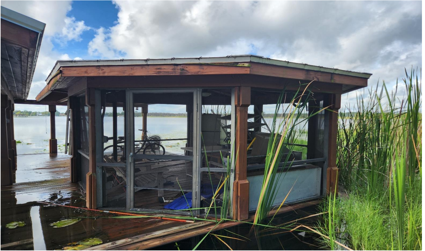
Facing south towards the existing dock to be removed
