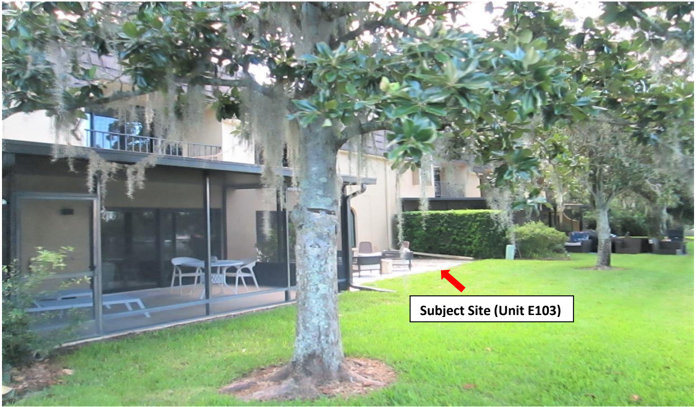
Facing southeast towards existing rear of adjacent condominium units
