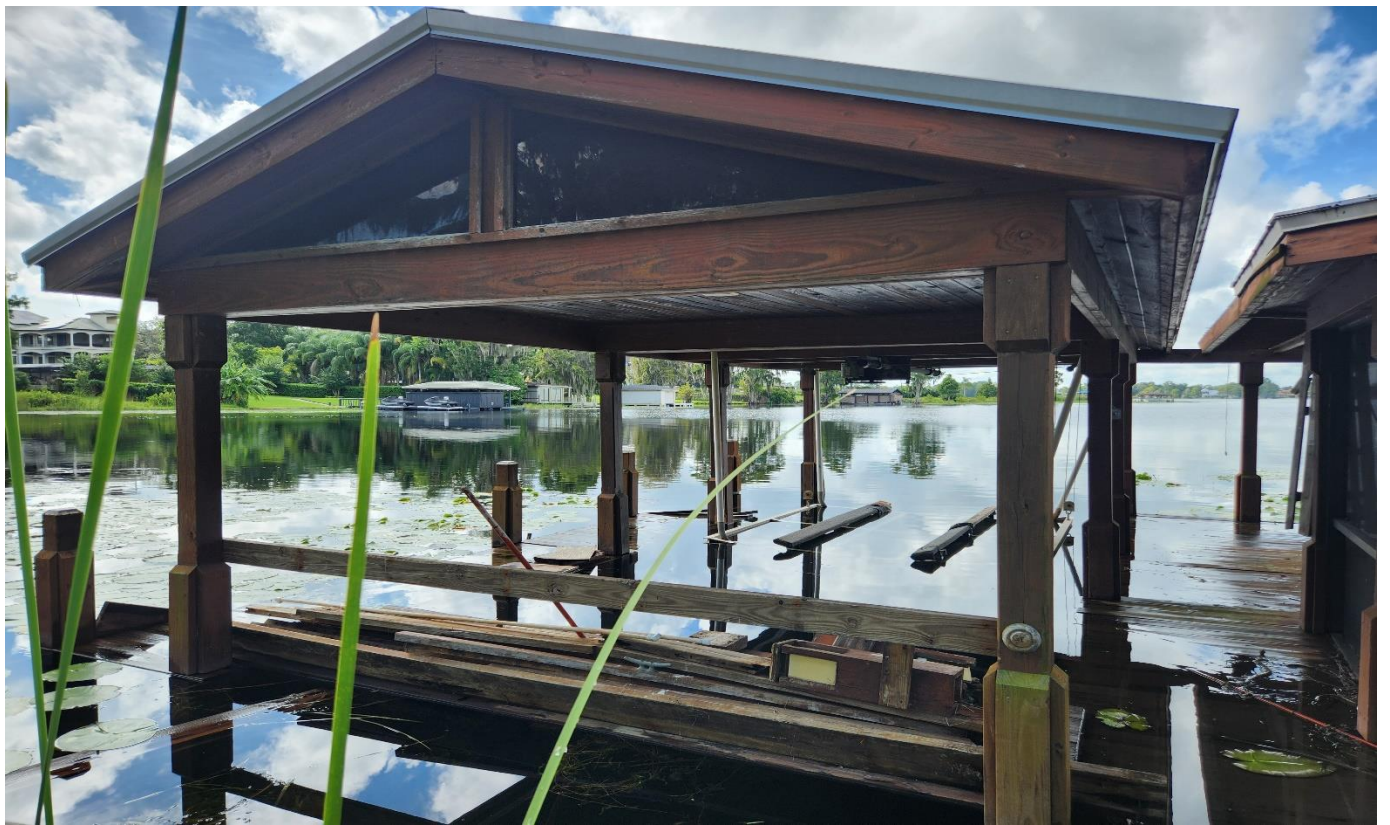
Facing south towards the existing boat dock to be removed
