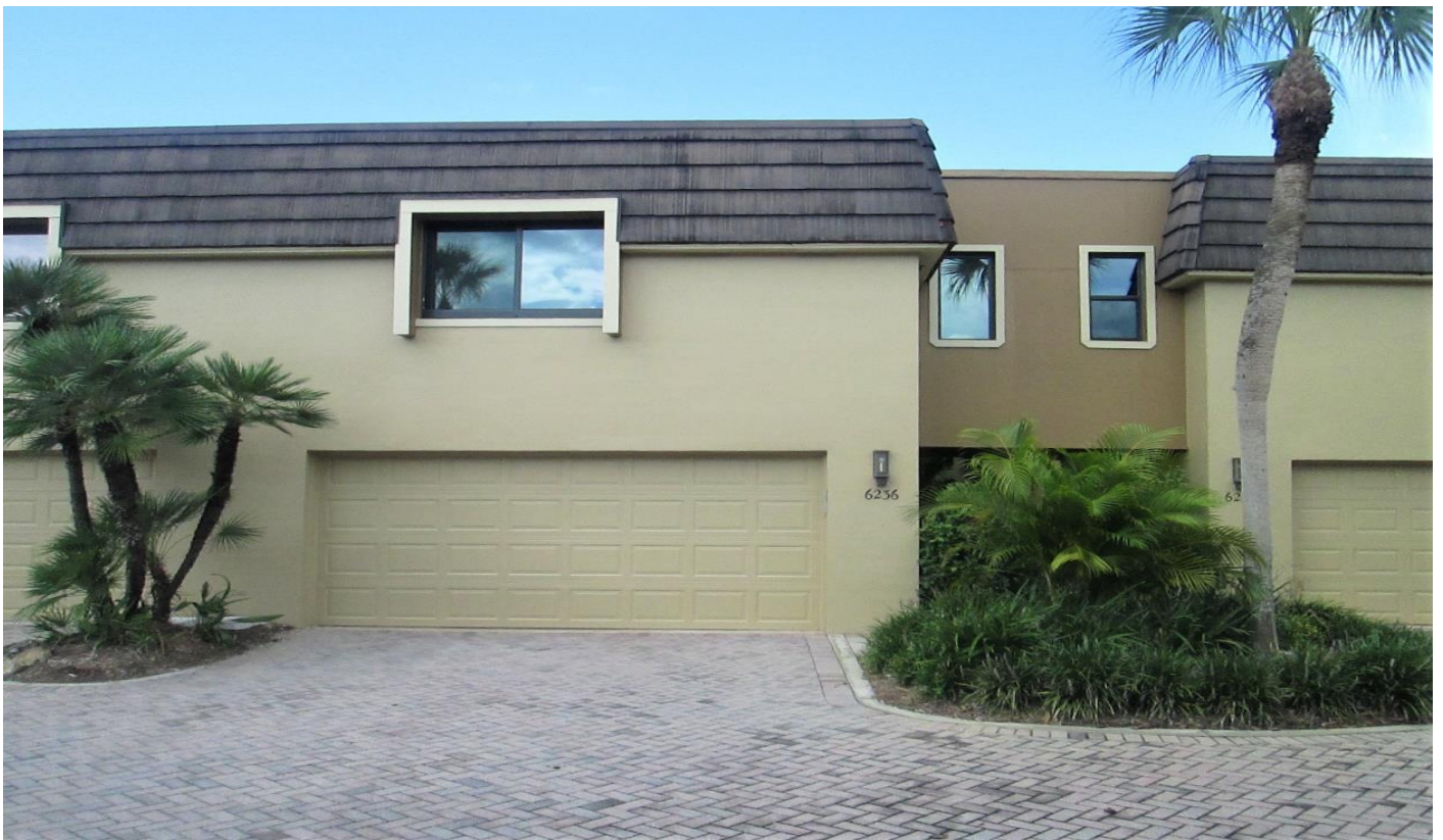
Facing west towards front of subject site (Unit E103)
