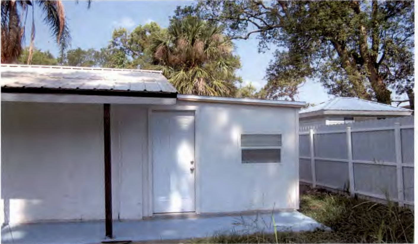
Front yard, west toward front of attached accessory structure
