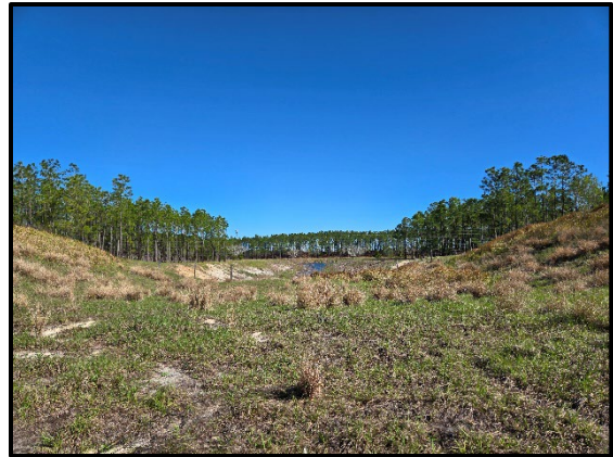
Photo 2.32. Retention pond with sloped berm at the east end of the project corridor north of Hartzog Road, facing north.
