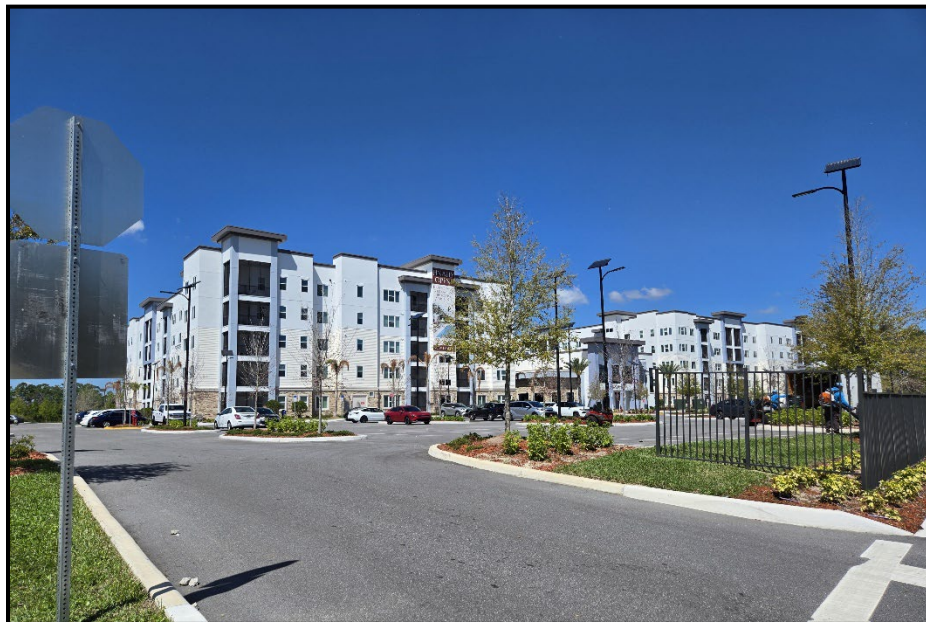
Photo 1. Looking northwest at the former location of the demolished resource (8OR11765).
