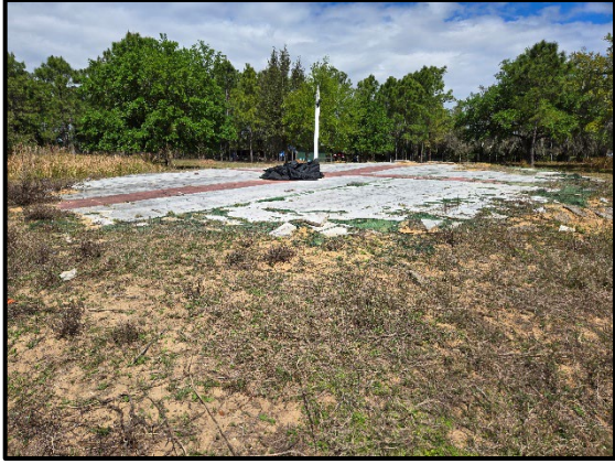
Photo 2.27. Elevated concrete foundation within south portion of FPC 1, facing north.
