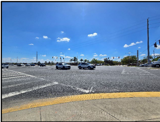
Photo 2.1. Conditions at the Avalon Road/U.S. 192 intersection, facing southeast.
