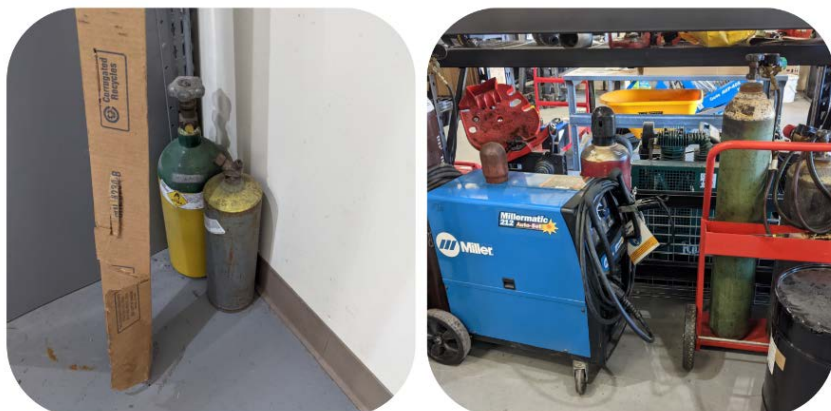
Oxygen and acetylene cylinders were stored within 20 feet of one another.
