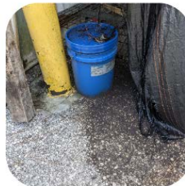
Open used oil container with used oil overflow
