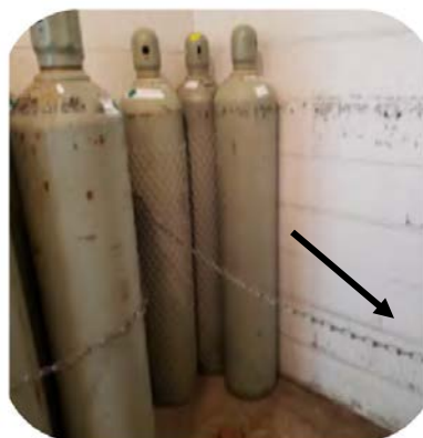
Chains around cylinders may not prevent them from tipping over.
