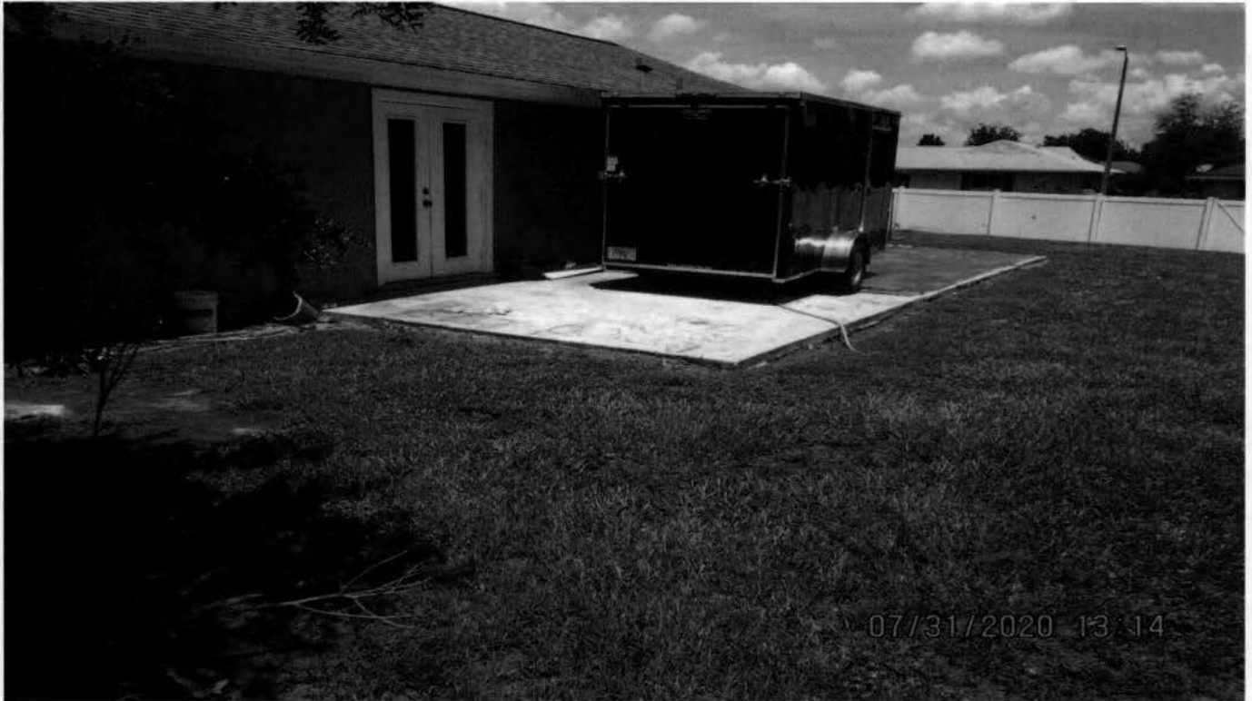
Location of addition in rear yard, looking north
