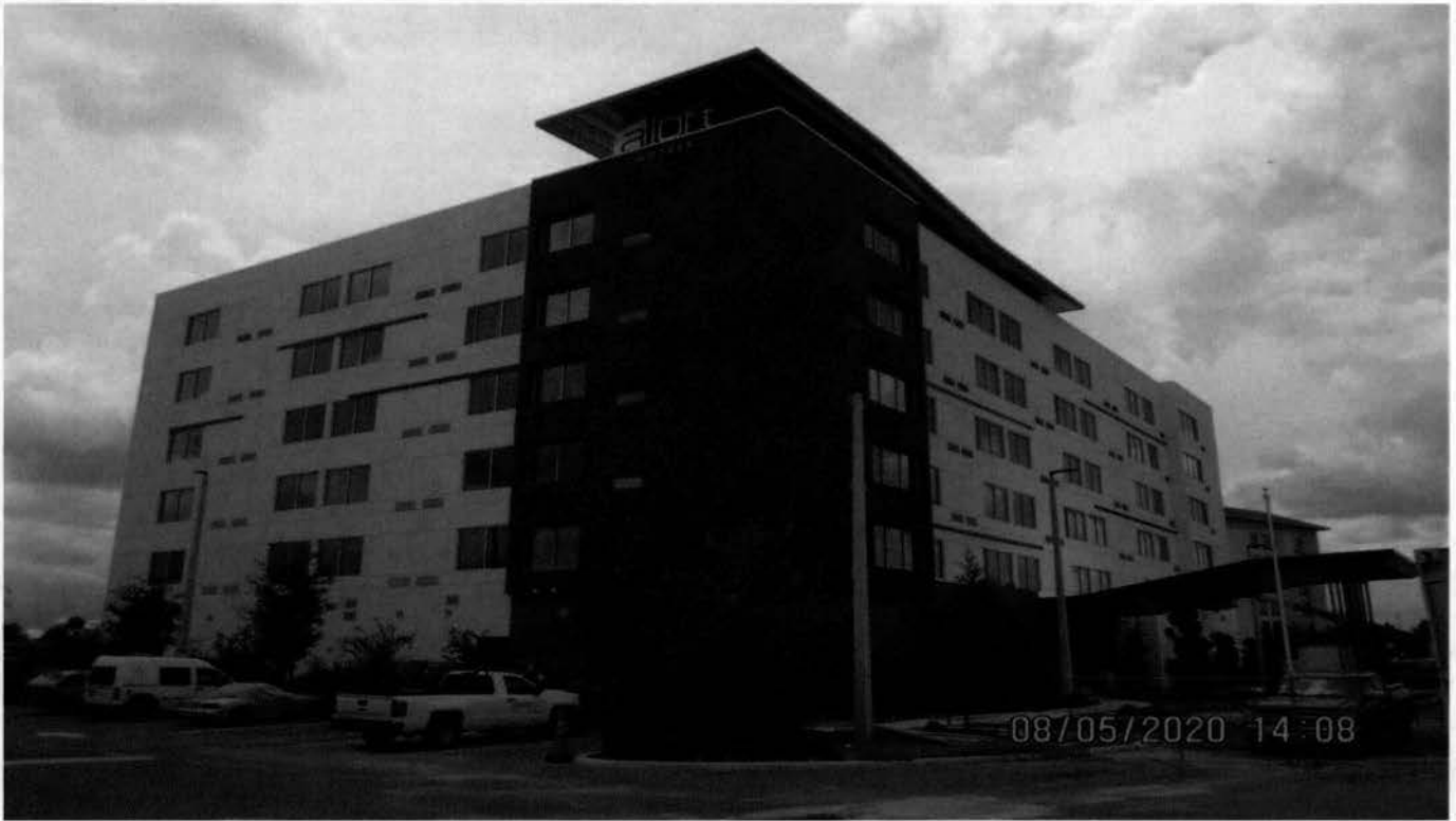
East side sign A (Secondary façade)
