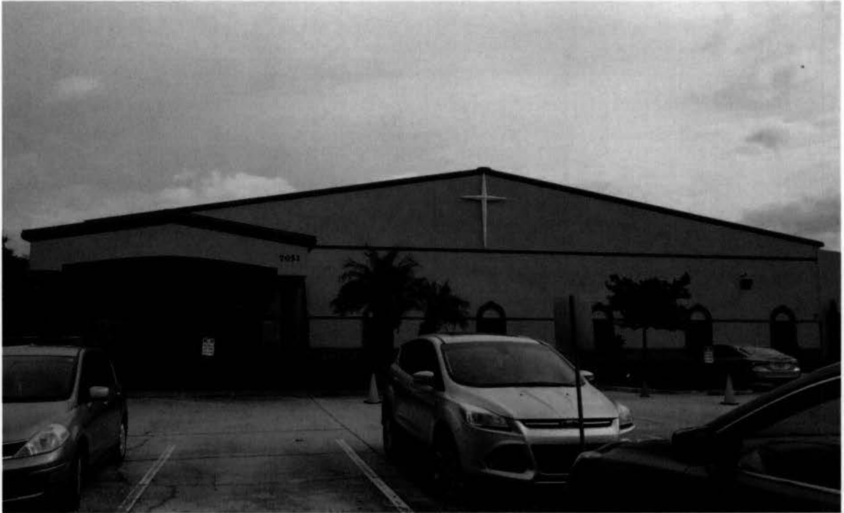
View of front façade facing north towards proposed drop off area enclosure location
