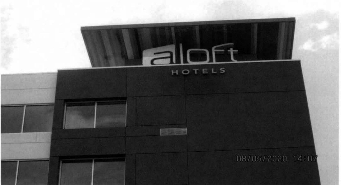
East side sign A (Secondary façade)
