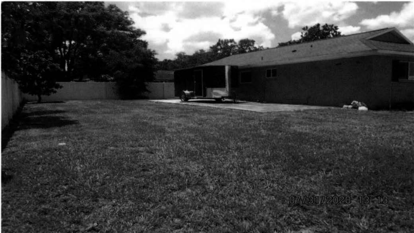
Location of addition in rear yard, looking south
