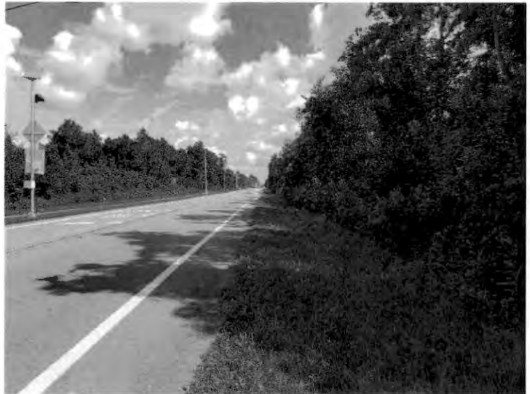
Roadside ditch facing north
