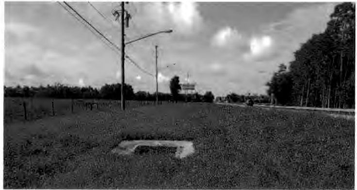
Ditch bottom inlet which conveys sheet flow from Chuluota Road to existing storm drain, facing south
