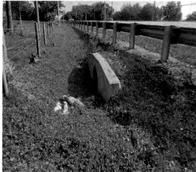
Cross drain which conveys runoff from basin 4-300 to storm drain on east side of Chuluota Road, facing north and east.
