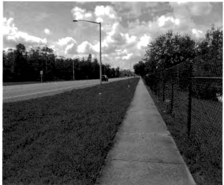
Roadside ditch facing south
