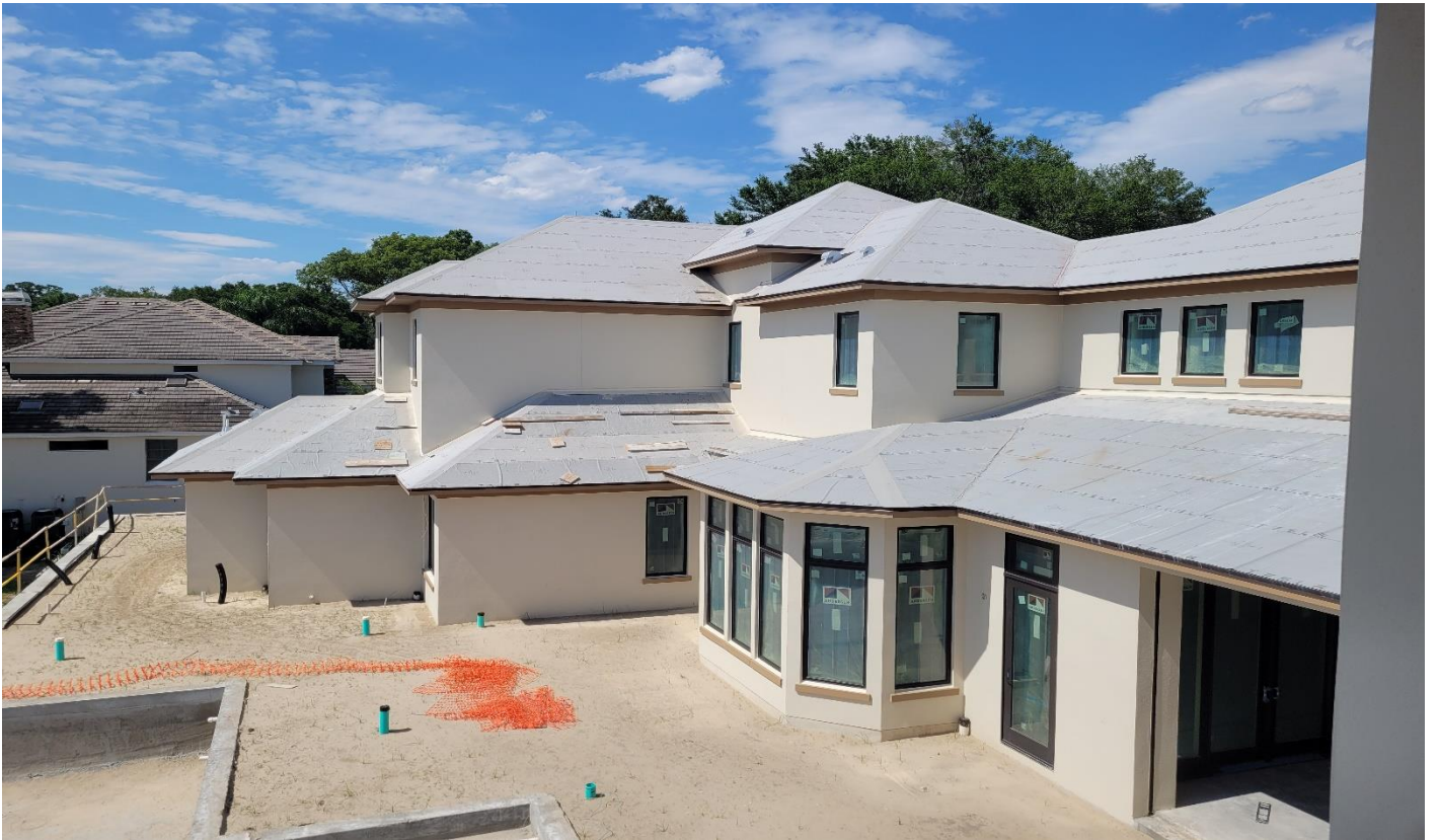
Rear ADU walls, facing north
