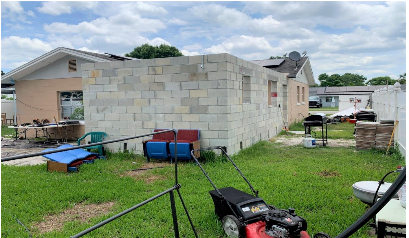
Rear yard, facing east towards proposed addition under construction
