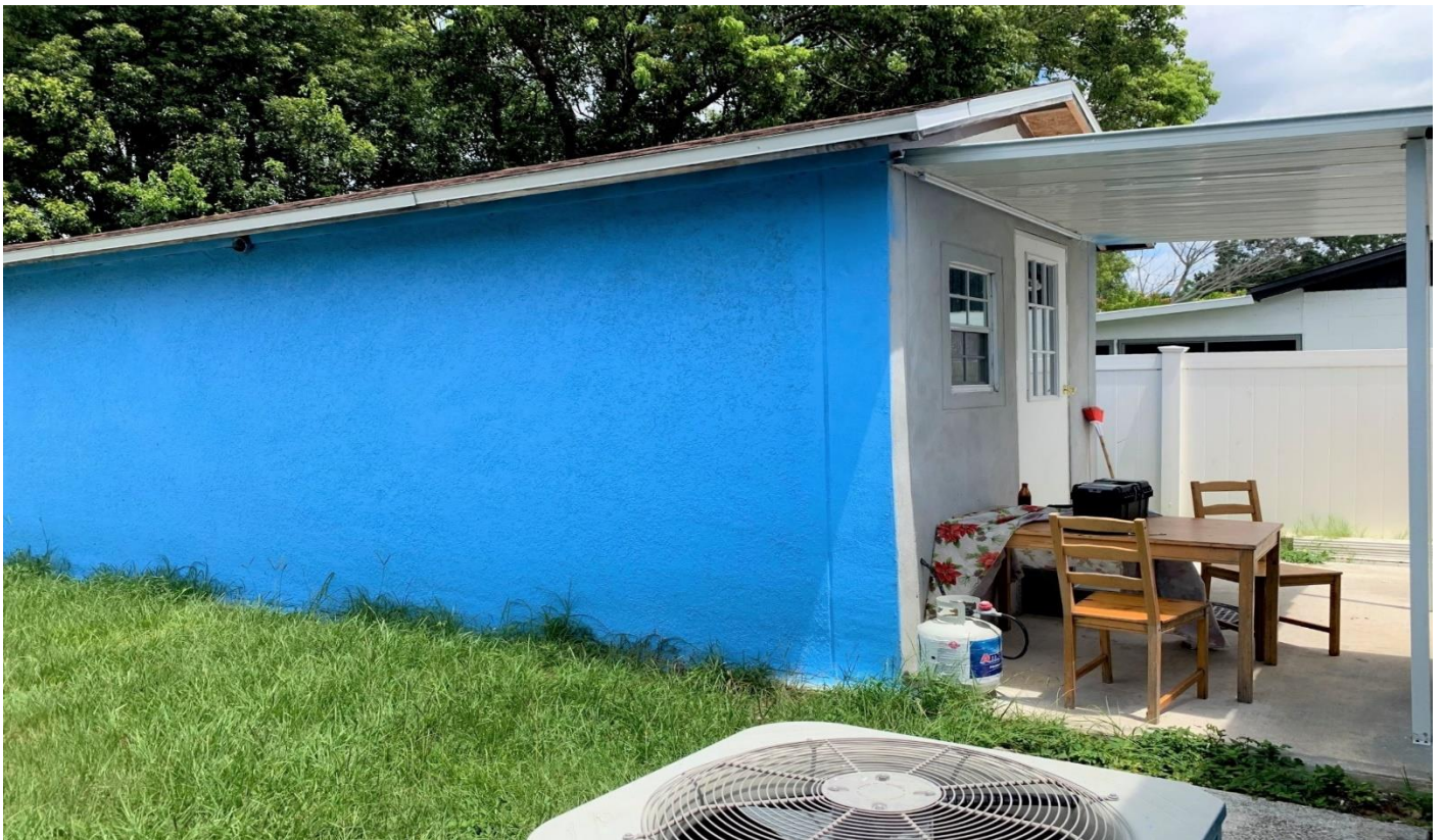
Rear yard, facing north towards existing shed
