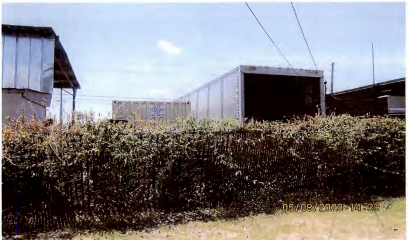
Rear alley, facing west towards Variance #2
