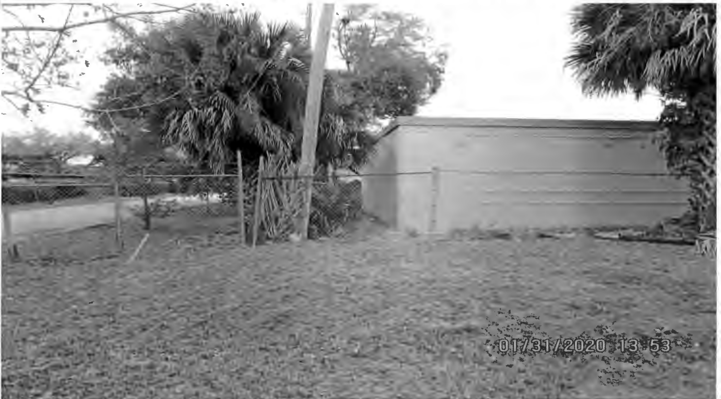
Variance #6; Bldg. H Existing 10.04 ft. Rear Setback in Lieu of 15 ft. Looking North
