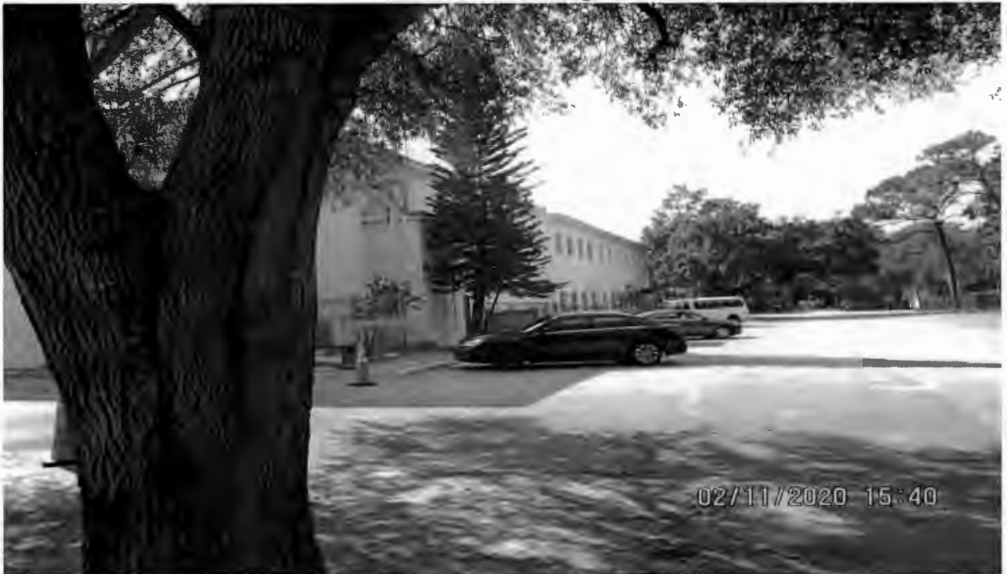
North side of Building with Paved Parking Looking West
