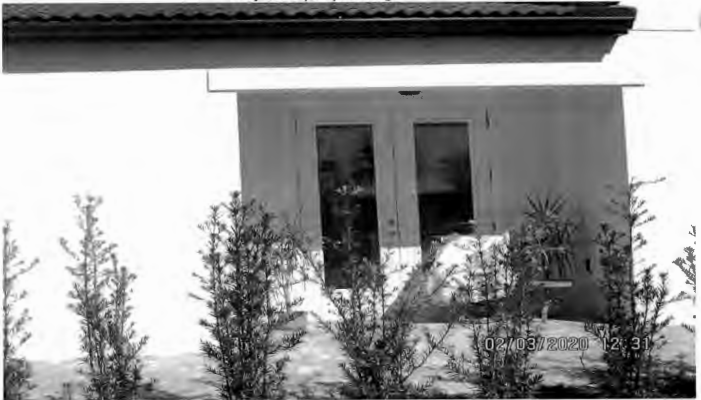
Patio and Kitchen Doors Looking North
