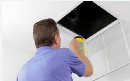
Duct Test & Repair >
