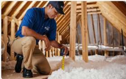
Attic Insulation Upgrade >
