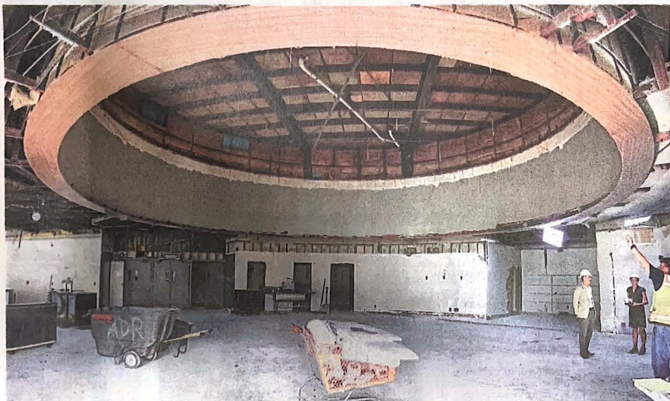
The gutted lobby area is under construction July 24 as part of the multimillion-dollar renovation of the Plaza Live in Orlando, which will also restore the iconic spire with a rotating sign, below. JOE BURBANK/ORLANDO SENTINEL
