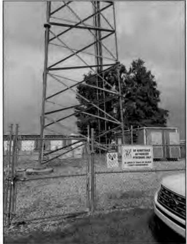
Figure 3 Lower Half of Lattice Tower
