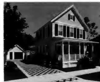
Plan NEH 1.0: 1771 SF Unit 4 bedroom / 3.5 Bath Building Footprint: 26' X 52' Estimated construction cost*: $200,000 - $230,000
