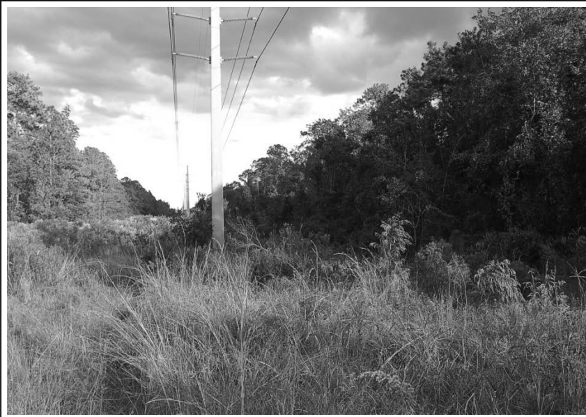
Existing, deforested utility crossing along p McCulloch Rd corridor.
