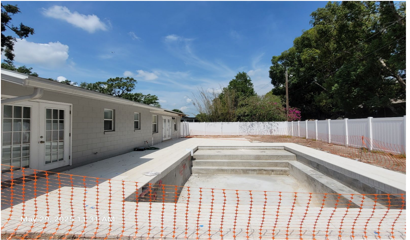
Rear yard, facing west towards proposed patio location
