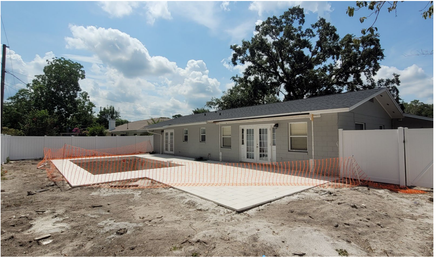
Rear yard, facing southeast towards proposed patio location
