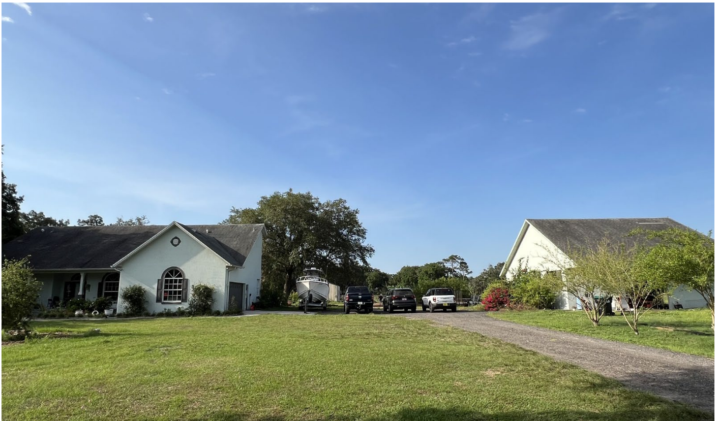
Front yard, facing south towards the house and proposed ADU on right
