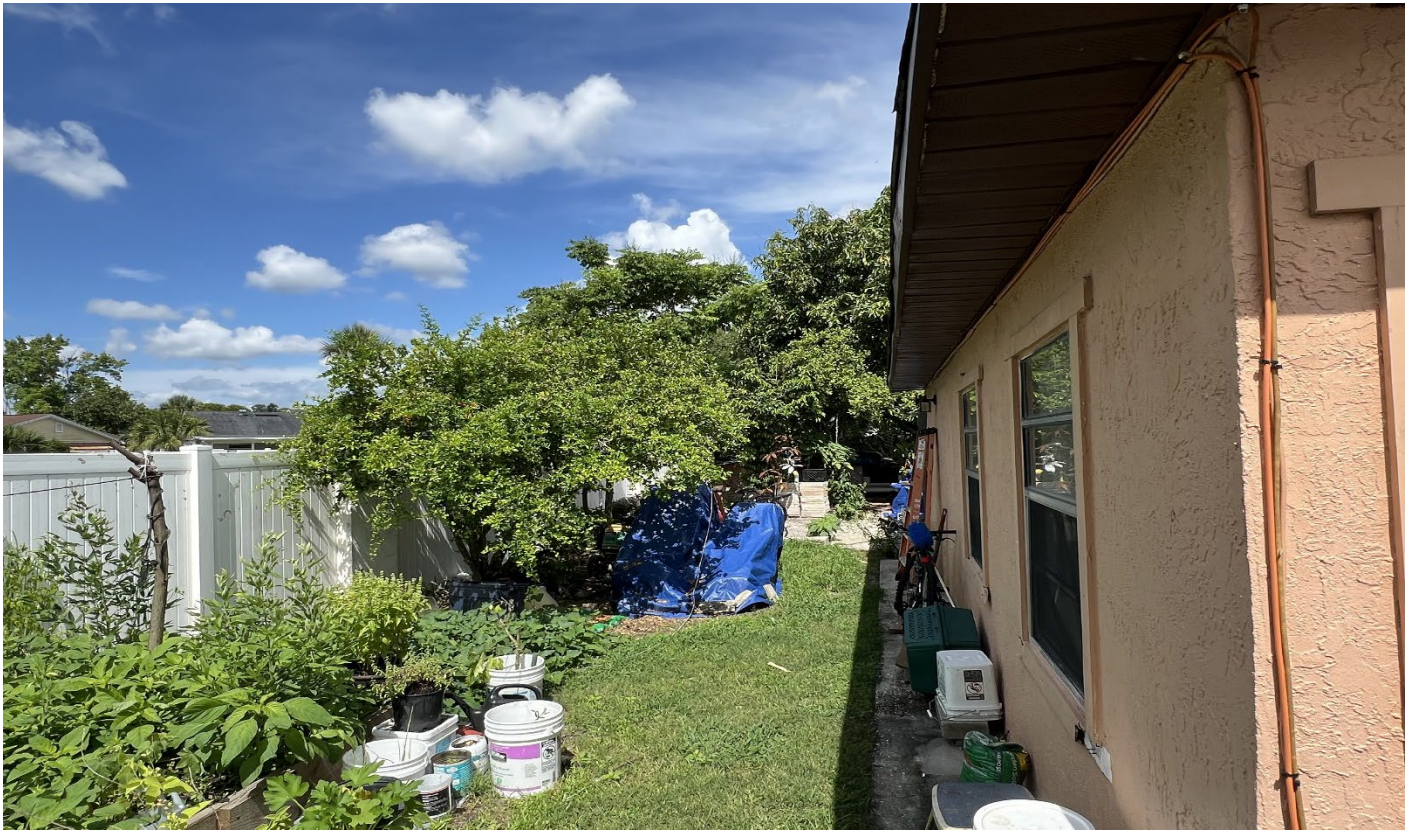
Rear yard, facing west towards the existing unpermitted addition and location of proposed addition
