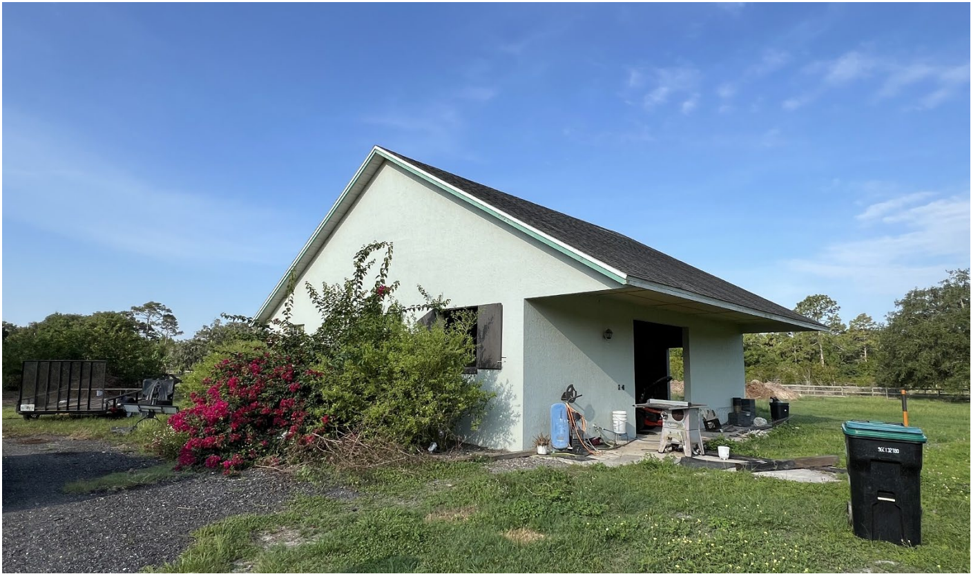
Front yard, facing southwest towards the proposed ADU
