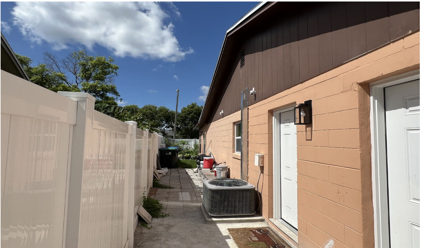
Side yard, facing south towards the existing home
