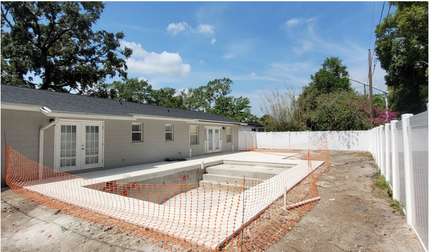
Rear yard, facing southwest towards proposed patio location
