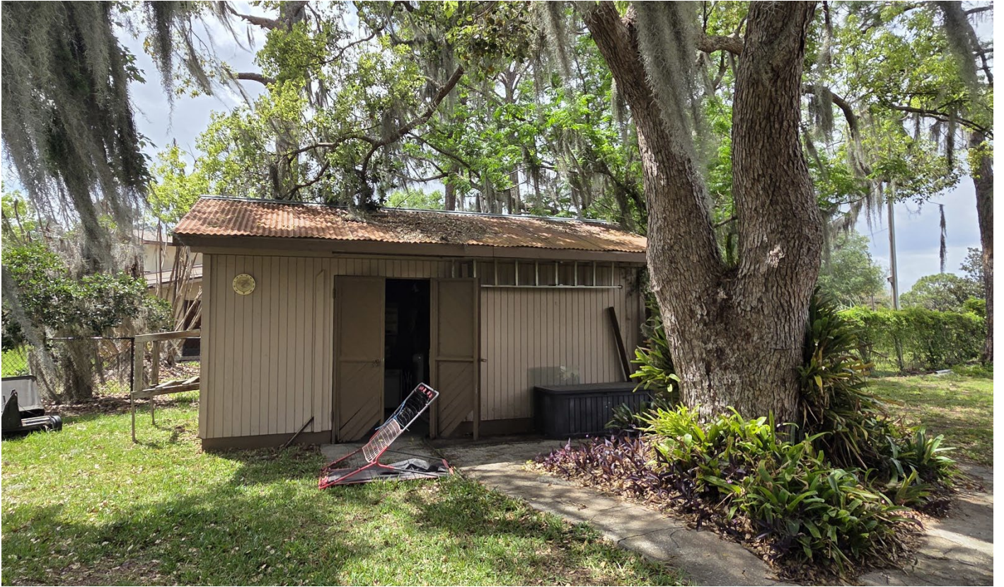
Rear yard, facing west towards the existing shed
