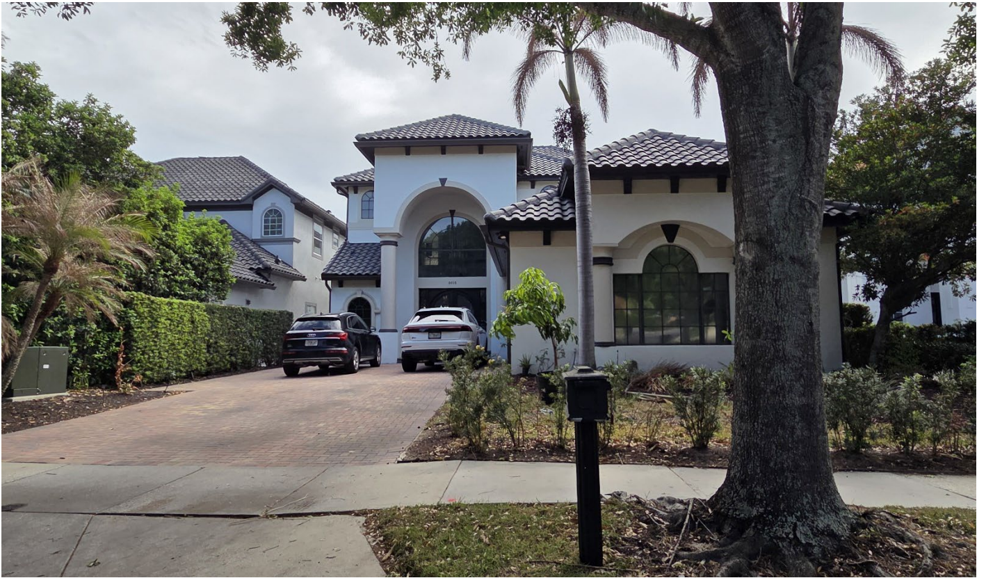
Facing south towards front of subject property
