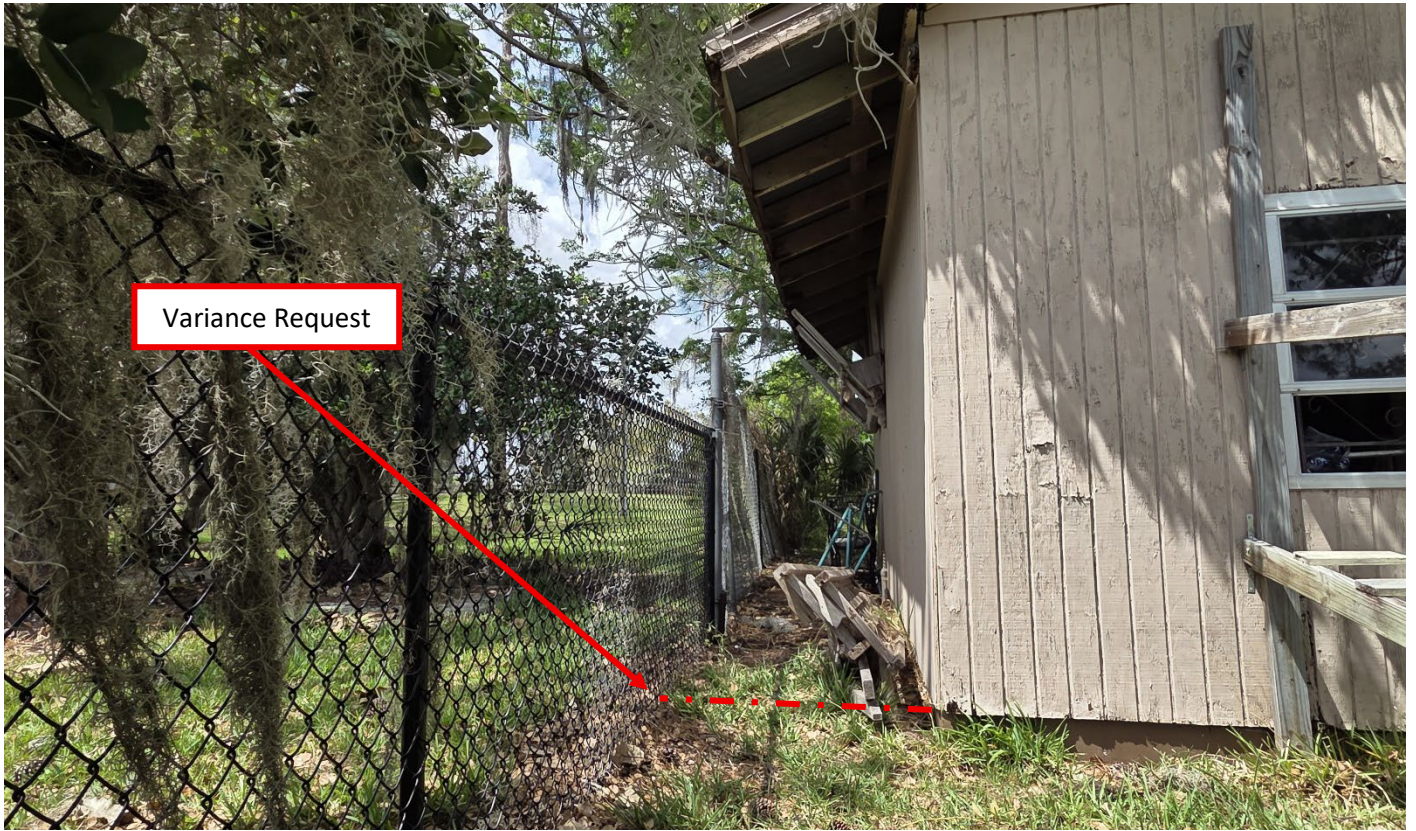
Side yard, facing northwest towards the existing shed
