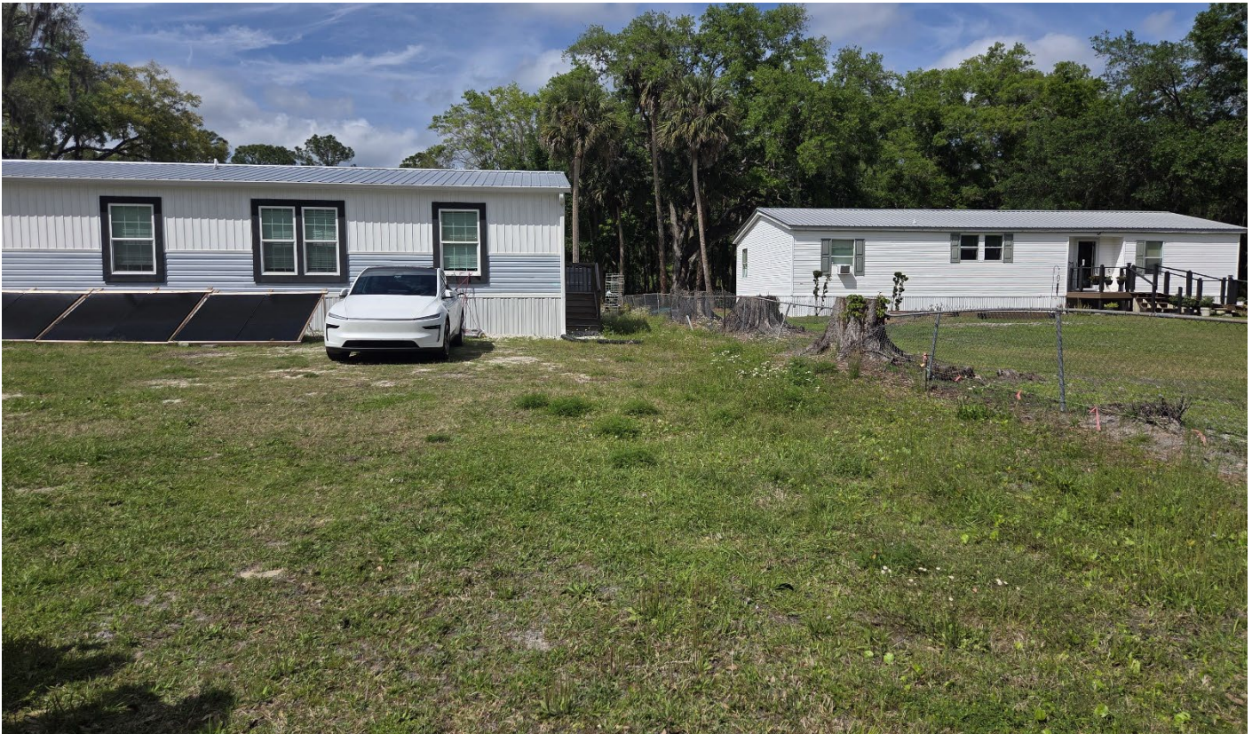
Facing north towards the proposed location of the garage and unpermitted solar panels
