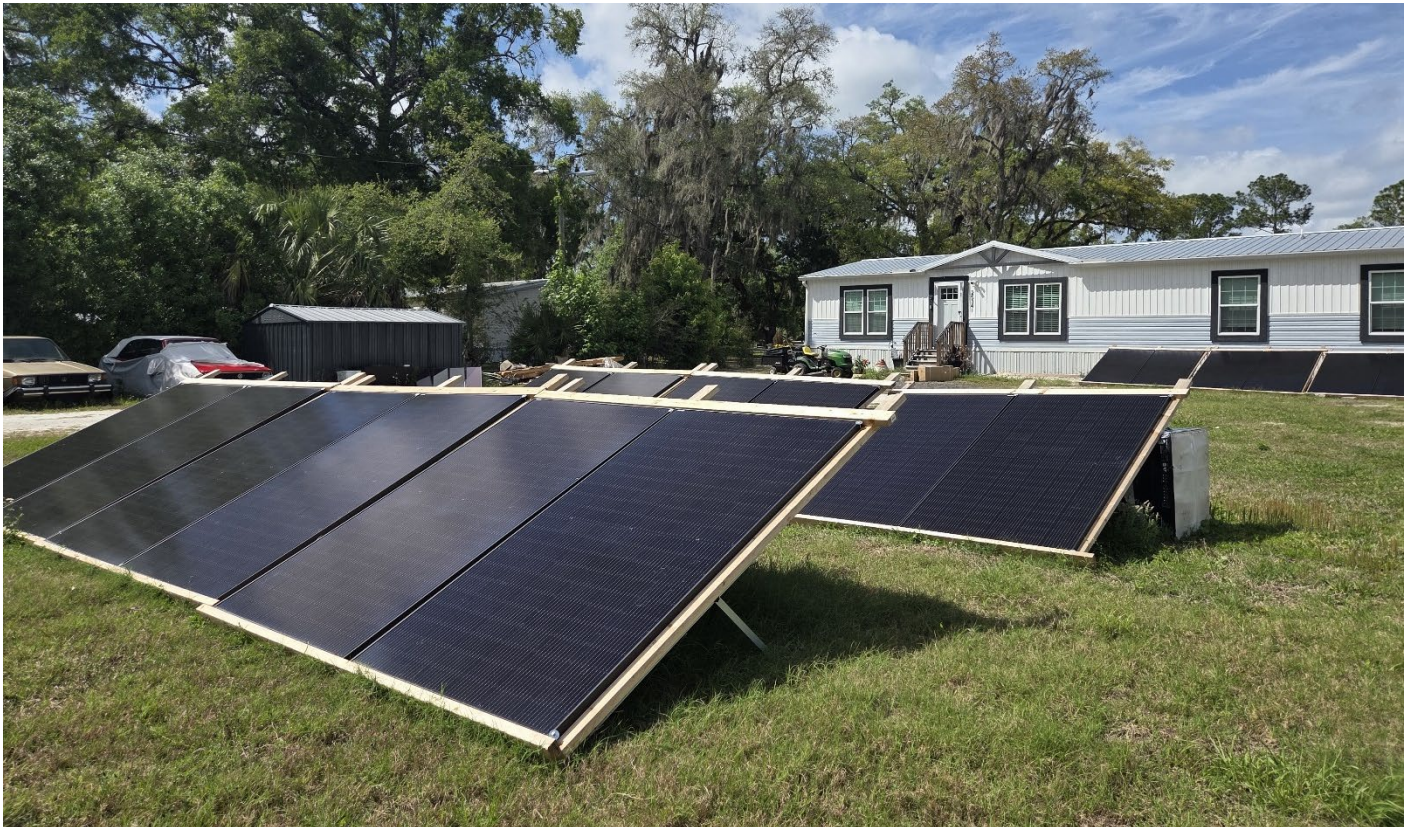
Facing northwest towards unpermitted solar panels and unpermitted shed
