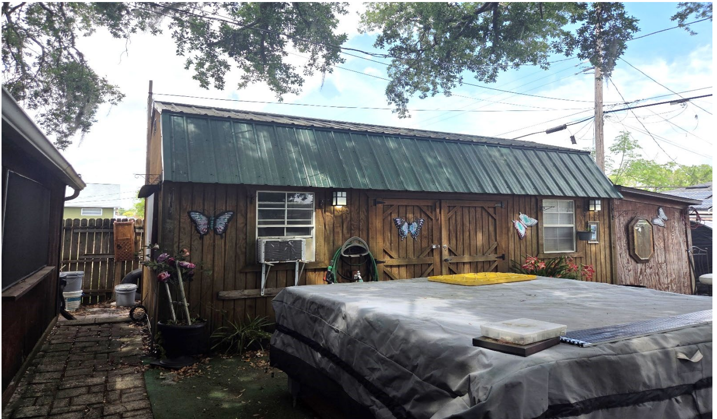
On the subject property, facing north towards the existing shed
