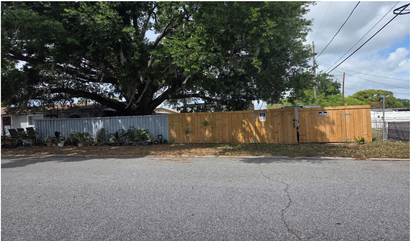
On Seaman St., facing north toward the side street yard and fencing in the right-of-way
