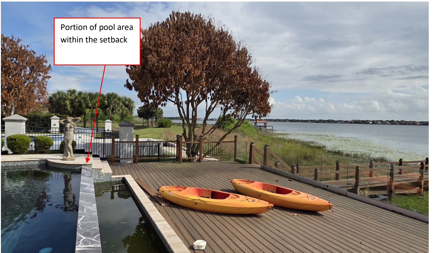
Rear yard, facing southeast towards pool/spa and deck (Variance #2) and wood deck (Variance #1)
