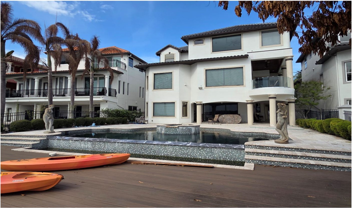
Rear yard, facing north towards pool area
