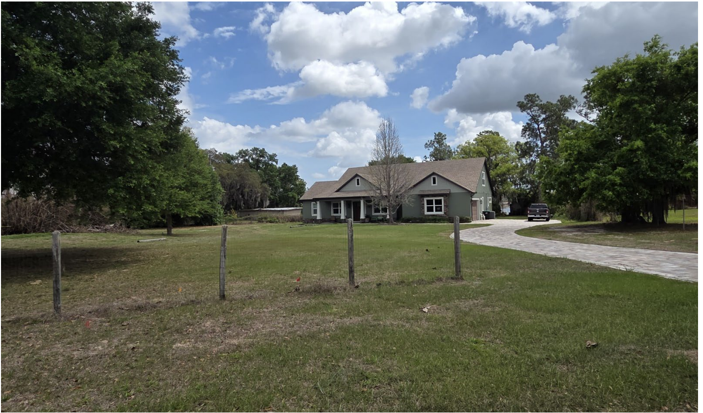
Front yard, facing southeast towards front of subject property
