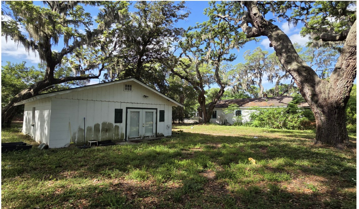
Facing southwest towards the existing structures to be demolished
