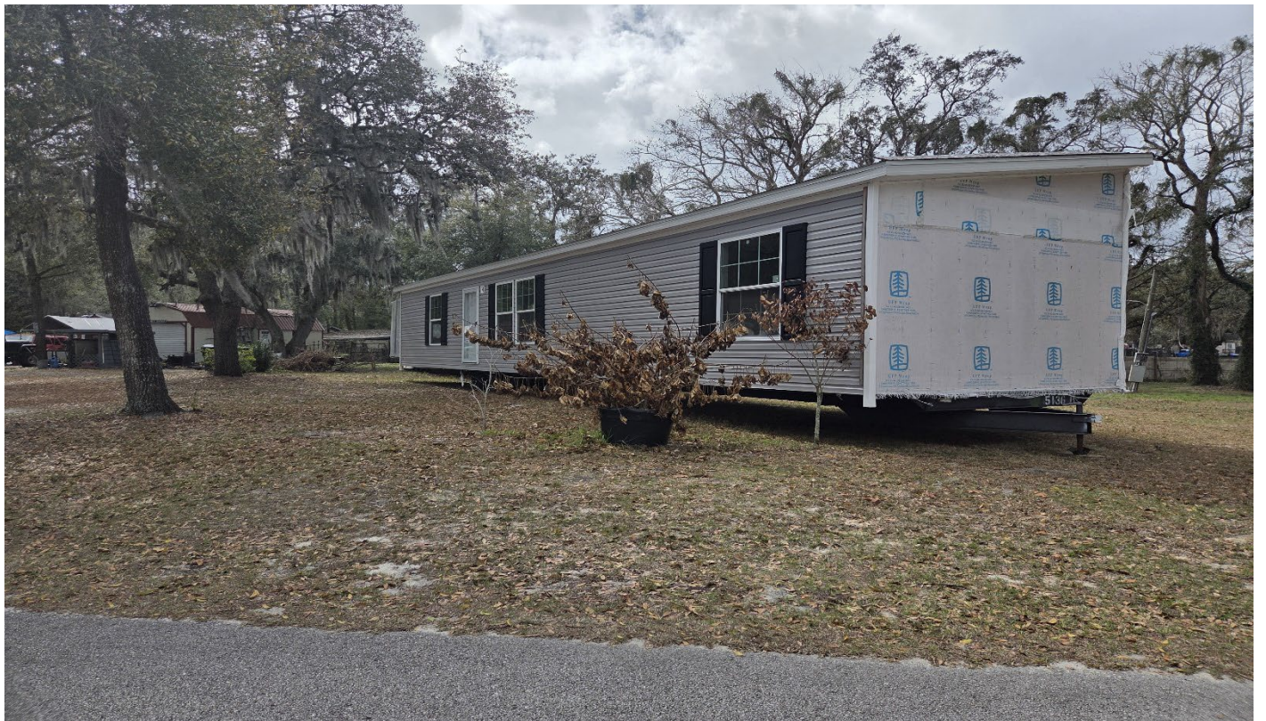
On Pine St., facing south towards front of subject property
