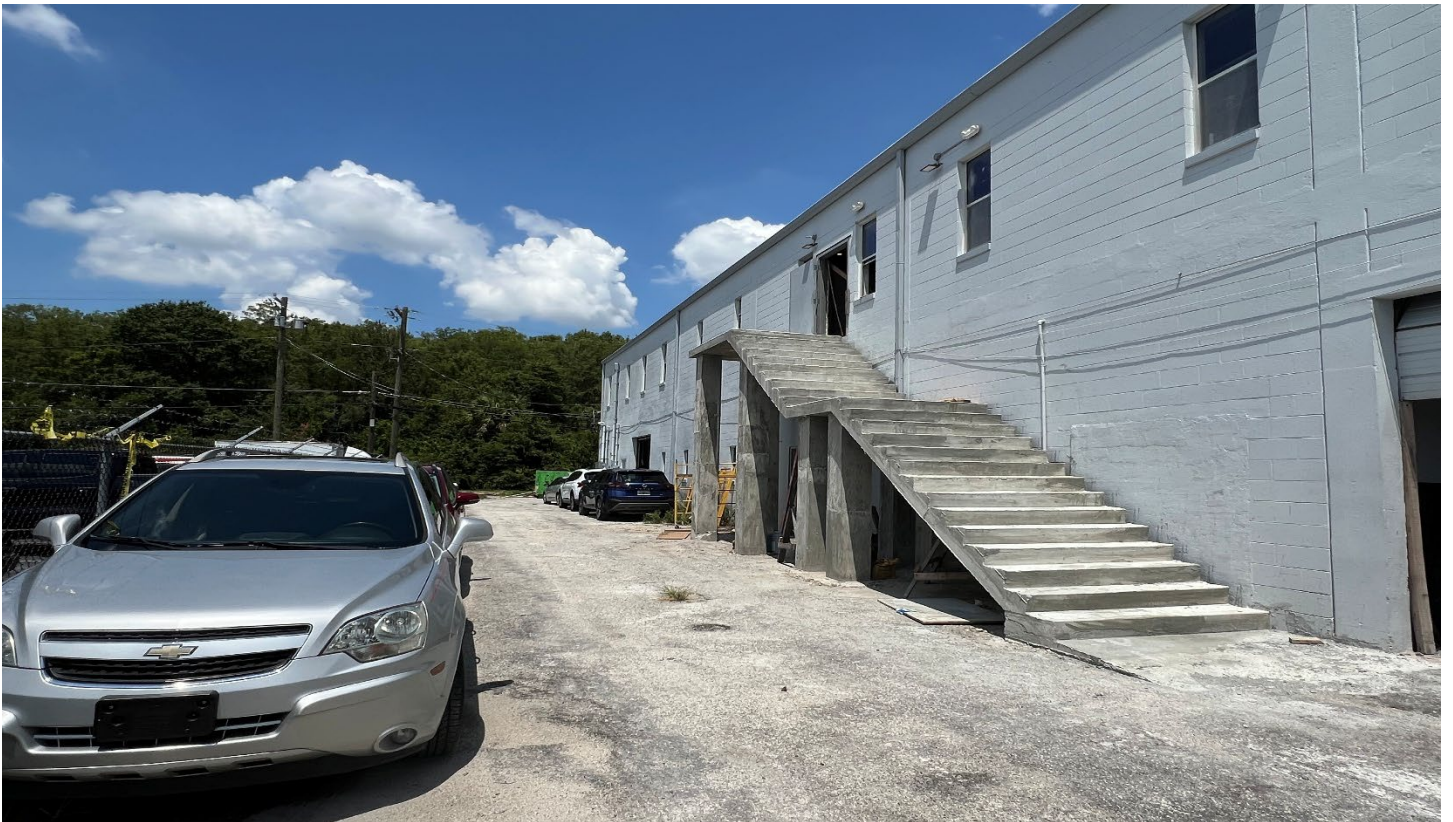
From south property line, facing the exterior staircase
