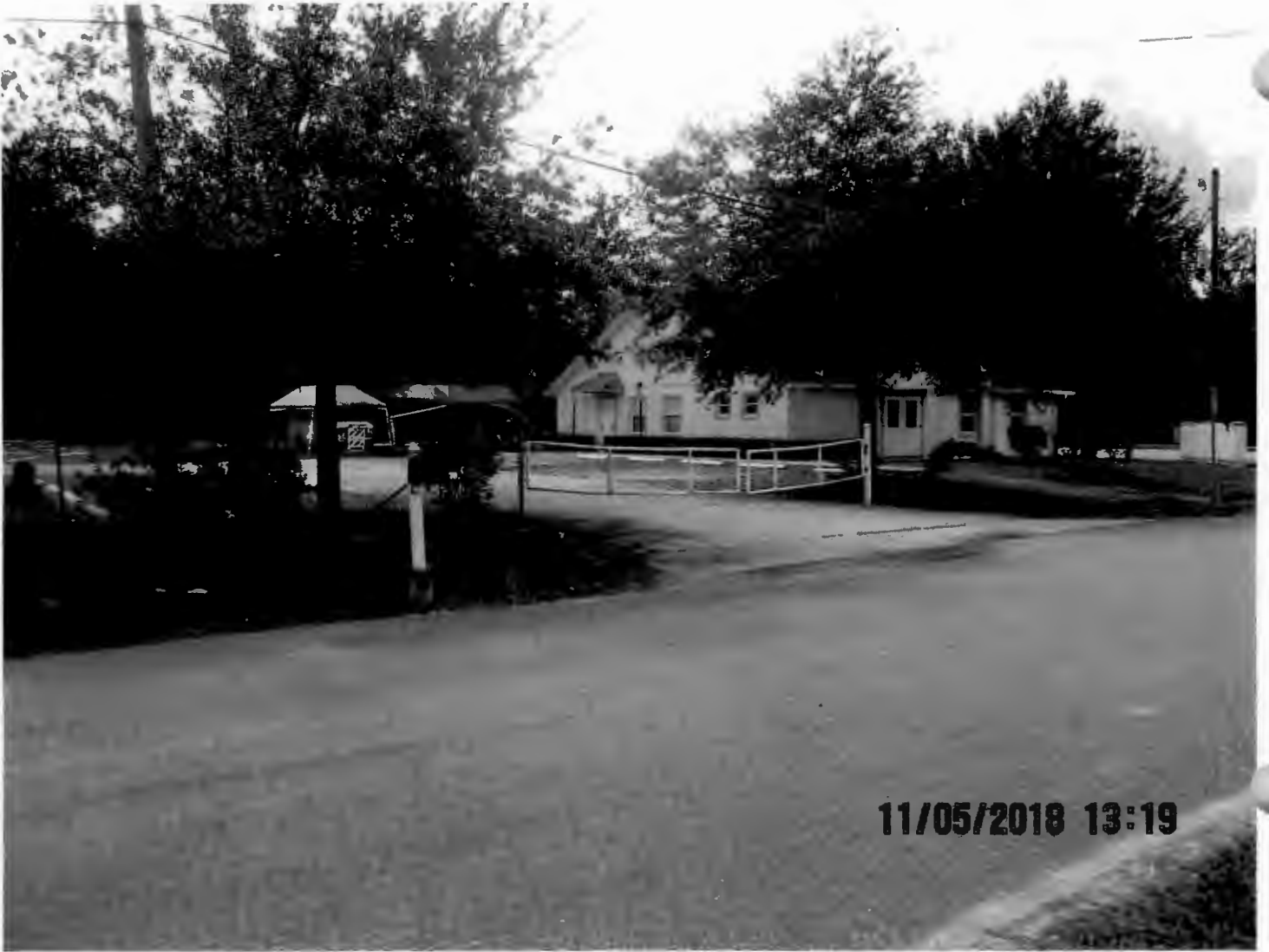
VIEW FROM ALCOCK RD.
