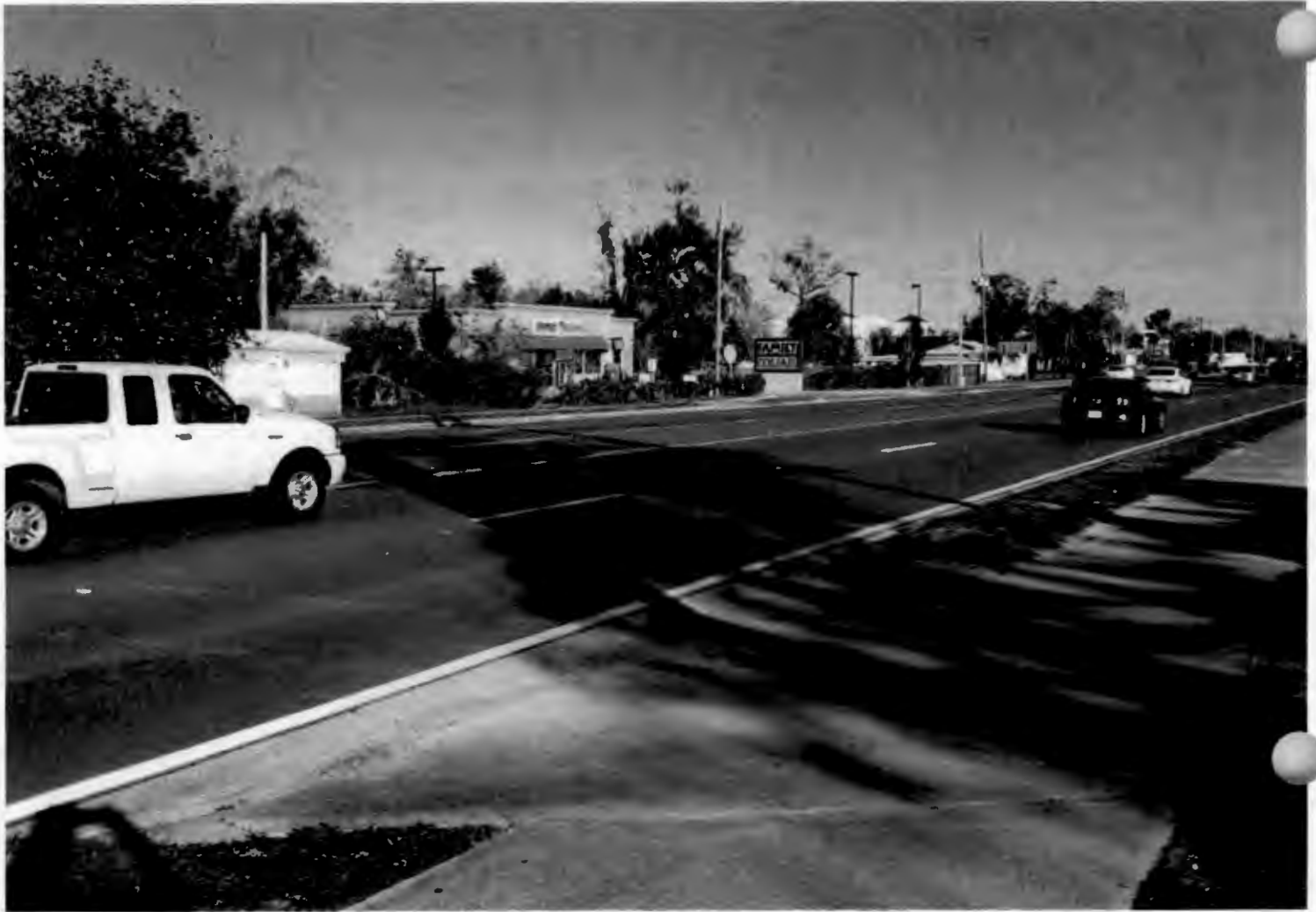
Looking North along Dean Rd. from subject property
