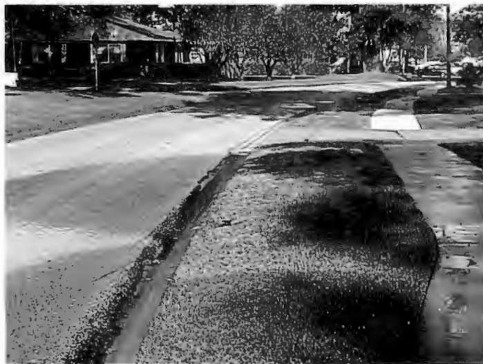
Figure 12. Poor design; sprinkler does not match area.
