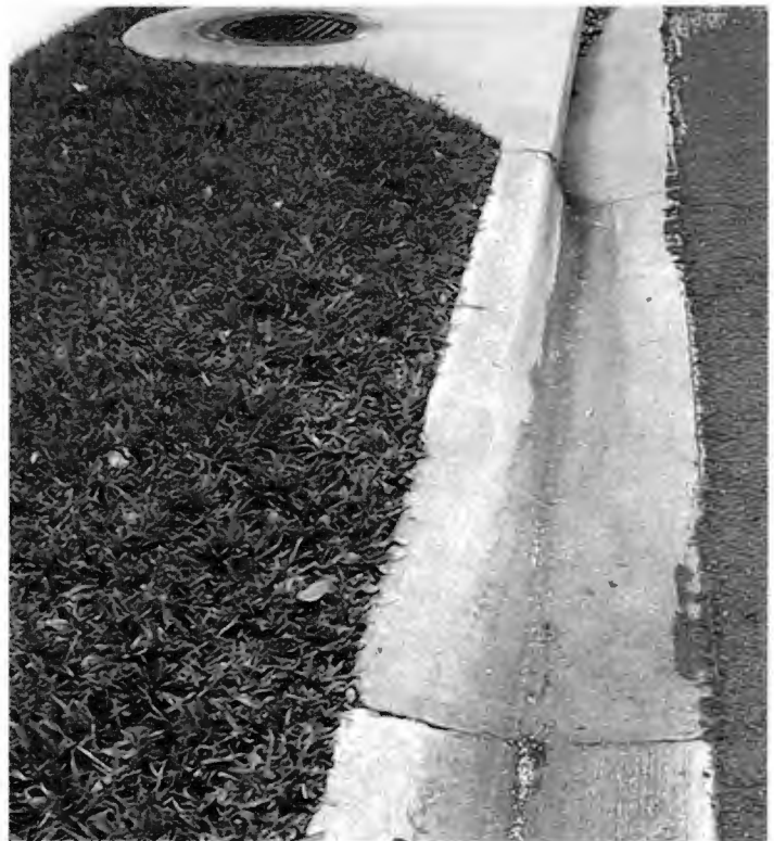
Figure 19. Slow or quick release, this fertilizer is going to a water body. Keep fertilizer away from impervious surfaces and water bodies.
