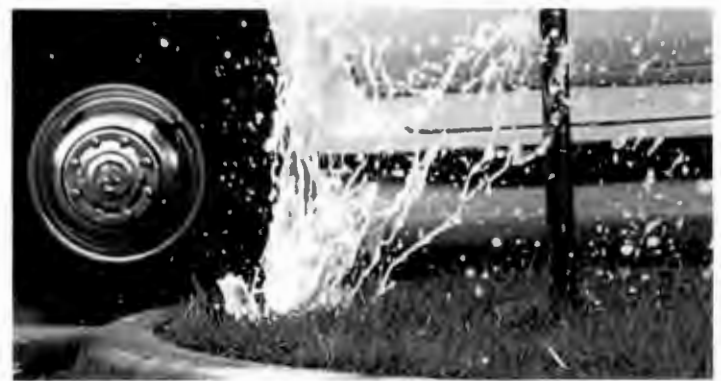
Figure 16. Water gushing from broken head.
