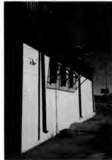
HVAC elevated above first-floor
