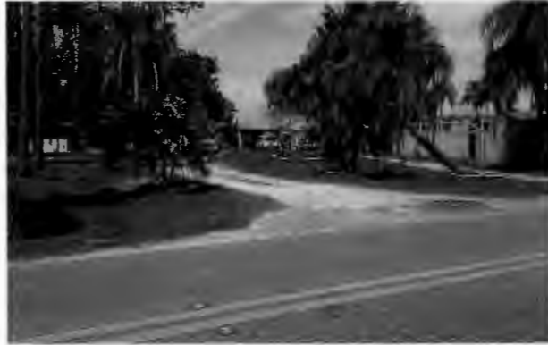
Drainage swale in front yard
