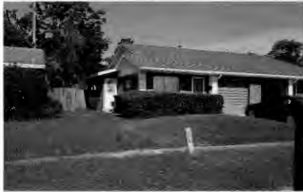
Drainage swale between lots
