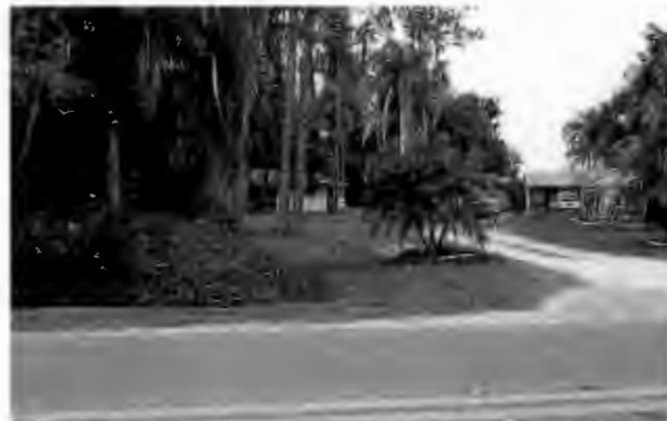
Drainage swale in front yard along road
