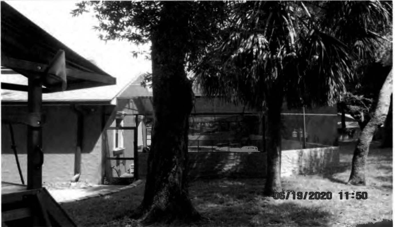
Proposed location of covered porch addition looking north
