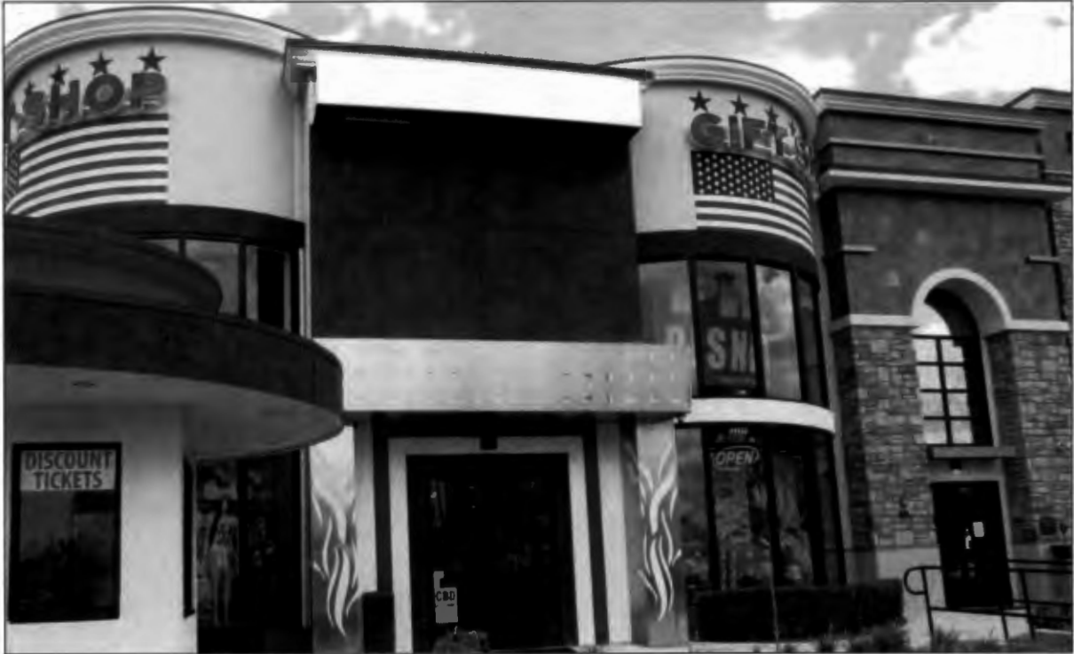
View of west building frontage along S. Apopka Vineland Road facing east
