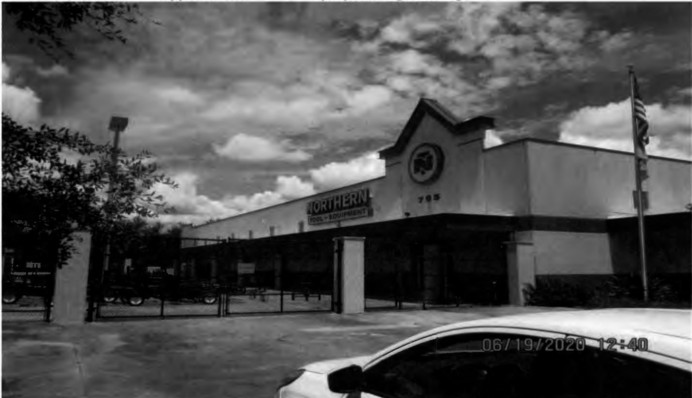
Existing sign looking northwest
