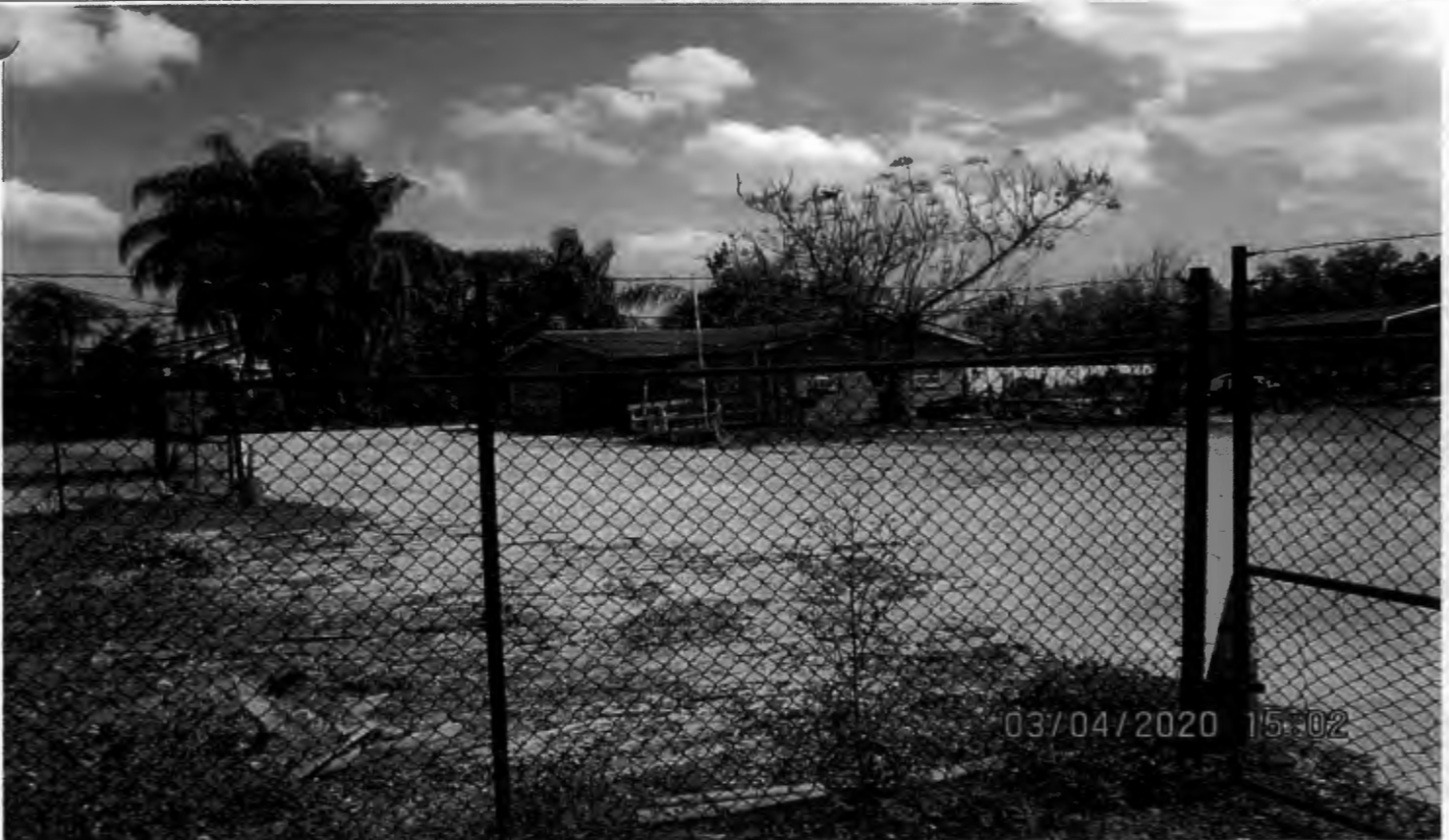
Existing office building for nursery, looking southeast
