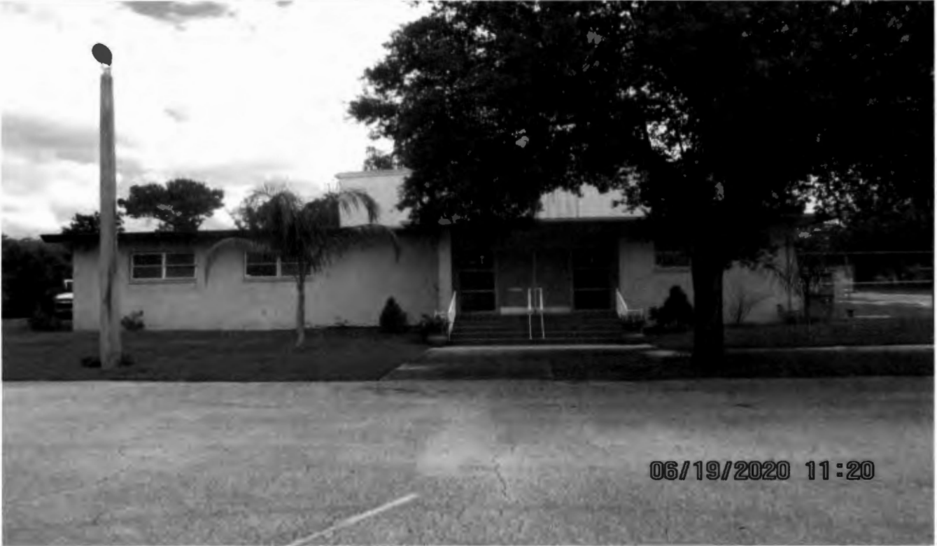
Side entrance to existing sanctuary building facing north from the existing parking lot
