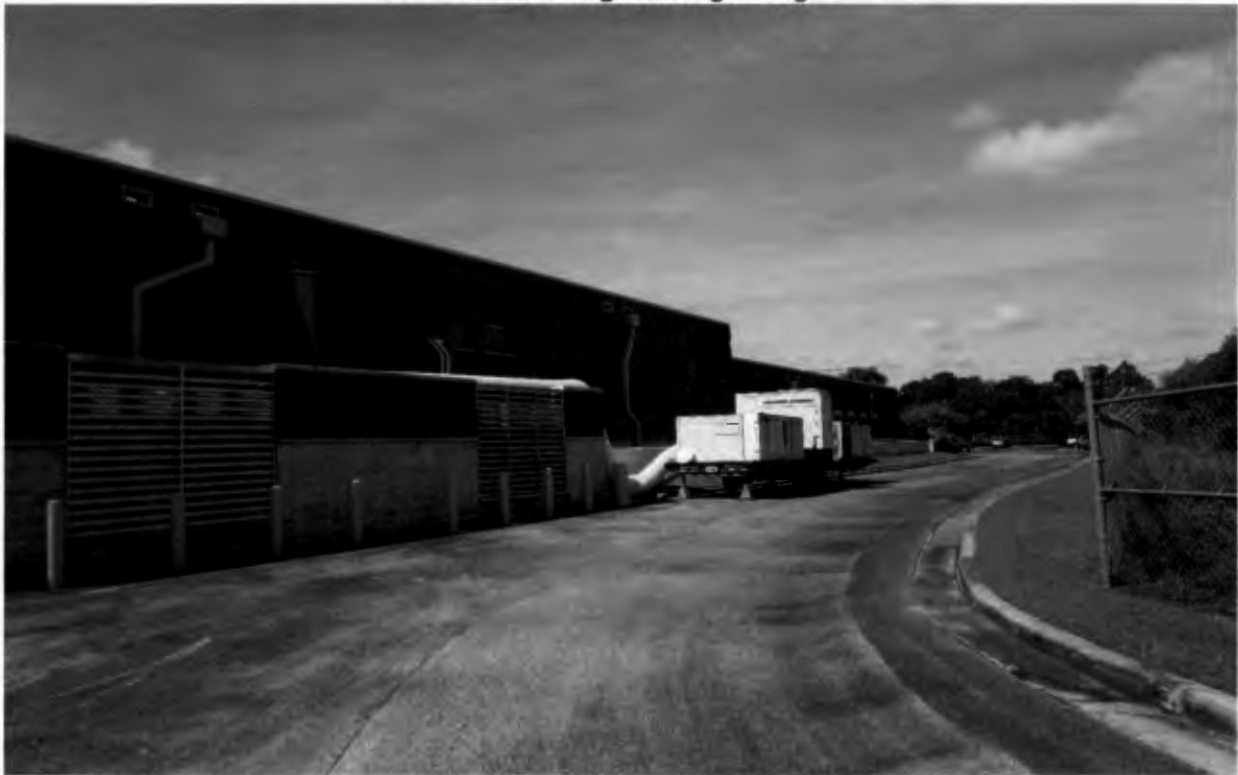
Rear of existing building facing northwest – the new building addition will be in the background
