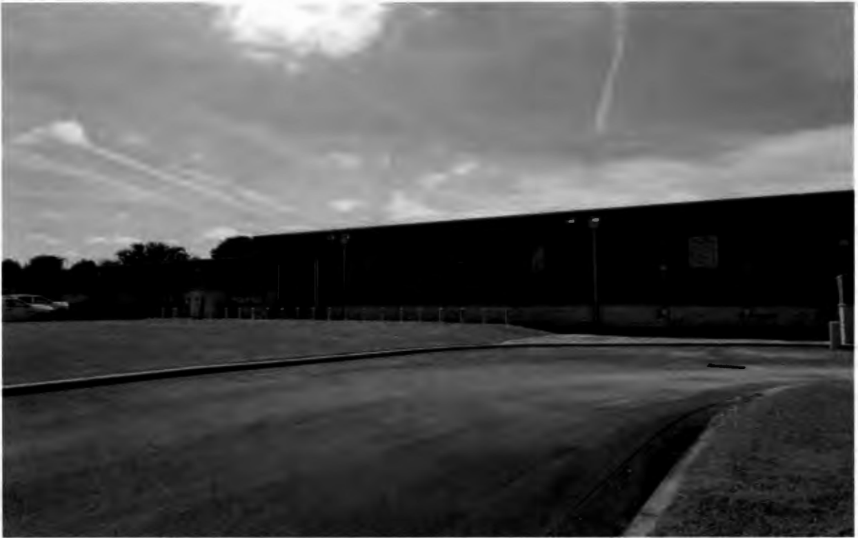
Approximate location of proposed addition facing southeast
