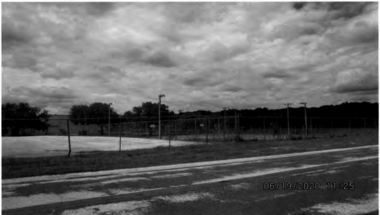
Facing west to the Pine Hills YMCA recreation facility – existing parking lot in foreground
