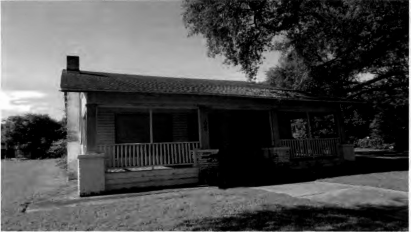
Residence proposed for conversion to offices facing southwest
