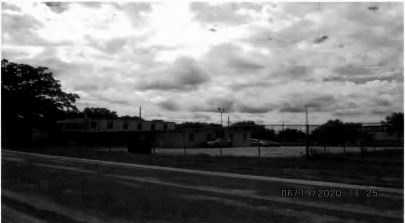
Facing southeast from Arundel Dr. to the location of proposed fellowship hall
