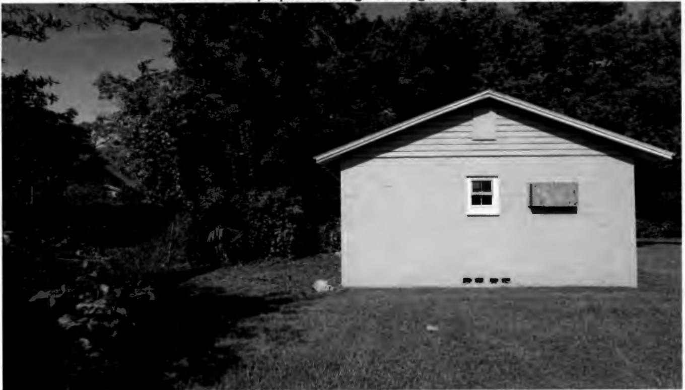
East side of proposed storage building facing west
