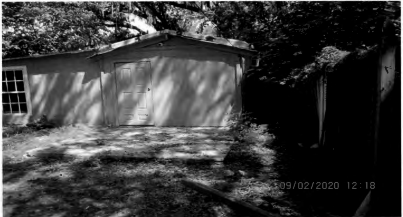
Accessory structure 6.4 ft. side (east) setback facing northeast
