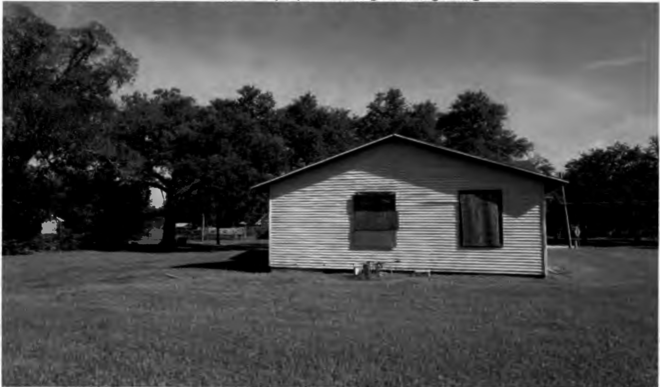
East side of building facing west
