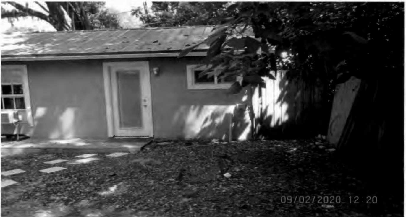
Residence 5.4 ft. side (east) setback facing northeast
