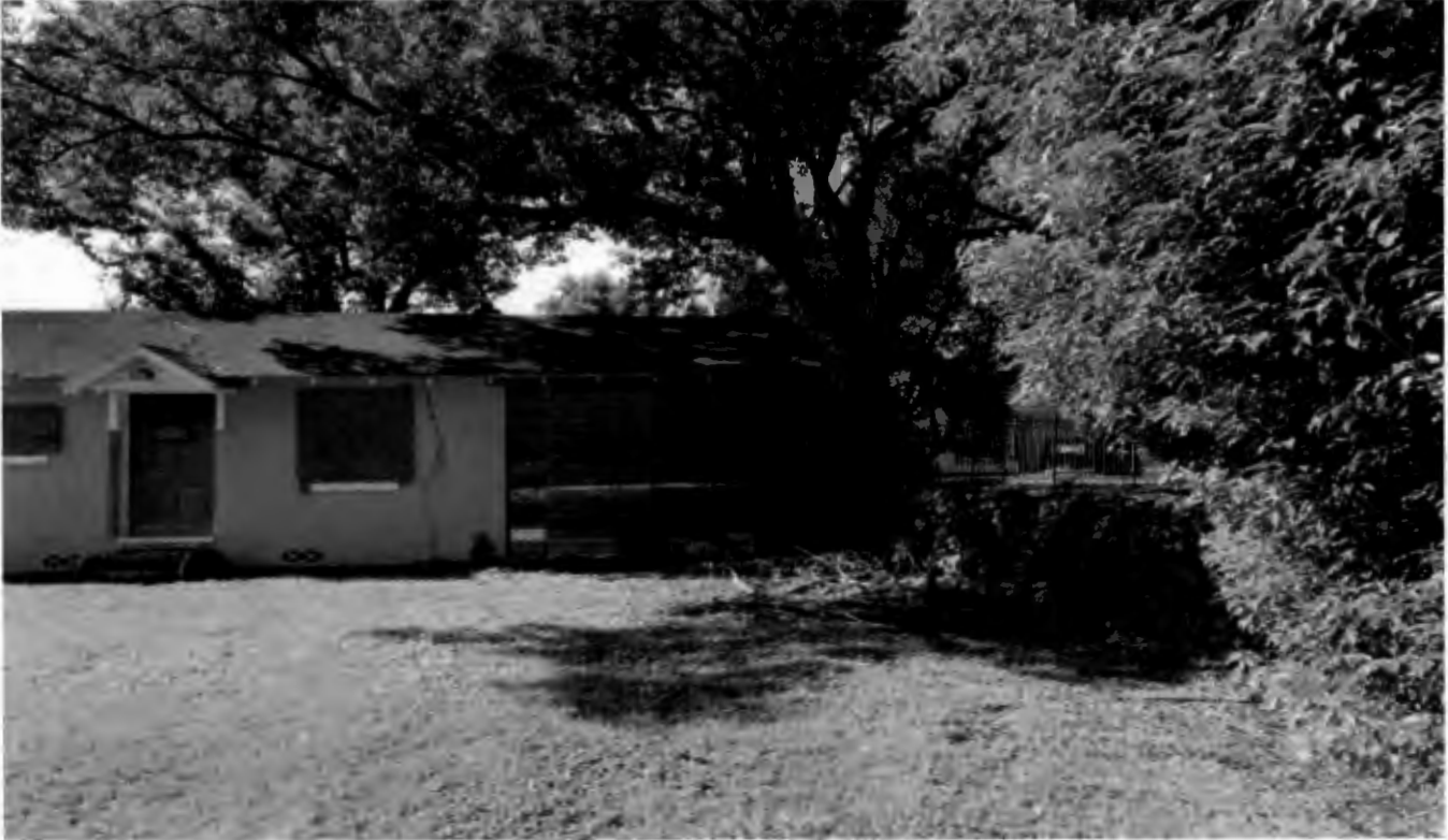
West side of proposed storage building facing south
