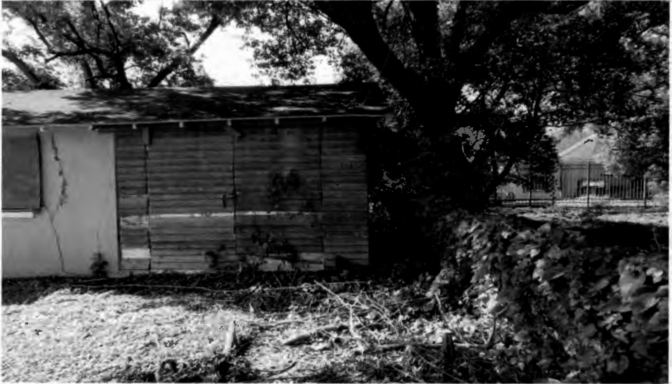
West side setback of proposed storage building facing south
