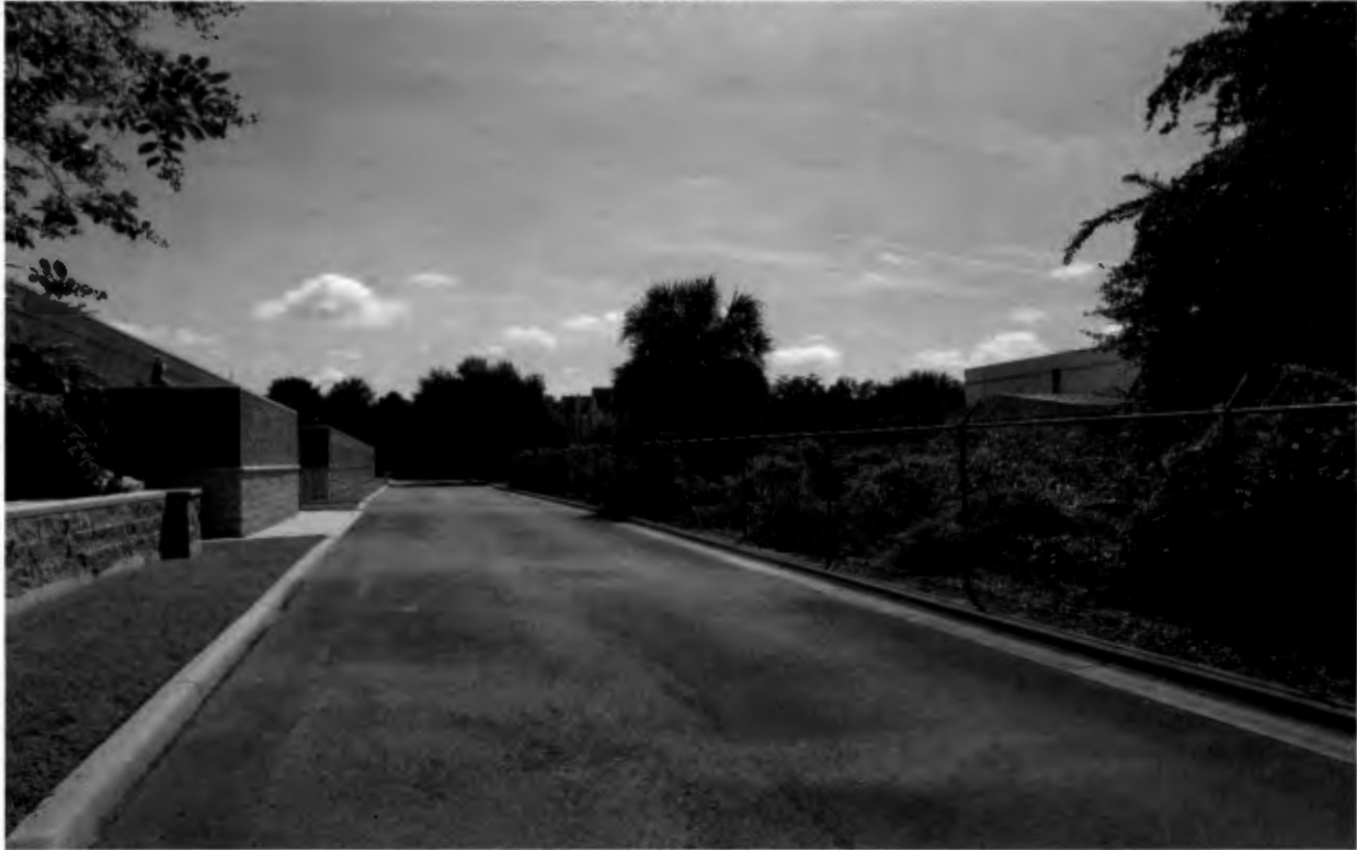
South side existing building facing east
