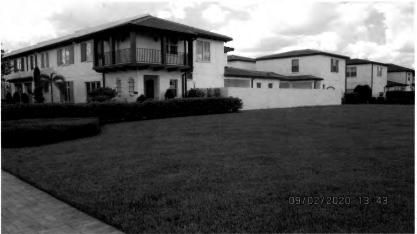
View of Front of property facing west
