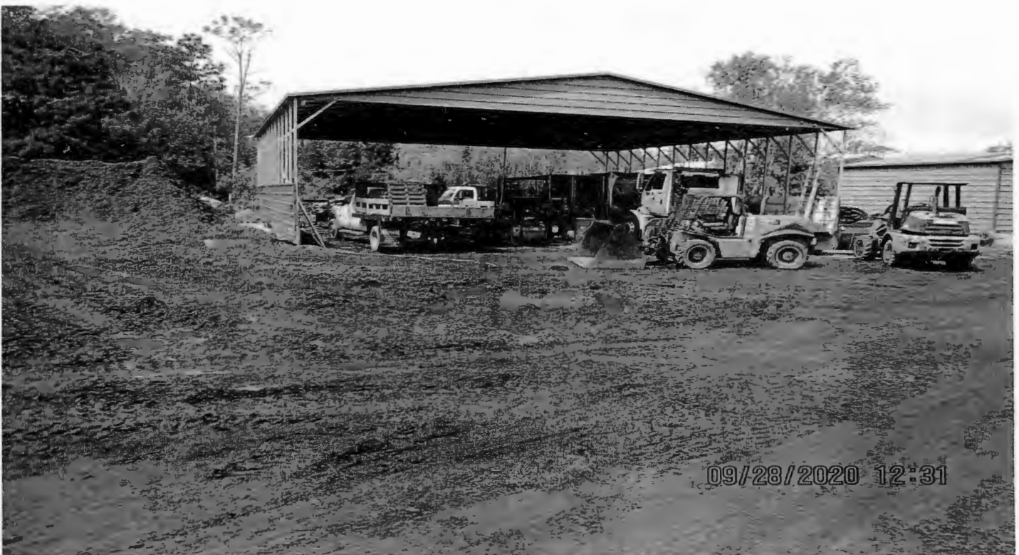
Bldg. D-2,525 sq. ft. pole barn, looking west
