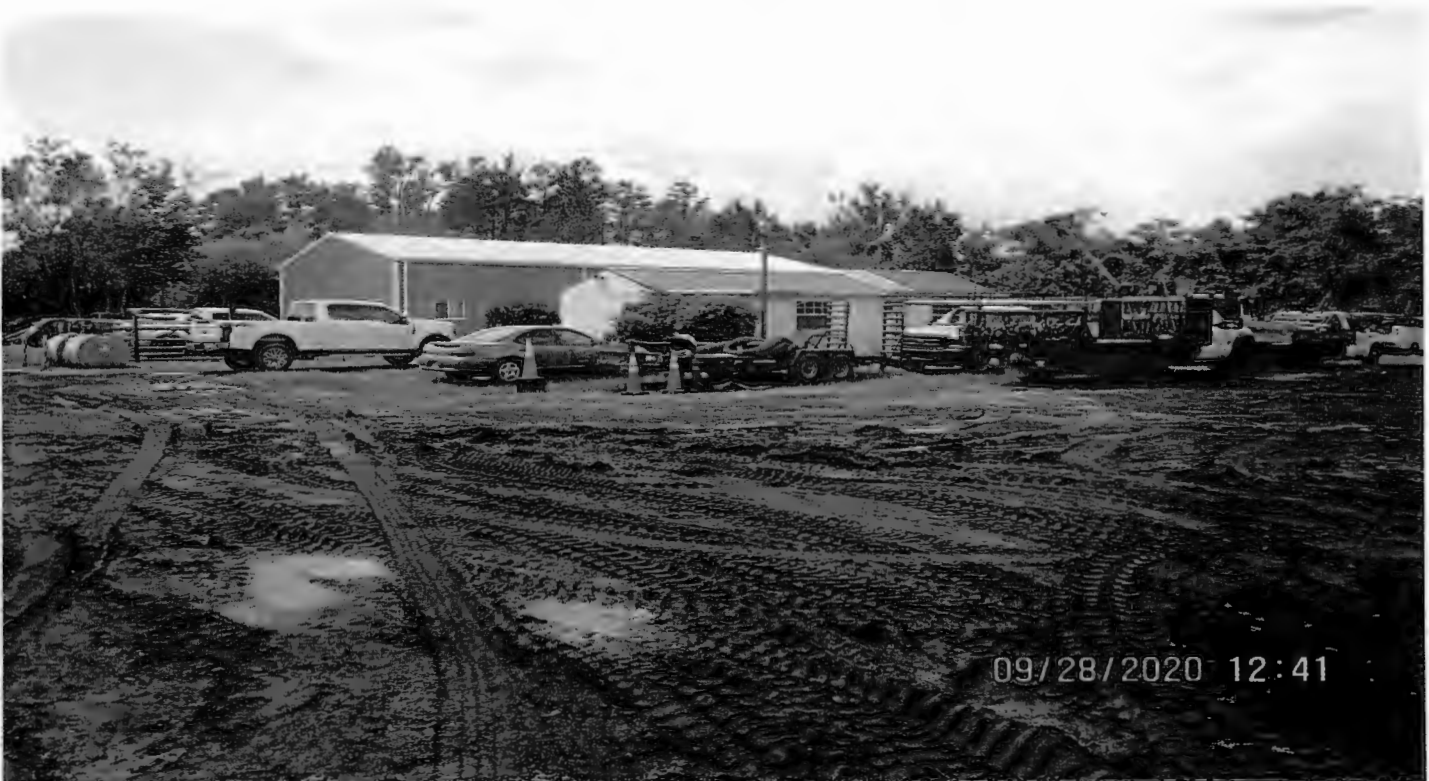
Bldg B-846 sq. ft. storage bldg., and Bldg C-3,000 sq. ft. Office-Warehouse, looking south
