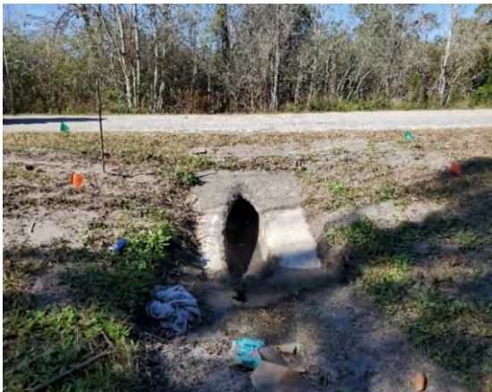
Figure 3-6 Existing Cross Drain, CD #1
