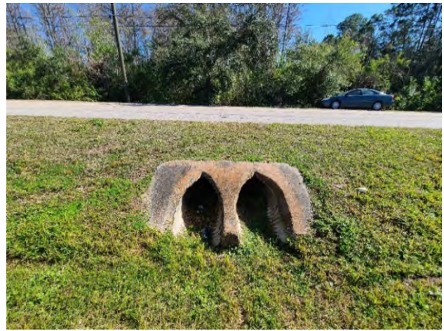
Figure 3-9 Existing Cross Drain (CD #3)
