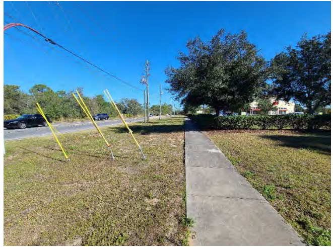
Figure 3-5 Roadside Ditch Facing North
