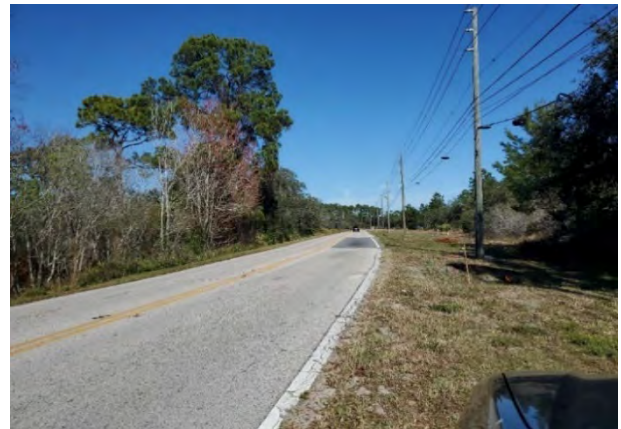
Figure 3-7 Roadside Ditch Facing North
