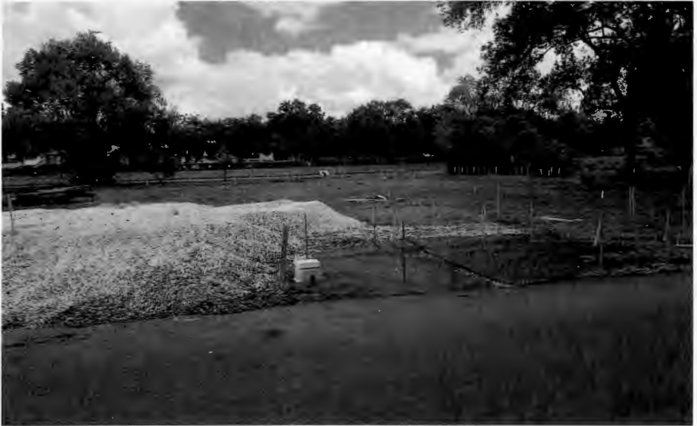
Existing parking lot under construction across Jessamine
