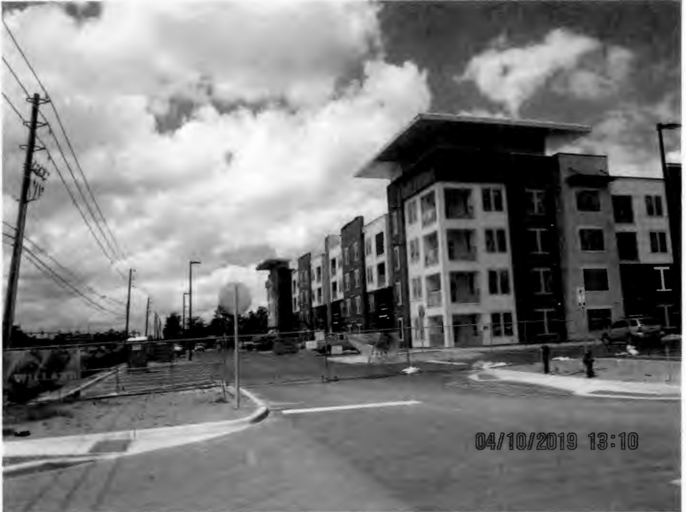
Site looking west
