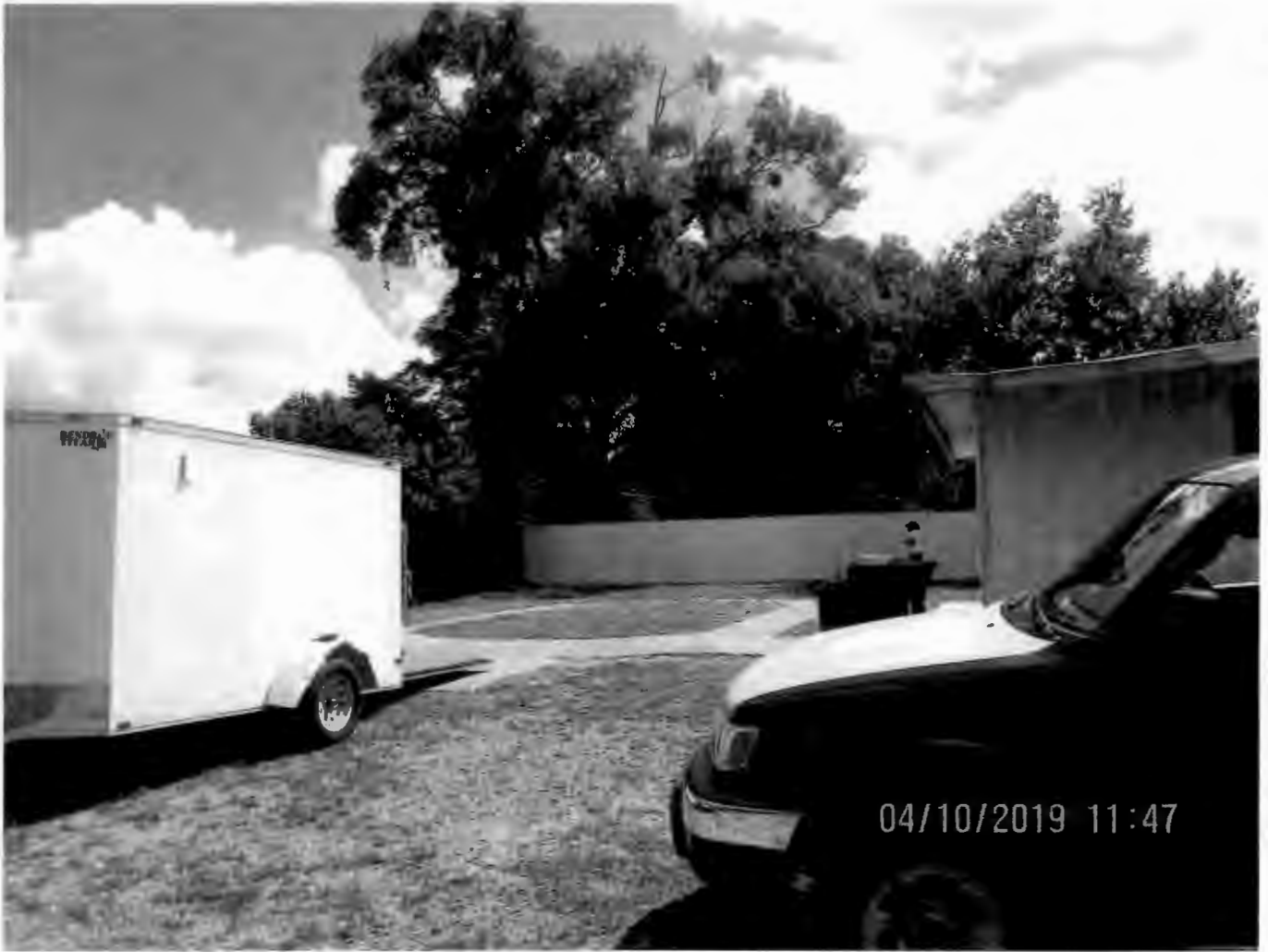
Side of Structure Where Addition Proposed Looking West
