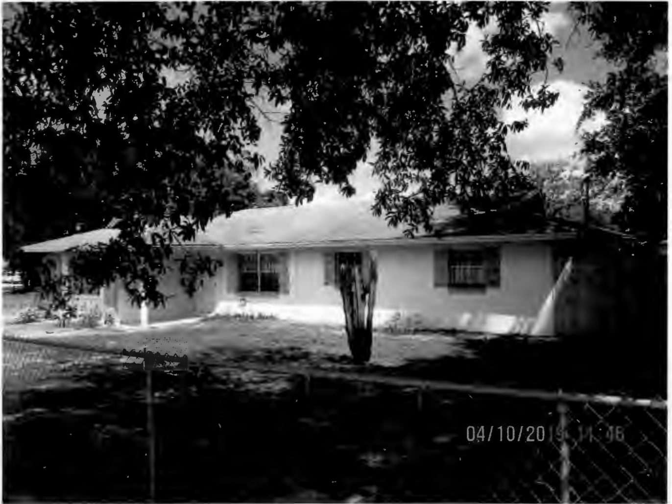
Side of Structure Looking North
