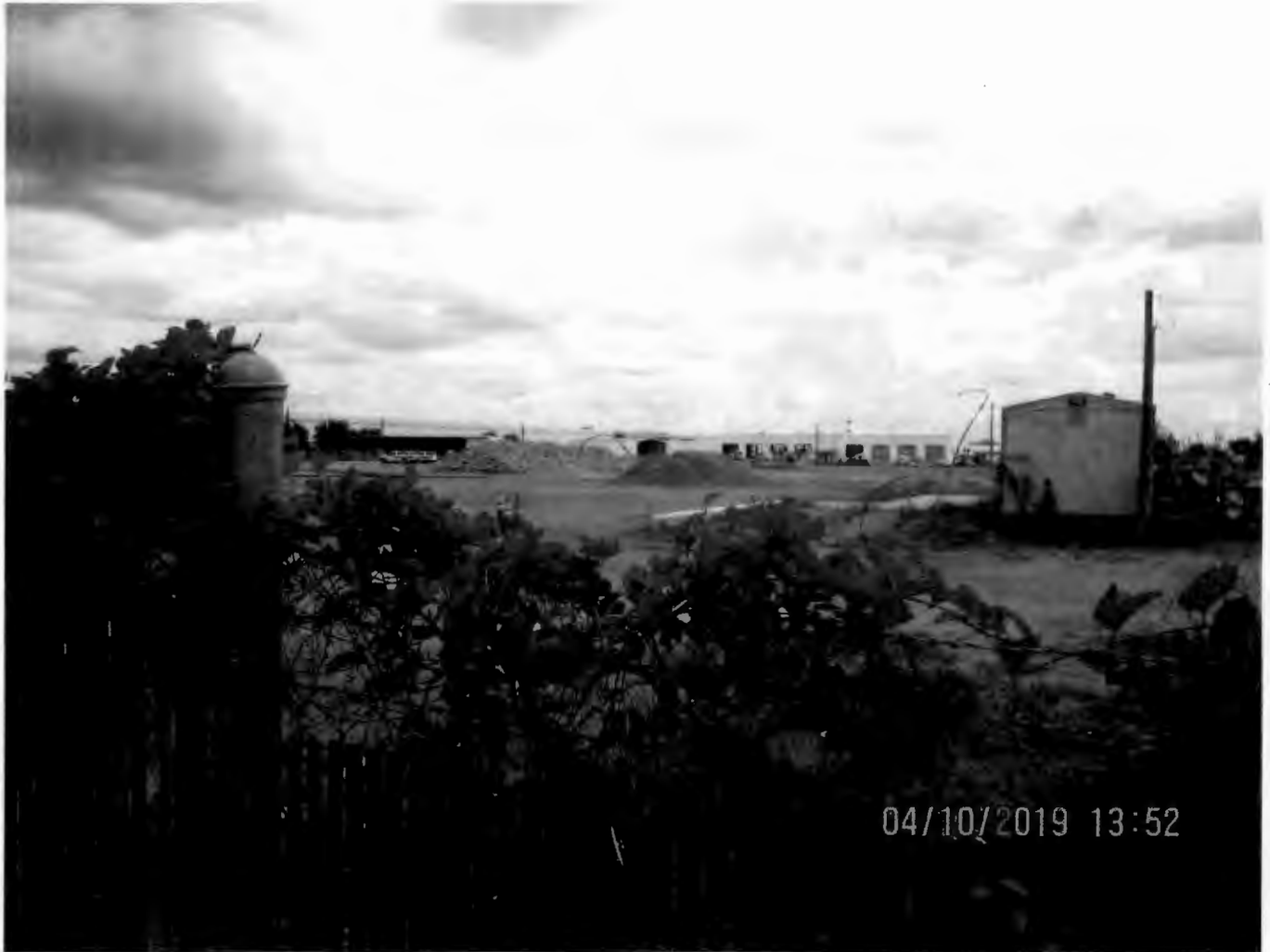
Site Looking East
