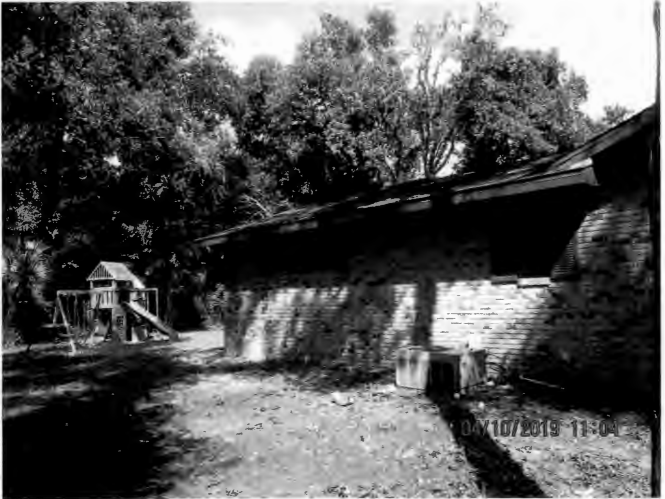
West Side of House proposed Location of Addition
