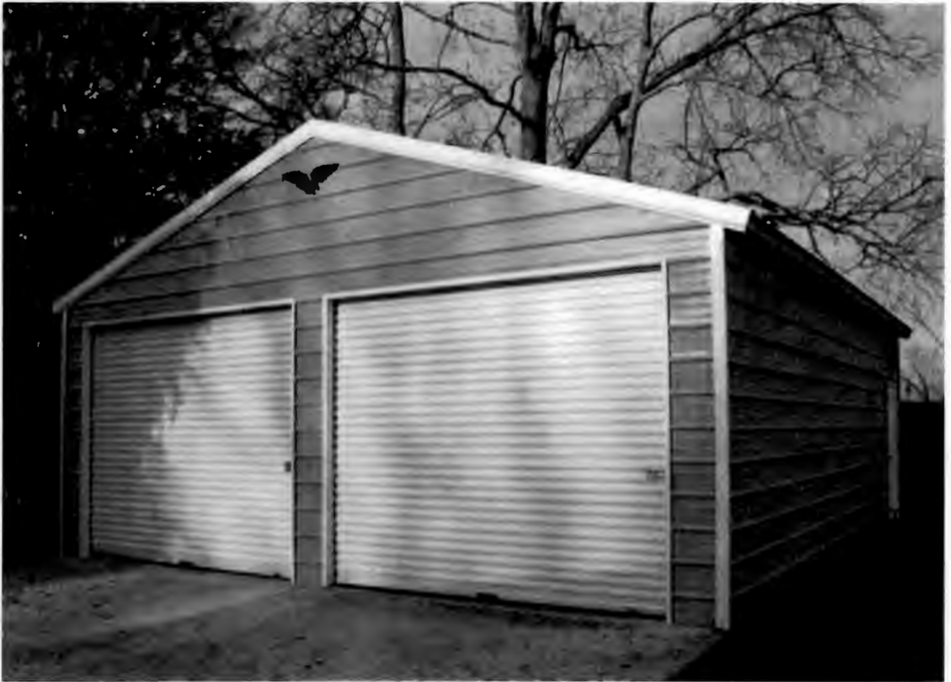
Example of steel building
