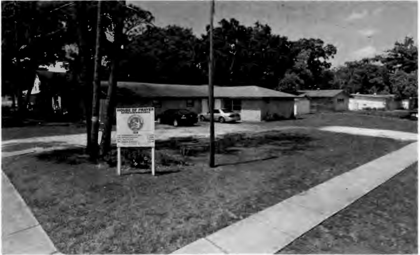
Street view from the intersection
