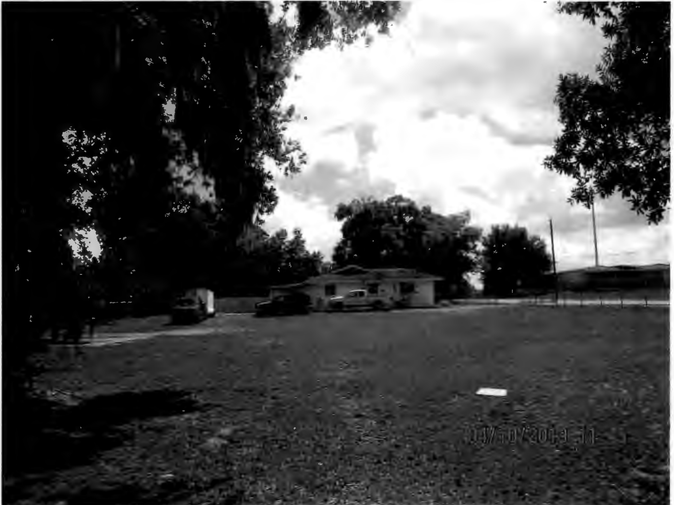
Front of Structure Looking from the west
