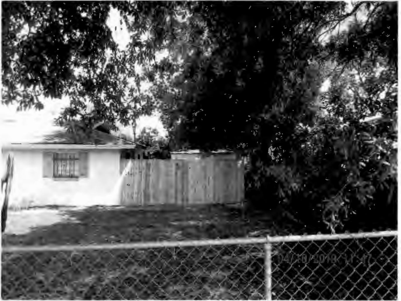
Rear of Structure Looking North
