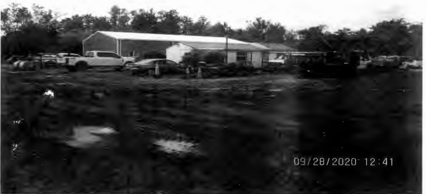
Bldg B-846 sq. ft. storage bldg., and Bldg C-3,000 sq. ft. Office-Warehouse, looking south
