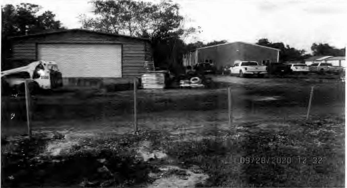
Bldg A-633 sq. ft. shed, and Bldg C-3,000 sq. ft. Office-Warehouse, looking west
