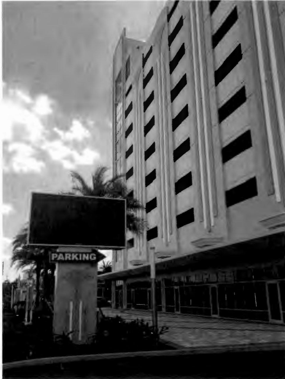
View from the north property line
