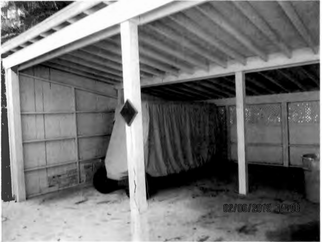
Interior of Existing Carport
