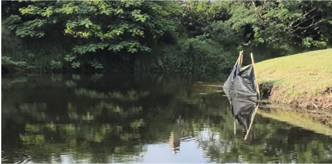
Inadequate soil control during construction
