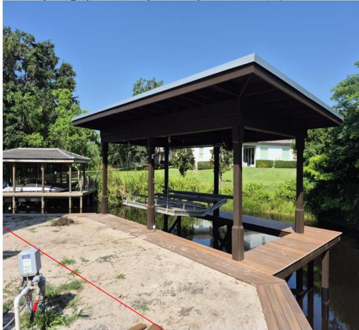
EPD photograph from compliance inspection on May 6, 2025
