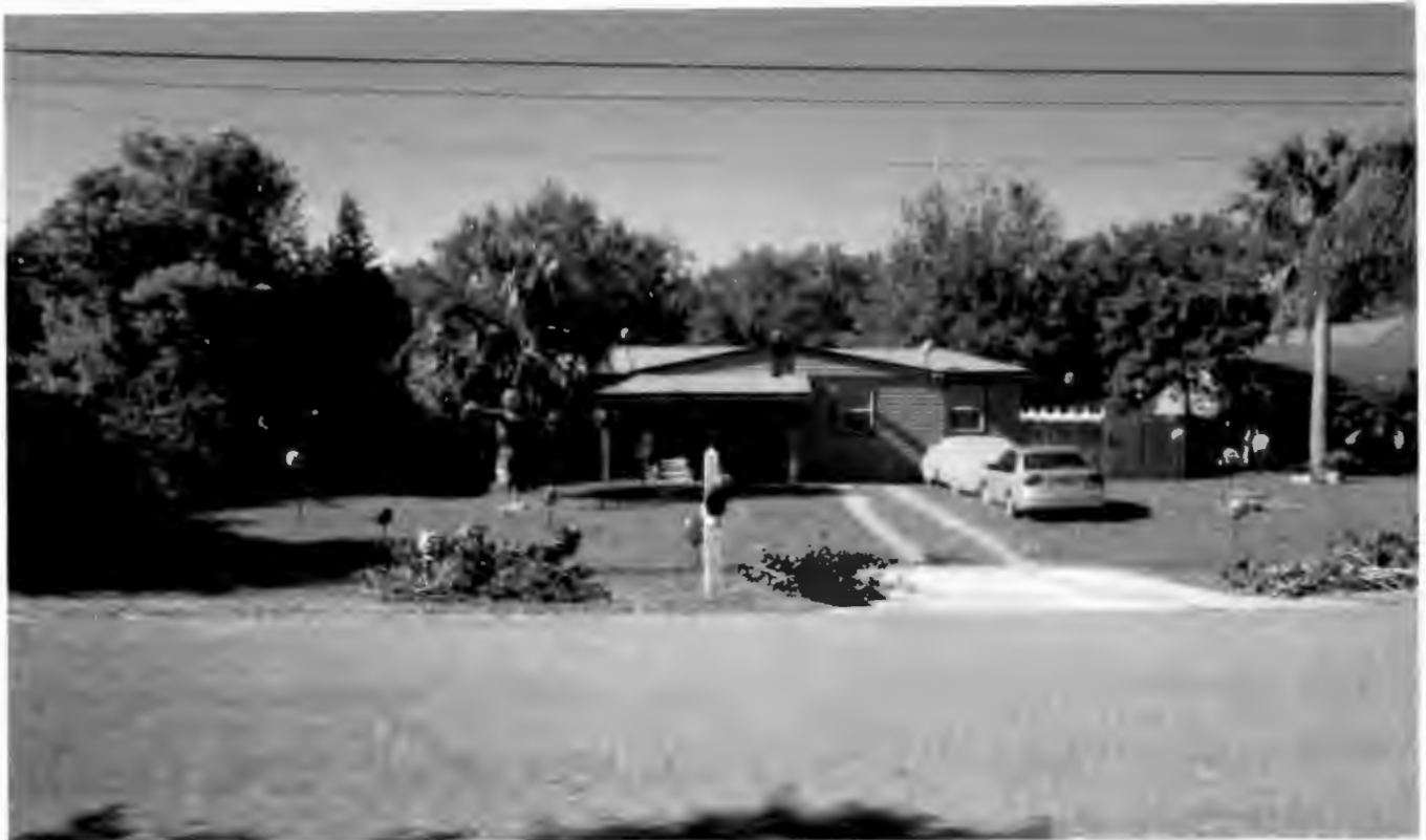
Facing south from Sawyer Shores Ln. towards proposed Additions #1 and #4
