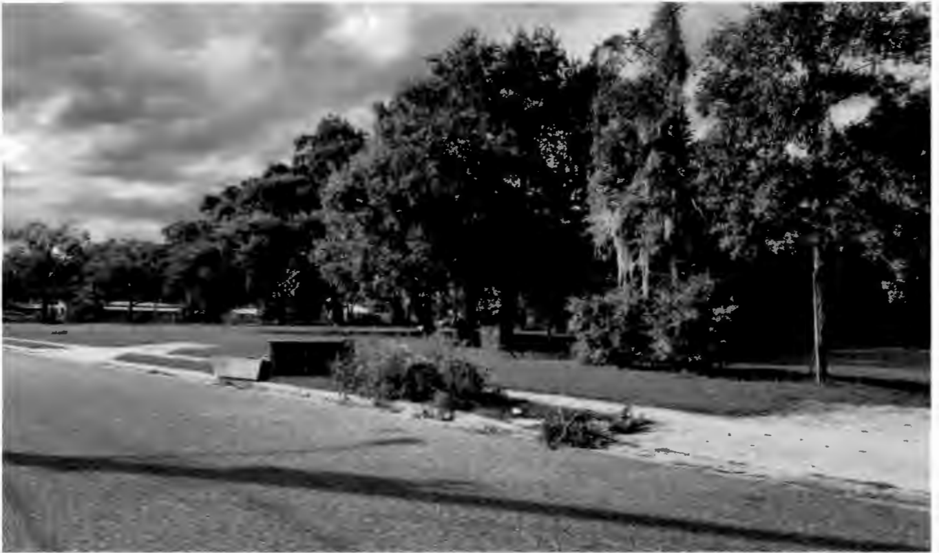
Facing northwest from 23 rd St. towards subject property
