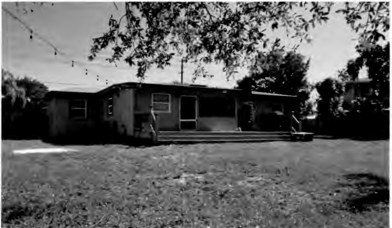
Rear yard, facing northeast towards proposed Addition #5
