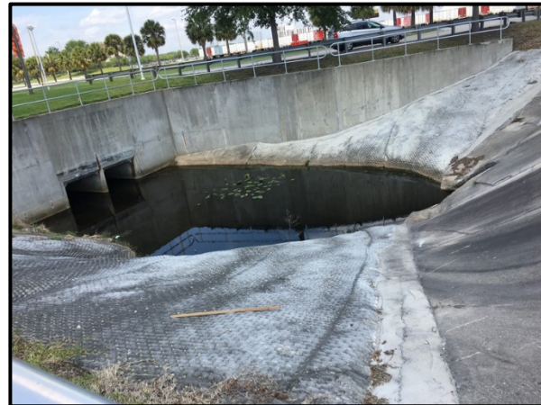
Upstream end of the 84-inch RCP culvert crossing (west of Tradeshow Boulevard).
