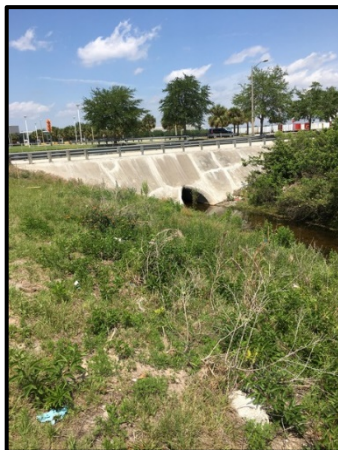
Downstream end of the 84-inch RCP culvert crossing (east of Tradeshow Boulevard).
