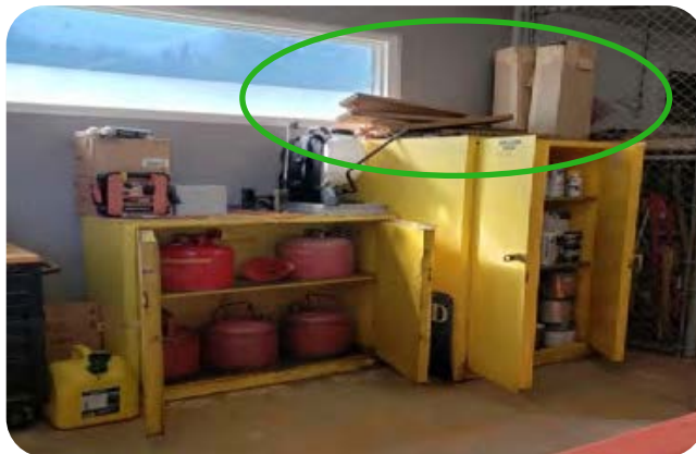
Cardboard on top of flammable cabinets
