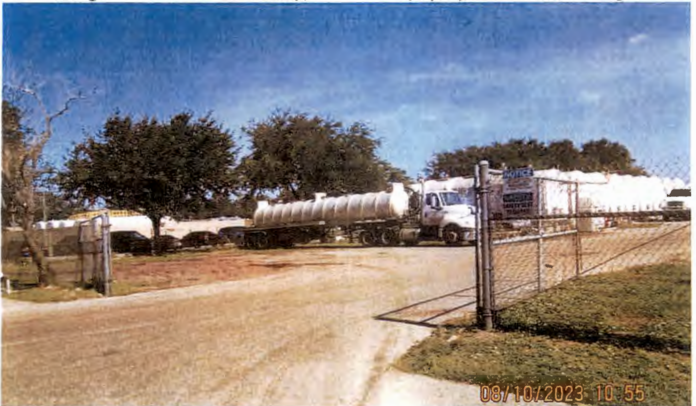
Facing north at entrance from Central Florida Pkwy., towards processing tanks
