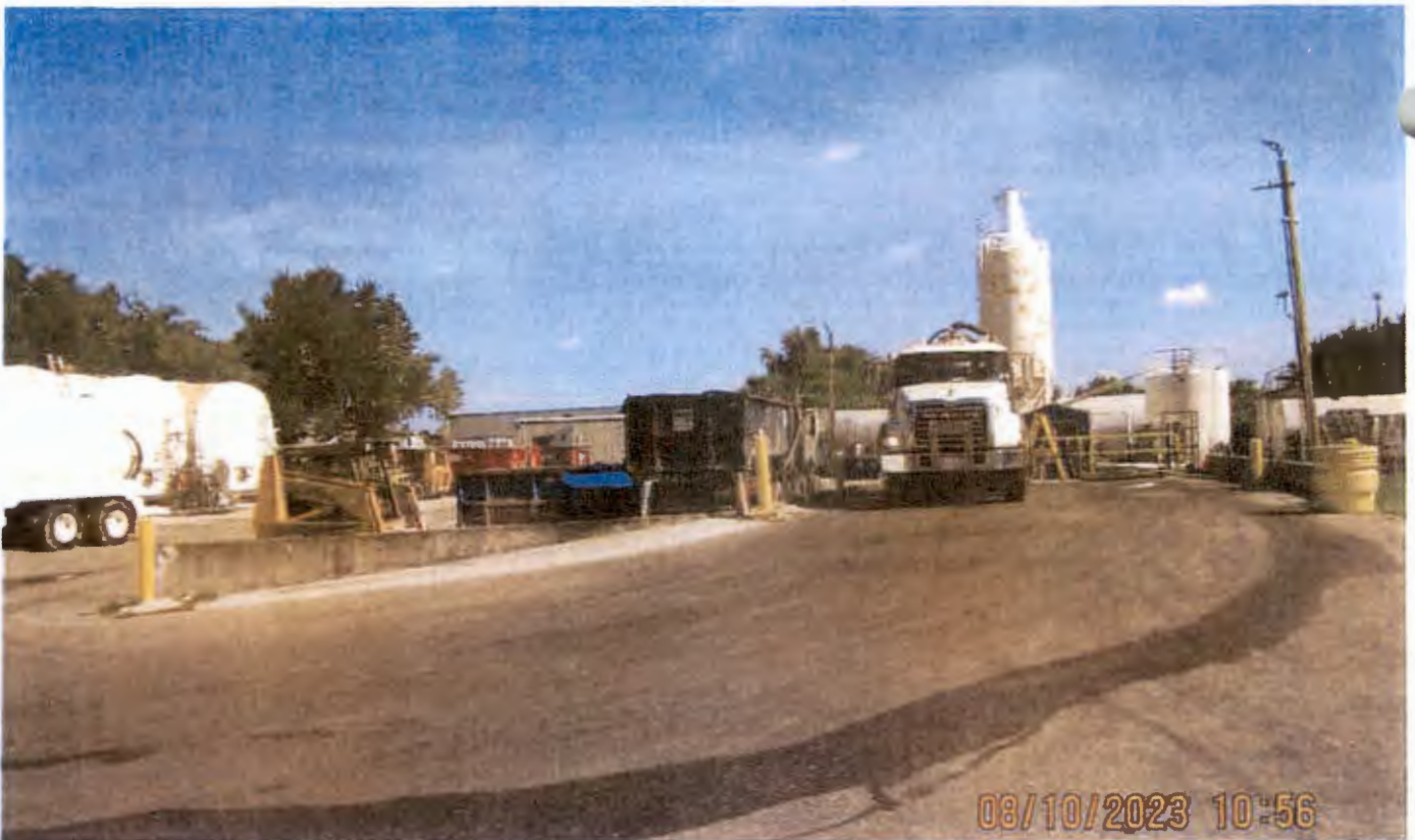
Within center of site facing towards parking area, internal circulation and tanks, left & right and silo at rear
