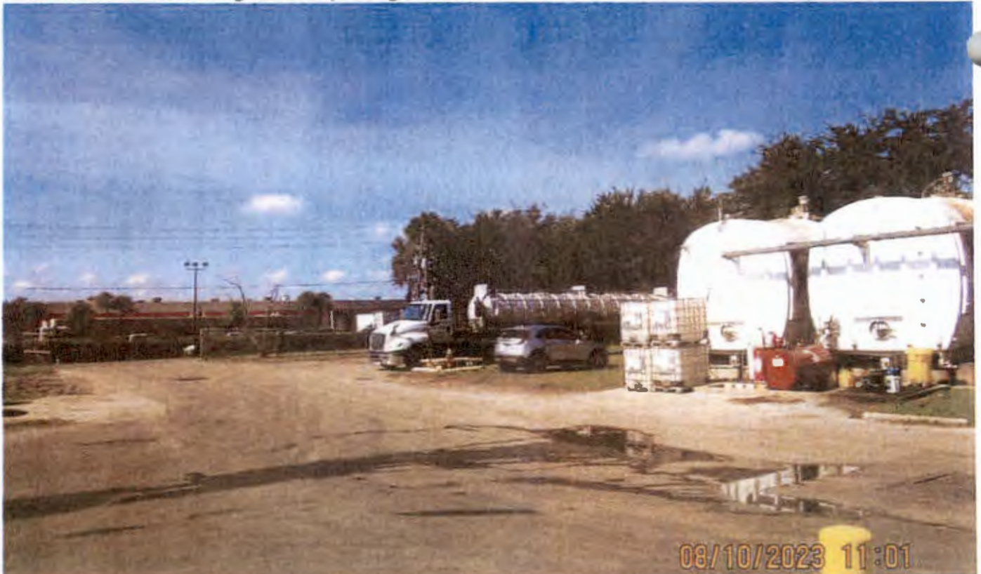
Facing south towards entrance & chemical site across the street, tanks to the right
