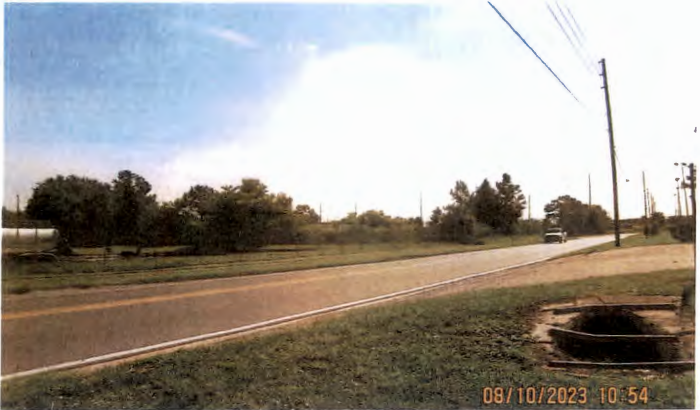
Facing east from Central Florida Pkwy., to east side of property, chemical site, to the right
