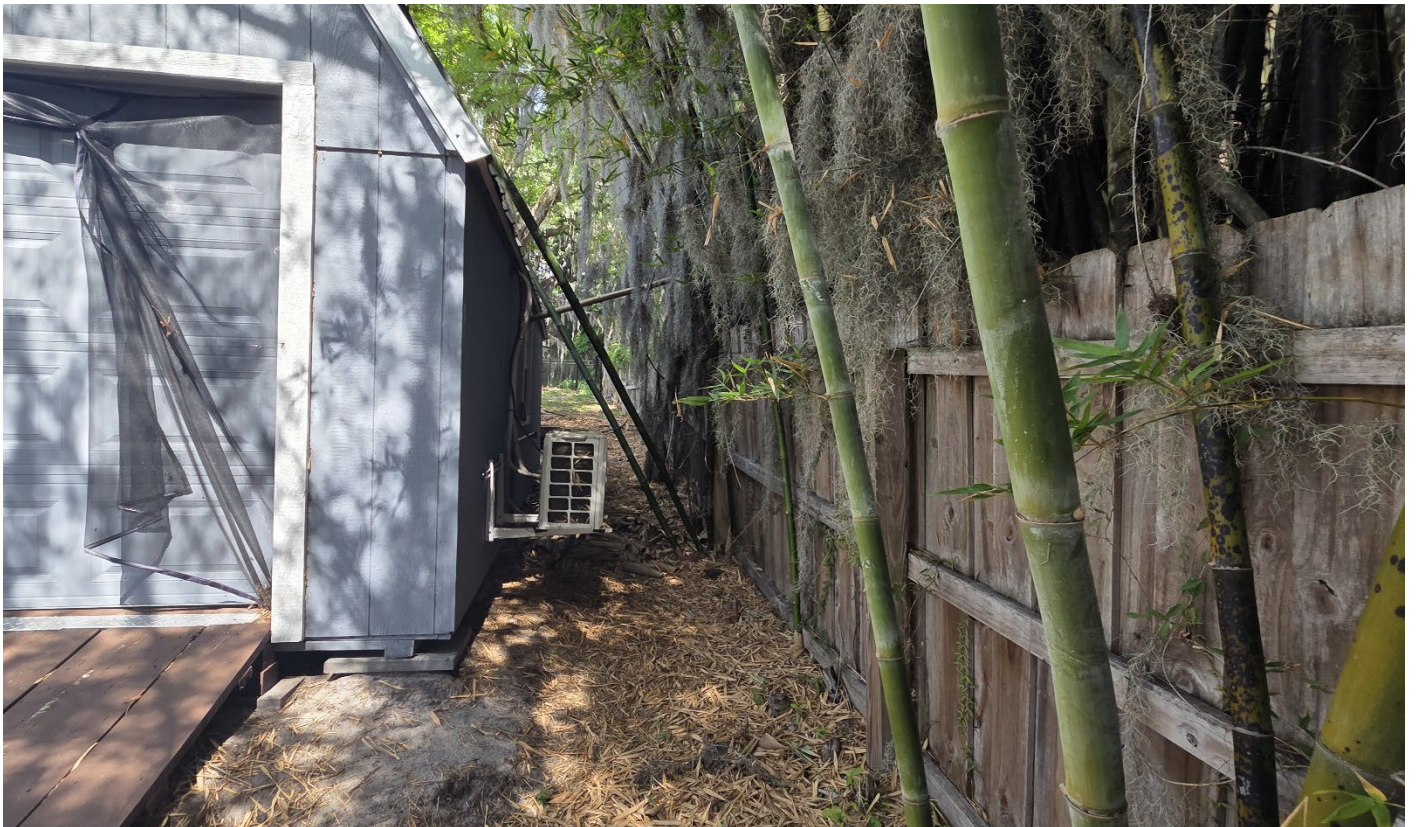
Facing west towards the side of the existing structures (shed and greenhouse)
