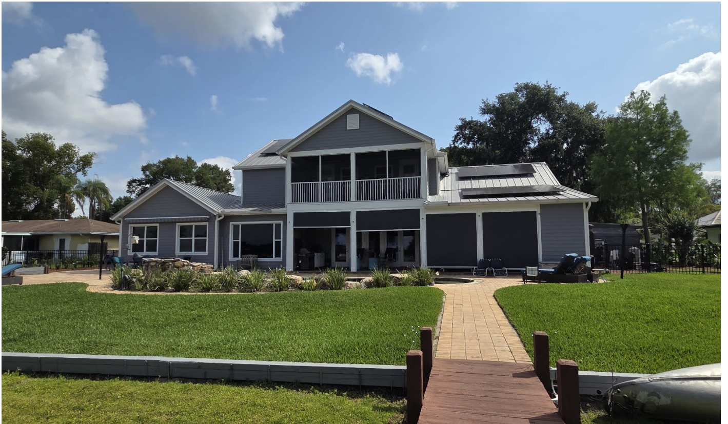
Rear yard, facing east towards the existing residence
