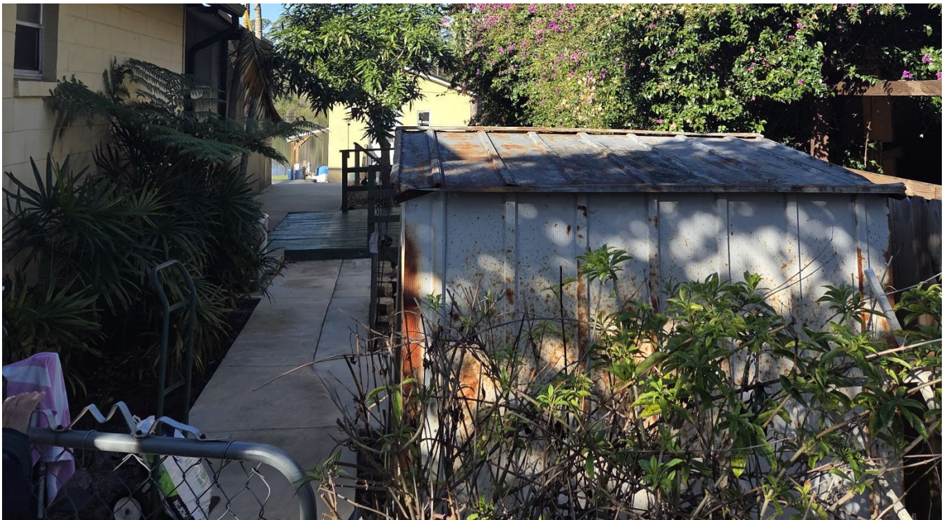
Facing west towards Shed 2 (to be removed) and side walkway
