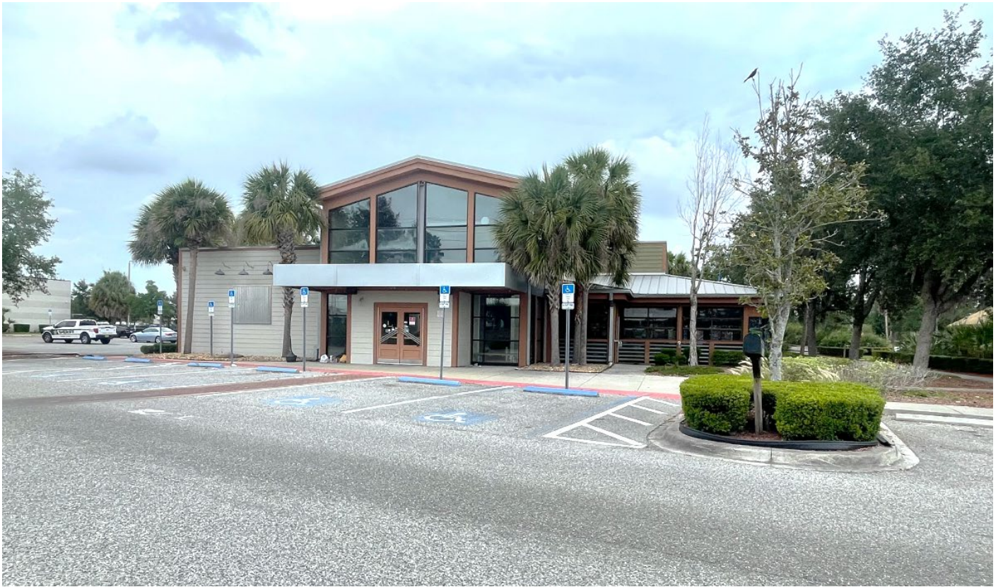
Facing northwest along W Irlo Bronson Hwy toward the front of the subject property
