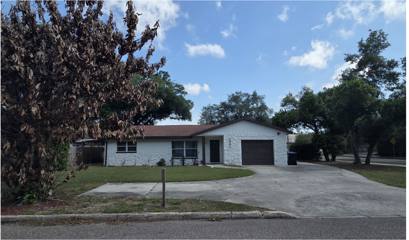
Sunshine St., facing north towards front of subject property
