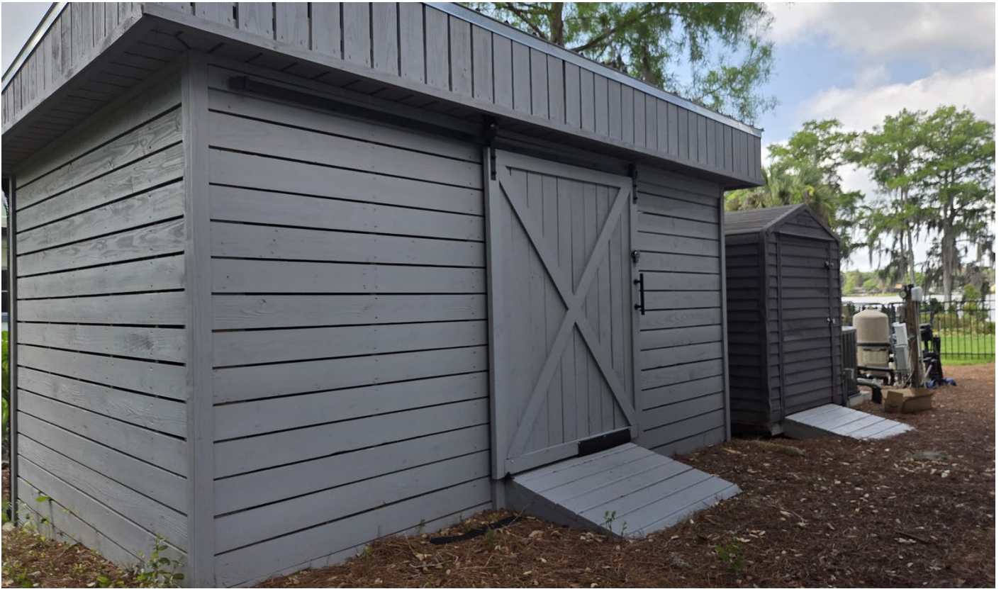
Side yard, facing southwest towards both existing sheds
