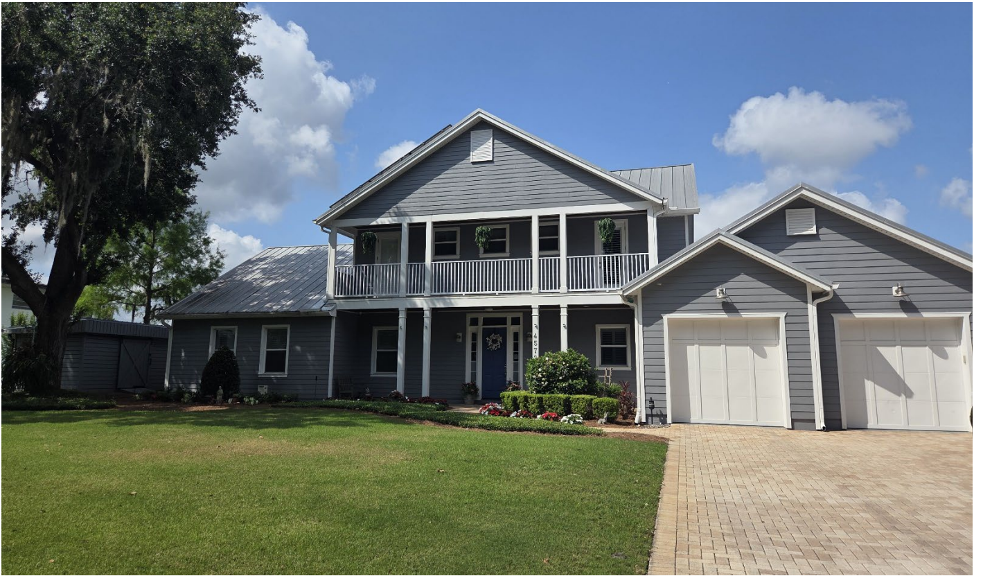
Front yard, facing west towards front of subject property
