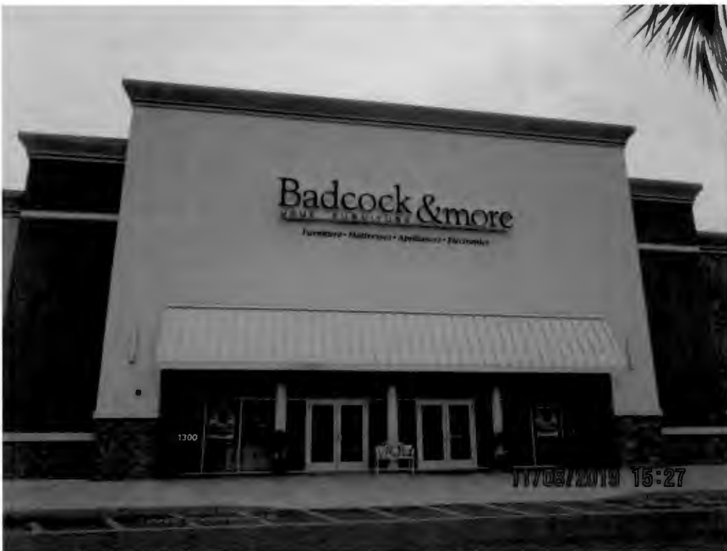
Close, detailed view of existing wall sign
