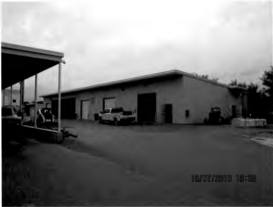
Existing Maintenance Building Looking Southwest
