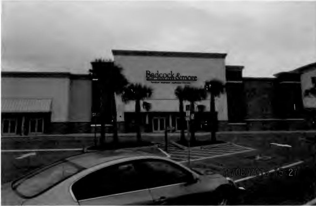
Subject site showing 153.9 sq. ft. wall sign as it exists today
