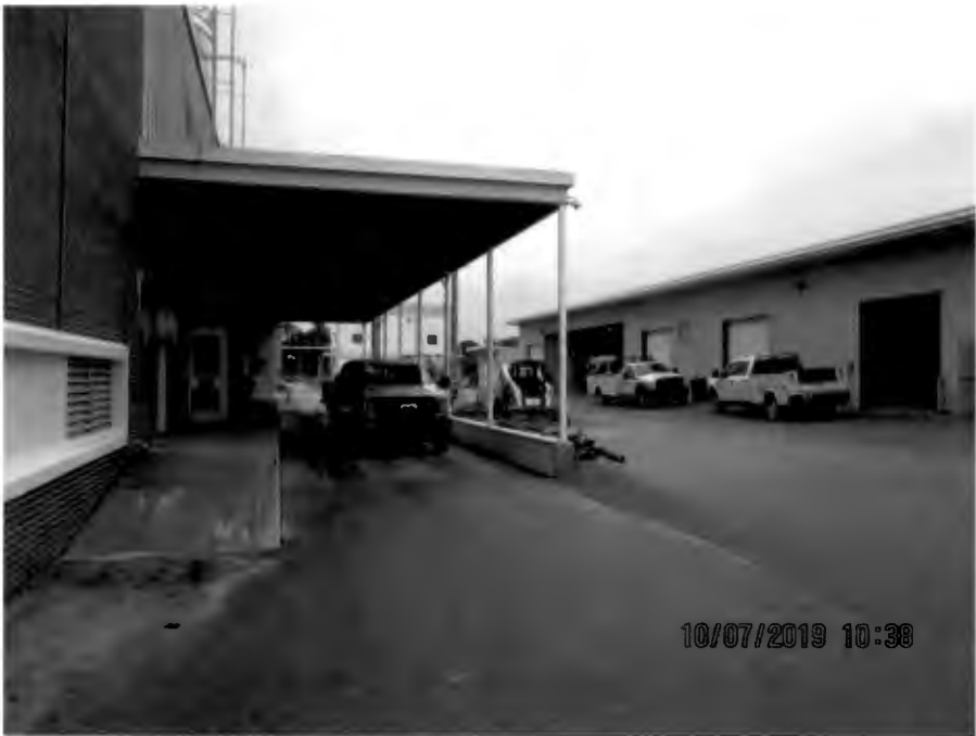
Maintenance Building and Receiving Building Looking South
