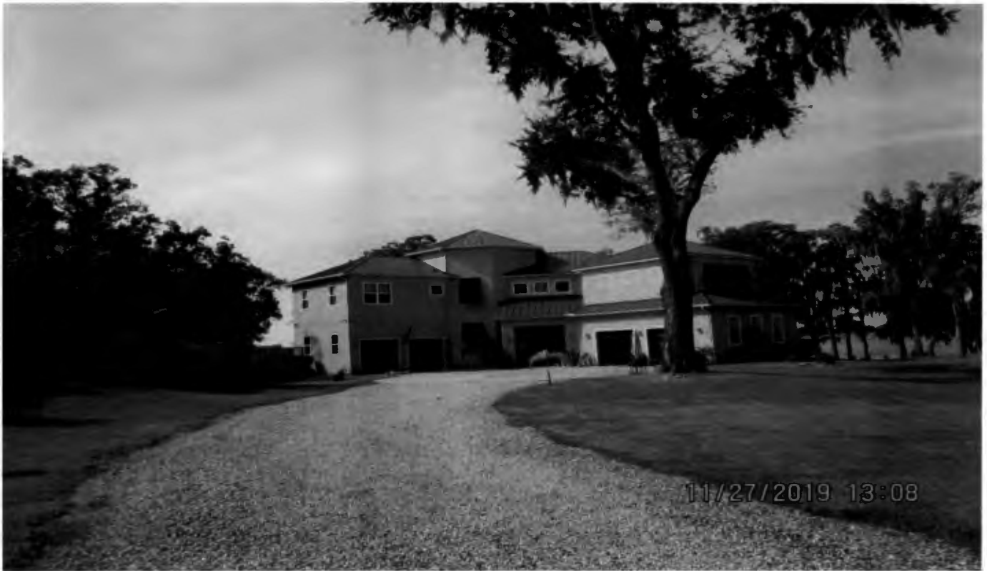
Subject Property Looking West
