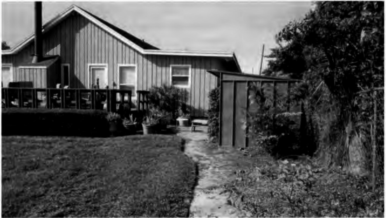
Rear shed to be removed
