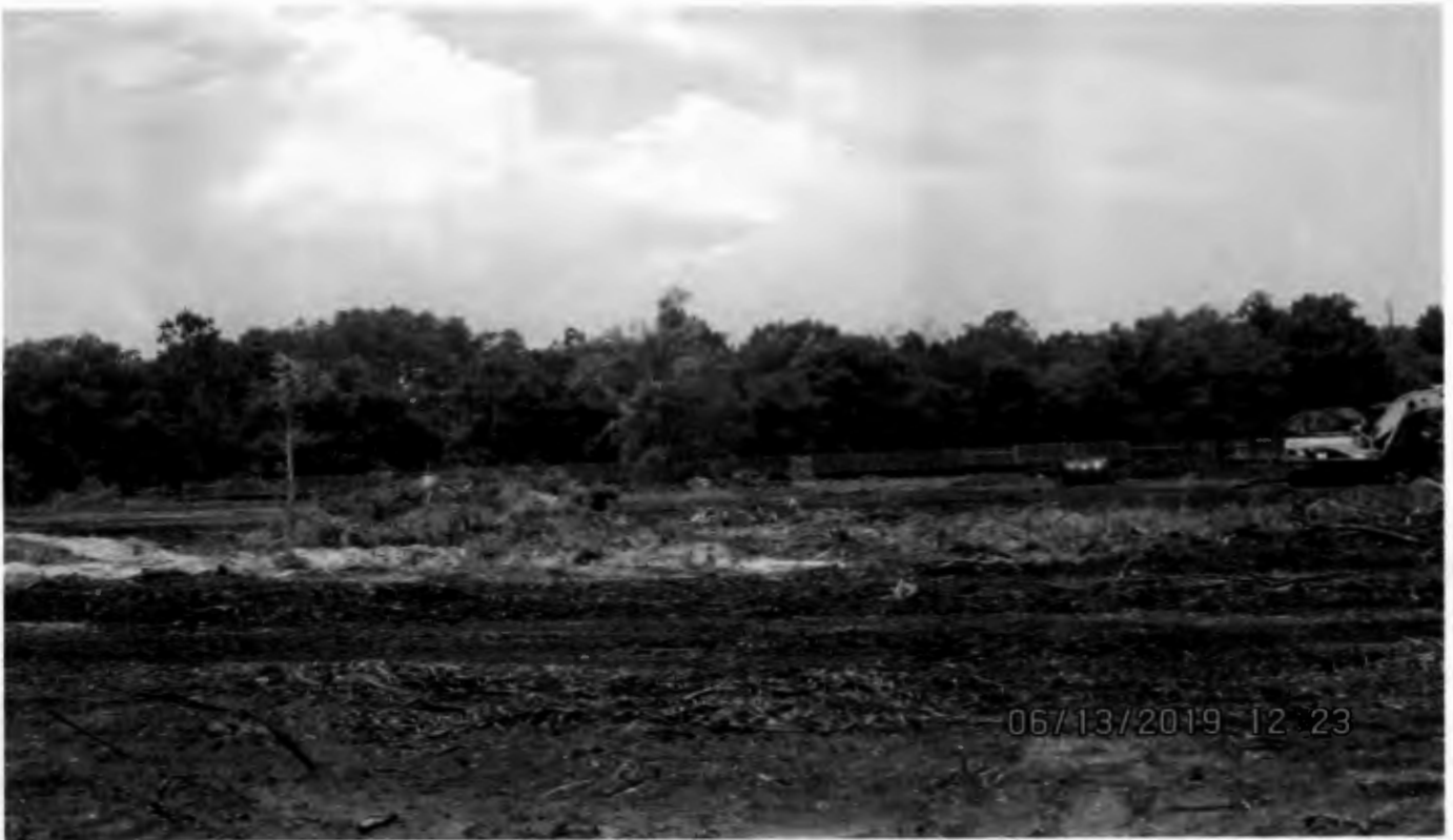
Site Looking South, Taken From Parkers Landing
