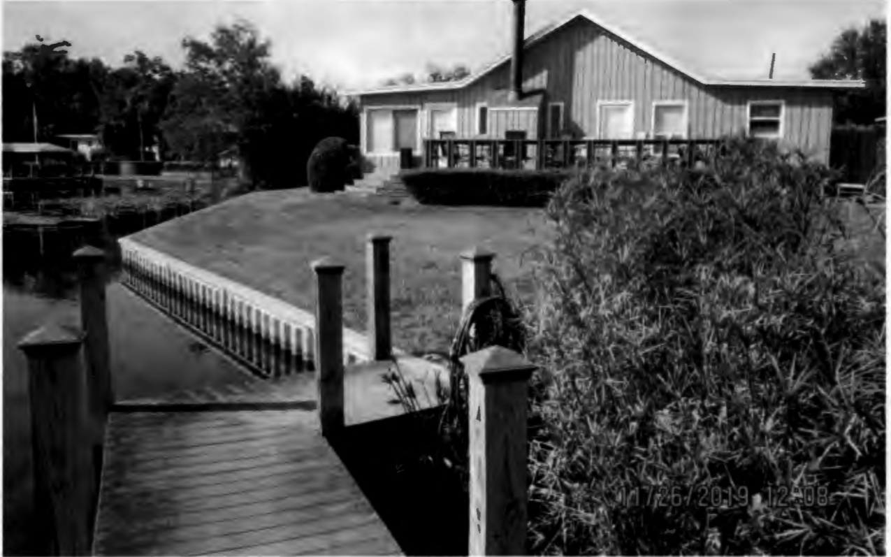
Rear deck and stairs adjacent to Little Lake Fairview
