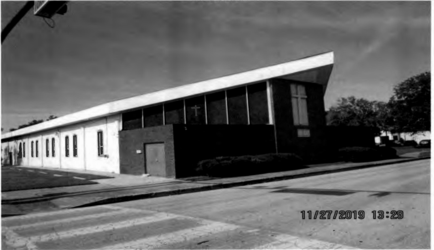
Location of Proposed Shared Parking Looking Northwest
