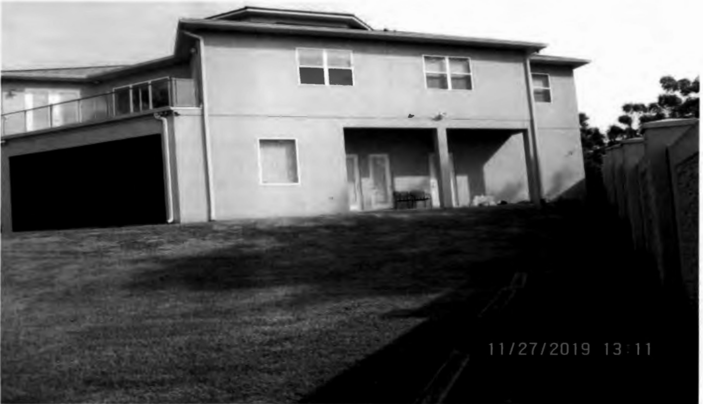
View from Bottom of Slope Looking East
