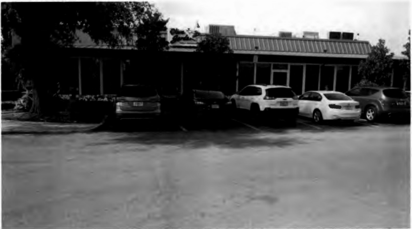
Side facing interior. Elevation C
