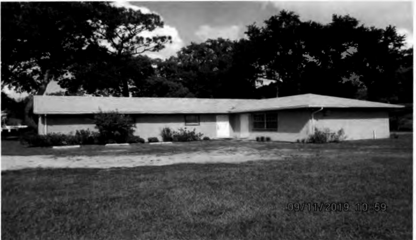
Existing Sanctuary and Multipurpose Room Looking West
