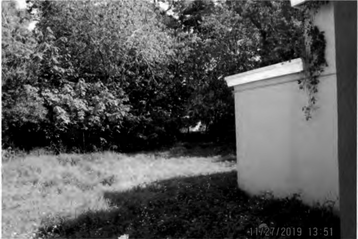
Rear Yard Looking East
