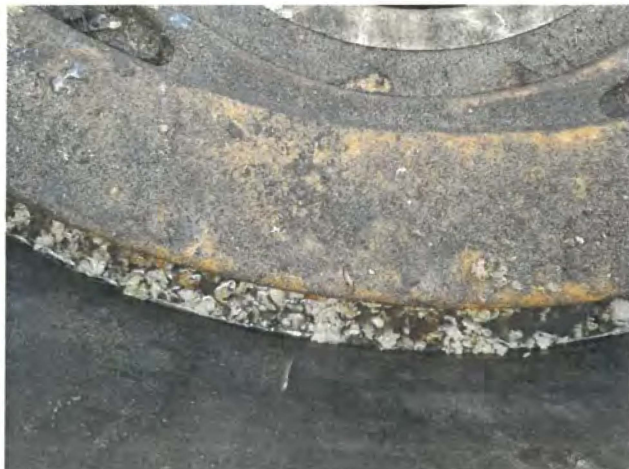
Sealant Tank 3 Fill
