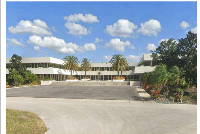
View of the Tupperware facility main entrance, facing east.
