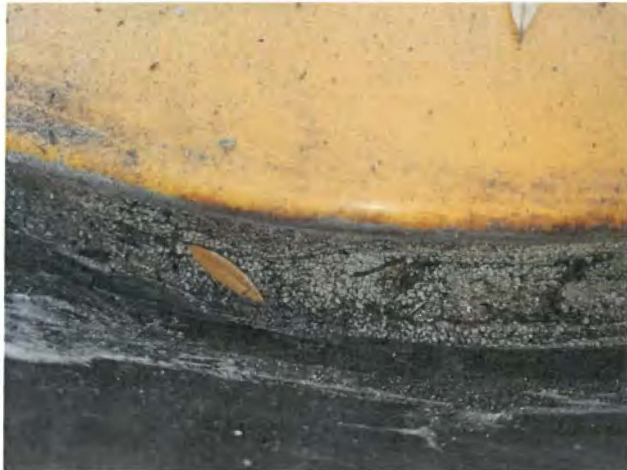
Sealant Tank 2 Fill
