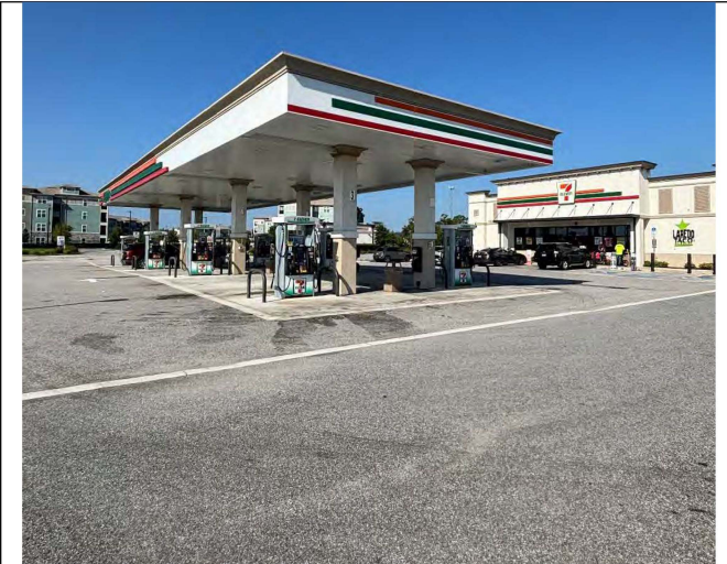
View of the 7-Eleven dispenser islands and store, facing southwest.
