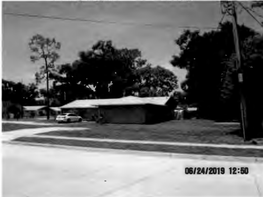
Subject Property Looking Southwest
