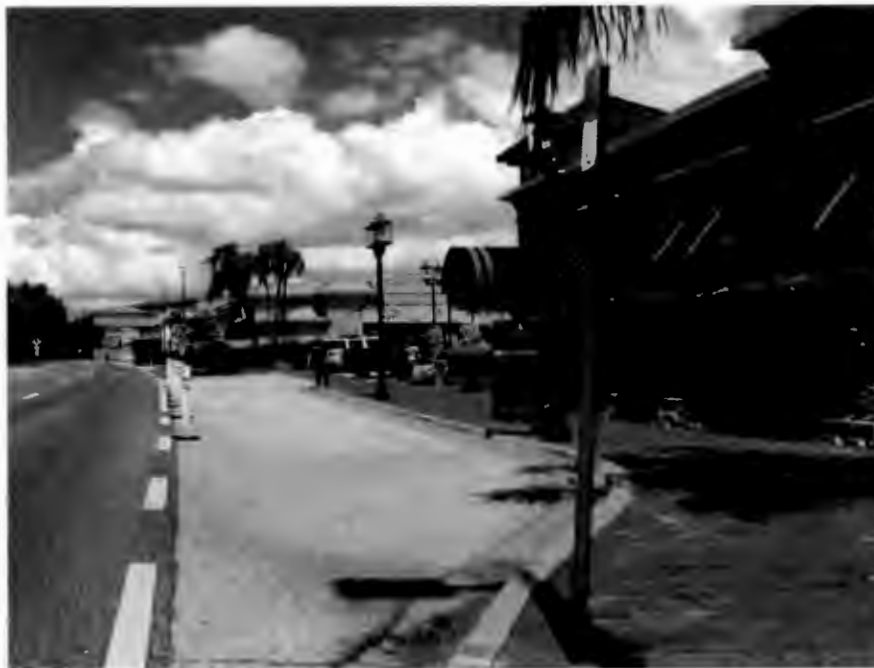
View from International Drive (west side of property), facing north. Showing view approaching Valet Plaza # 1
