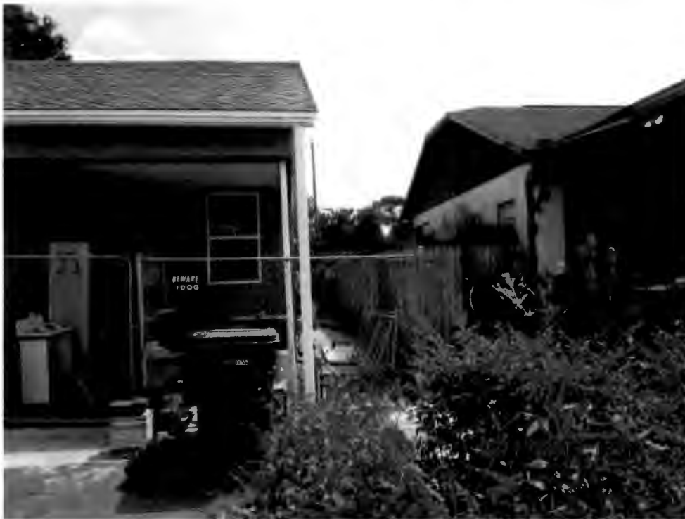
Carport and Side Setback Looking East
