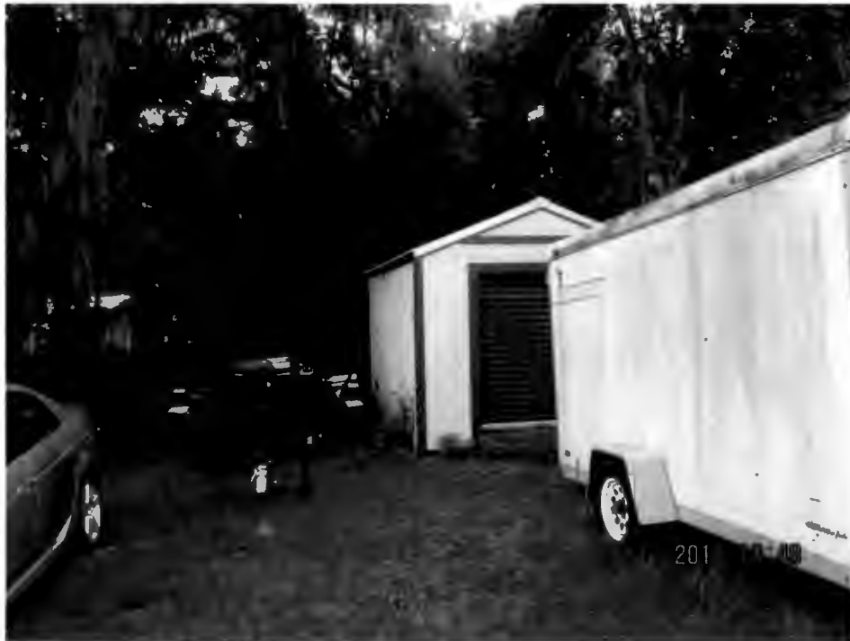
South Side and Front of Shed Looking West
