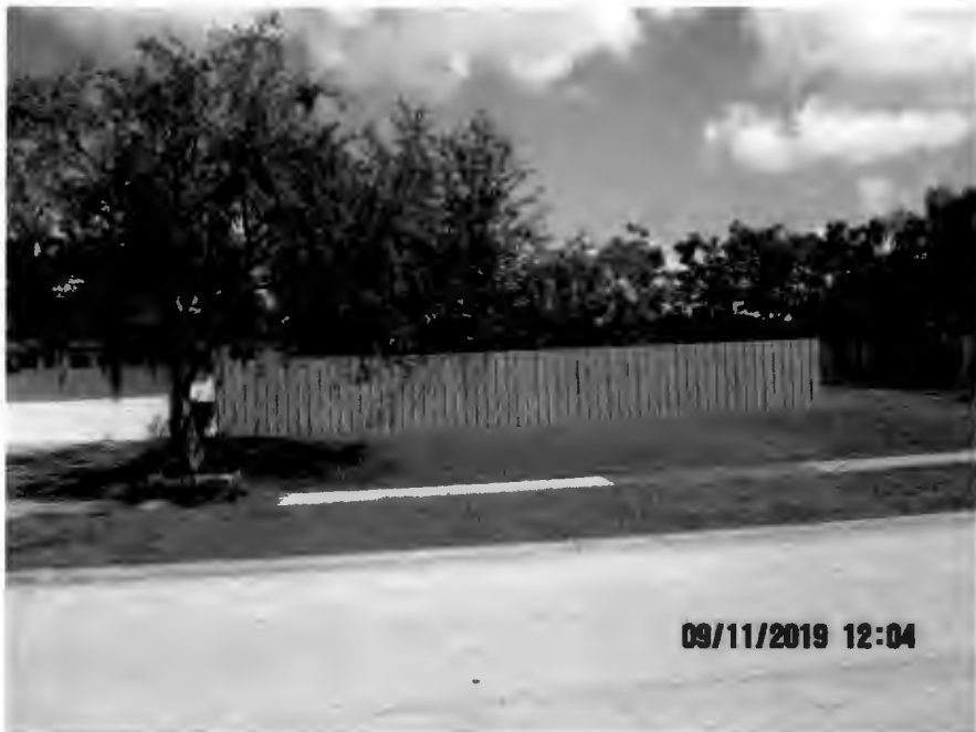
Screening Fence Looking North
