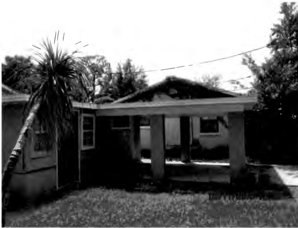
Carport and Neighboring Home Looking South
