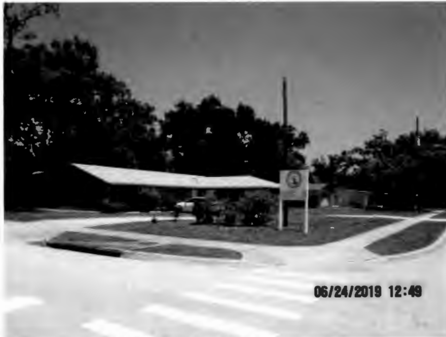
Existing Sanctuary Looking Northwest
