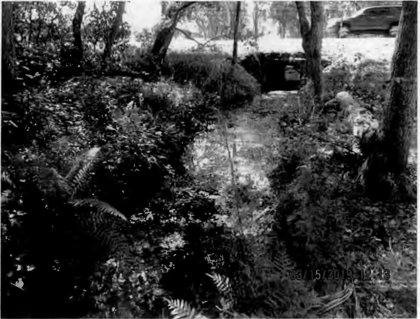
Ditch Looking towards front of property
