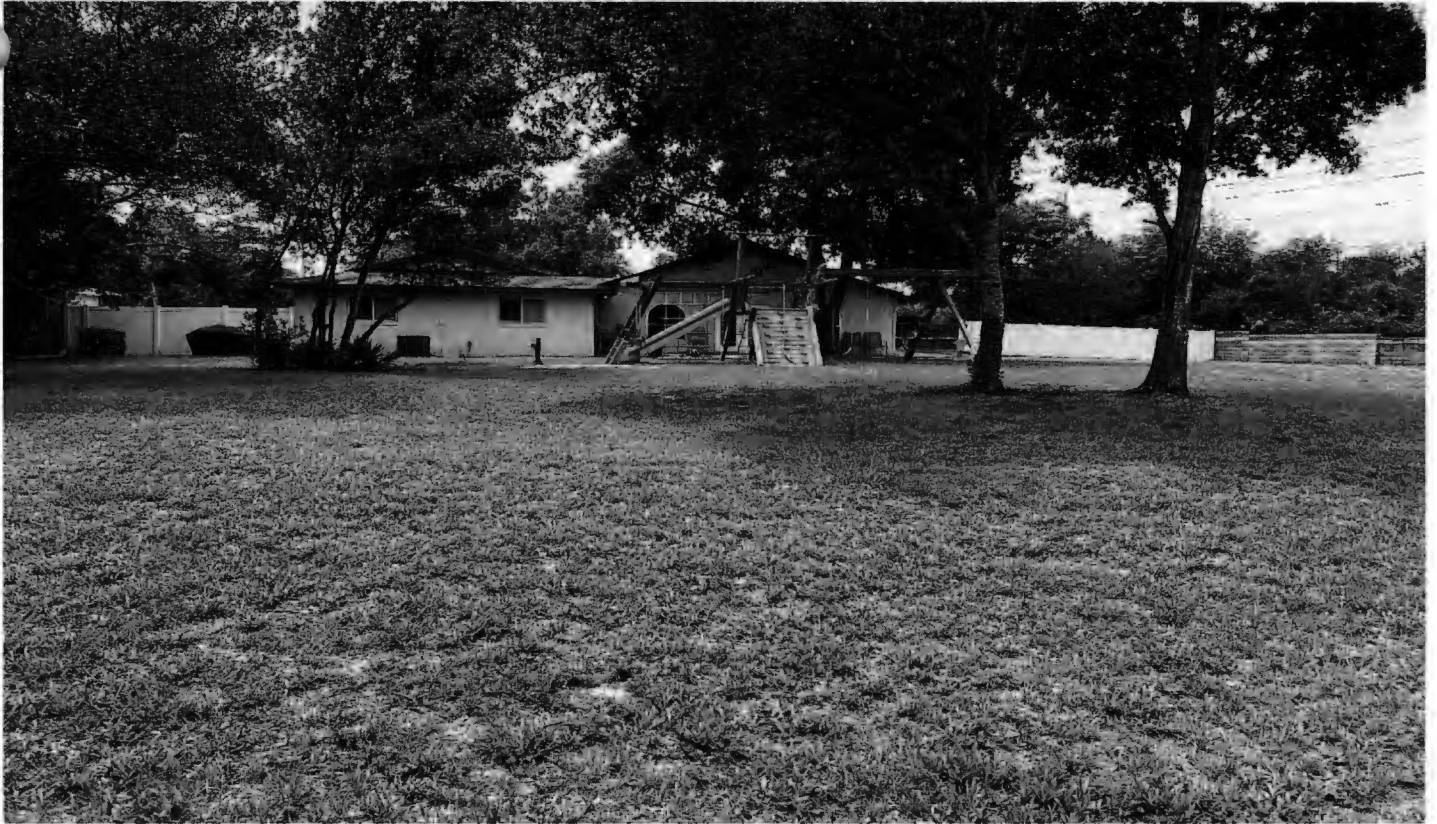
Rear of the house looking toward the proposed parking area entrance and parking area
