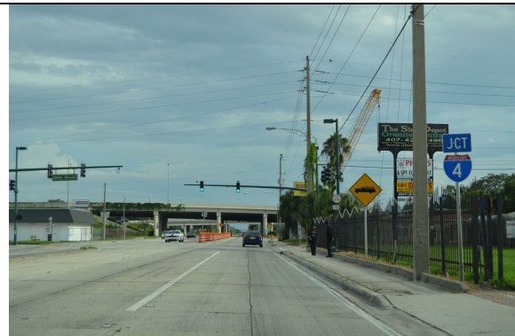
(OBT CRA Area- Picture 20) 29 th Street intersects OBT at a signal preceding westbound on-ramp for Interstate 4. 29 th Street parallels the freeway west.
