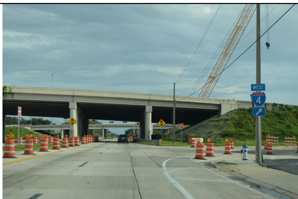
(OBT CRA Area- Picture 21) From 29 th Street on OBT I-4 Ultimate construction through 2021 reconfigures the directional cloverleaf interchange with U.S. 17-92-441 to accommodate the Express toll lanes. There is no direct access to I-4 east from OBT southbound.
