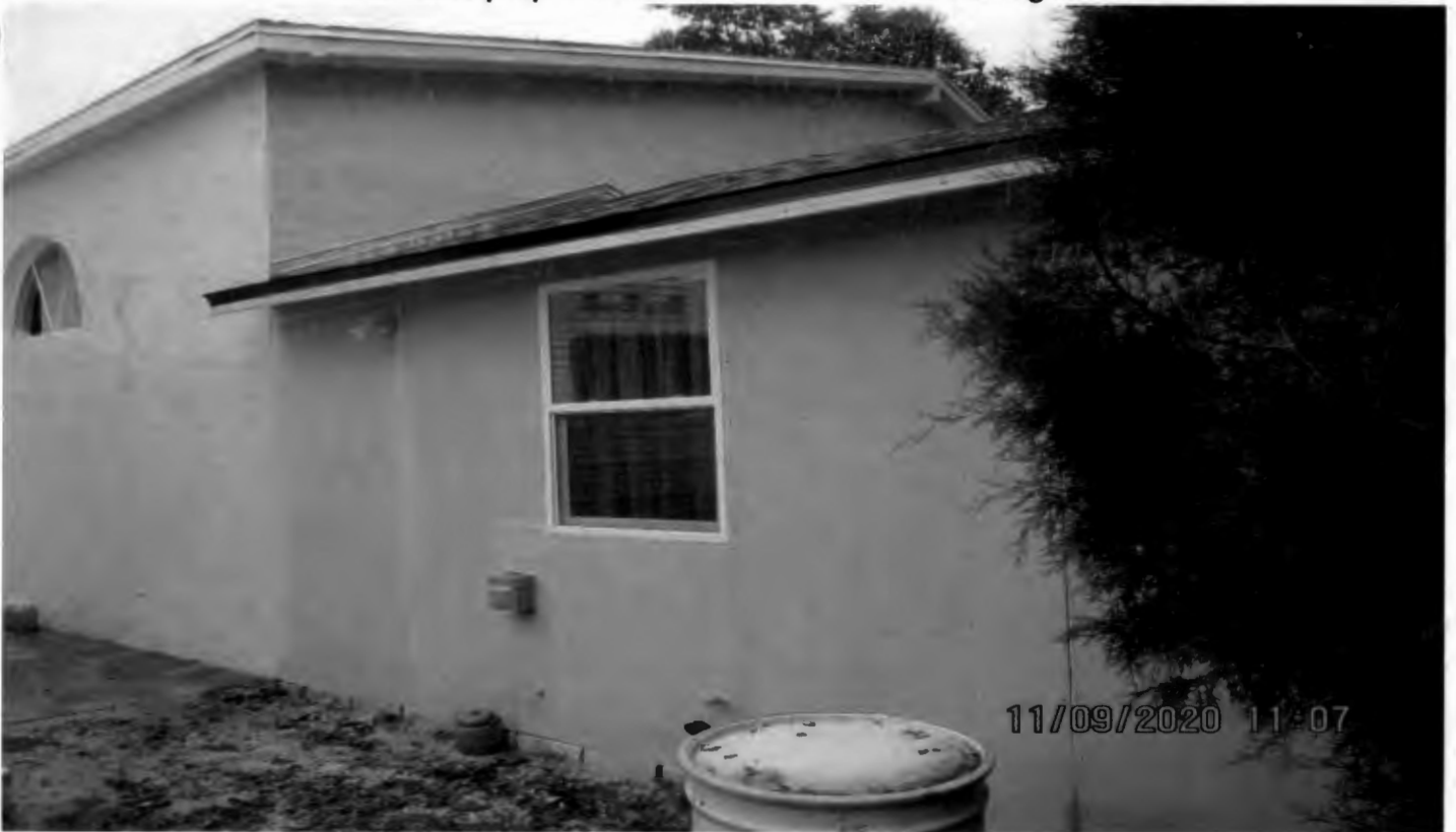
Side of addition looking northeast
