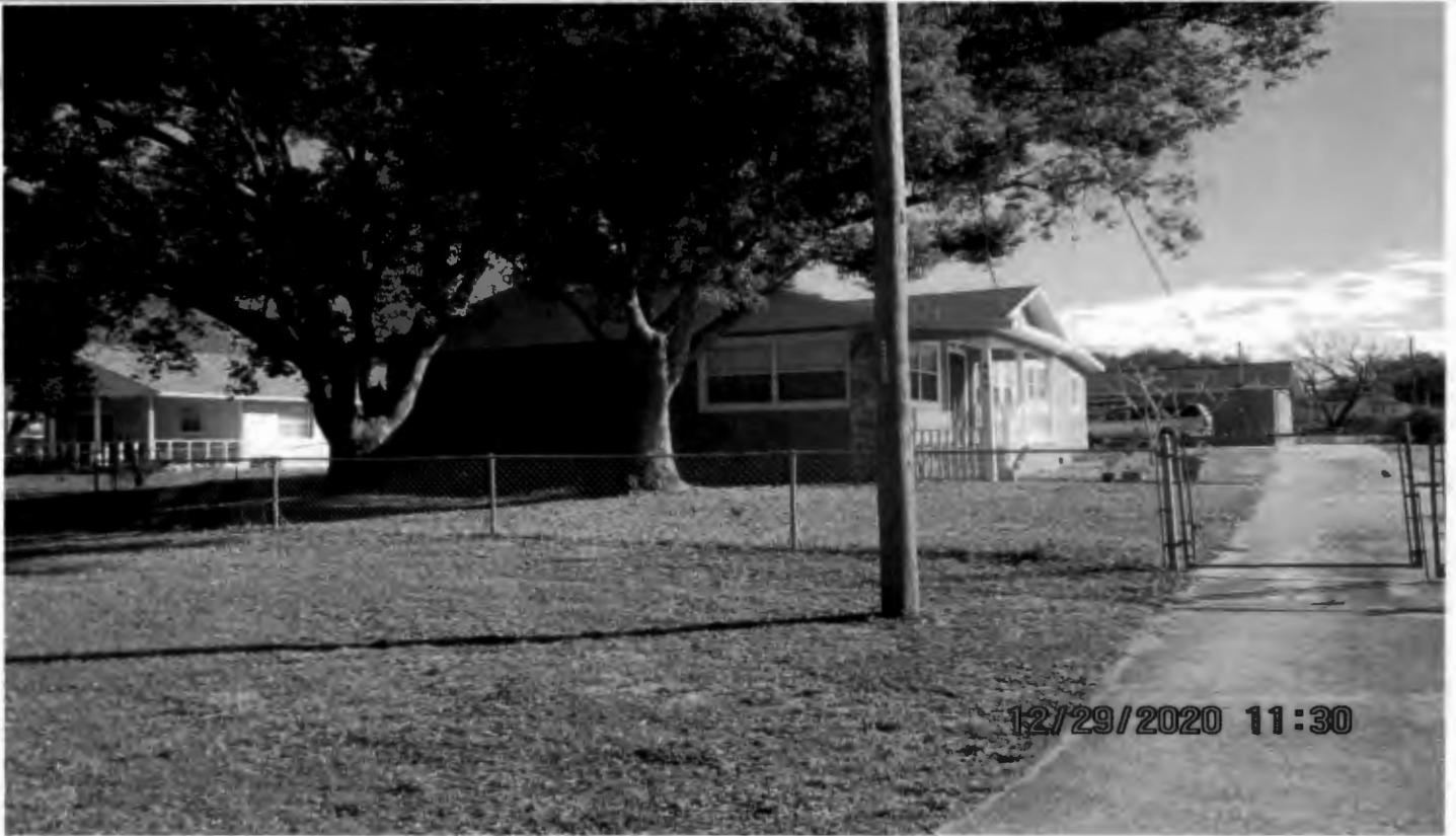
Subject property looking east from 1 st St.
