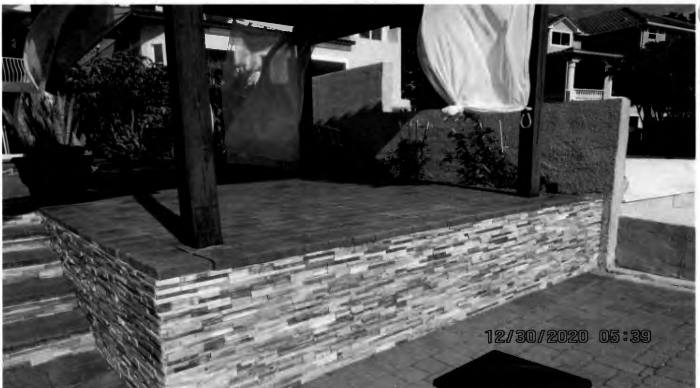
2/4/2021 BZA-Wall reduced to 4 ft. within NHWE setback, looking north
