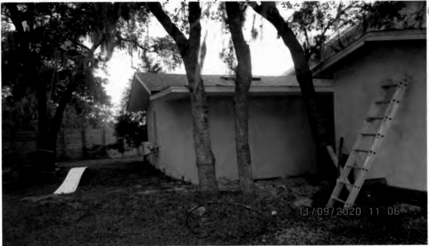
Addition looking west
