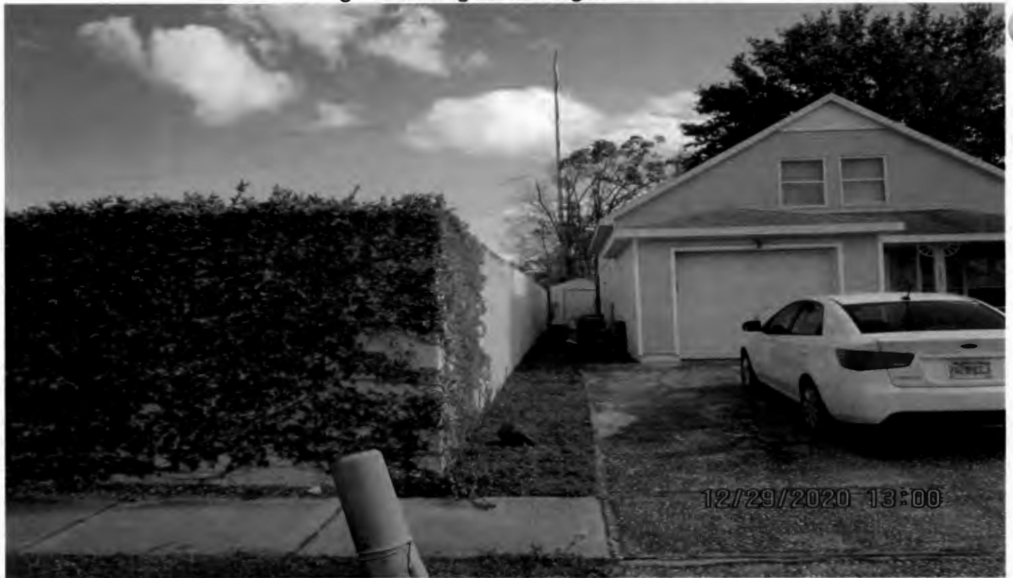
Wall extending east along the side property line looking east
