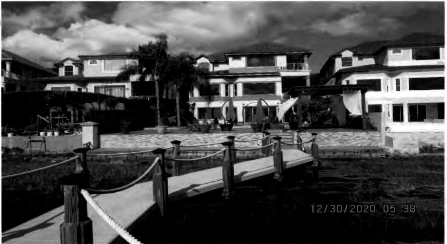
Rear, looking north
