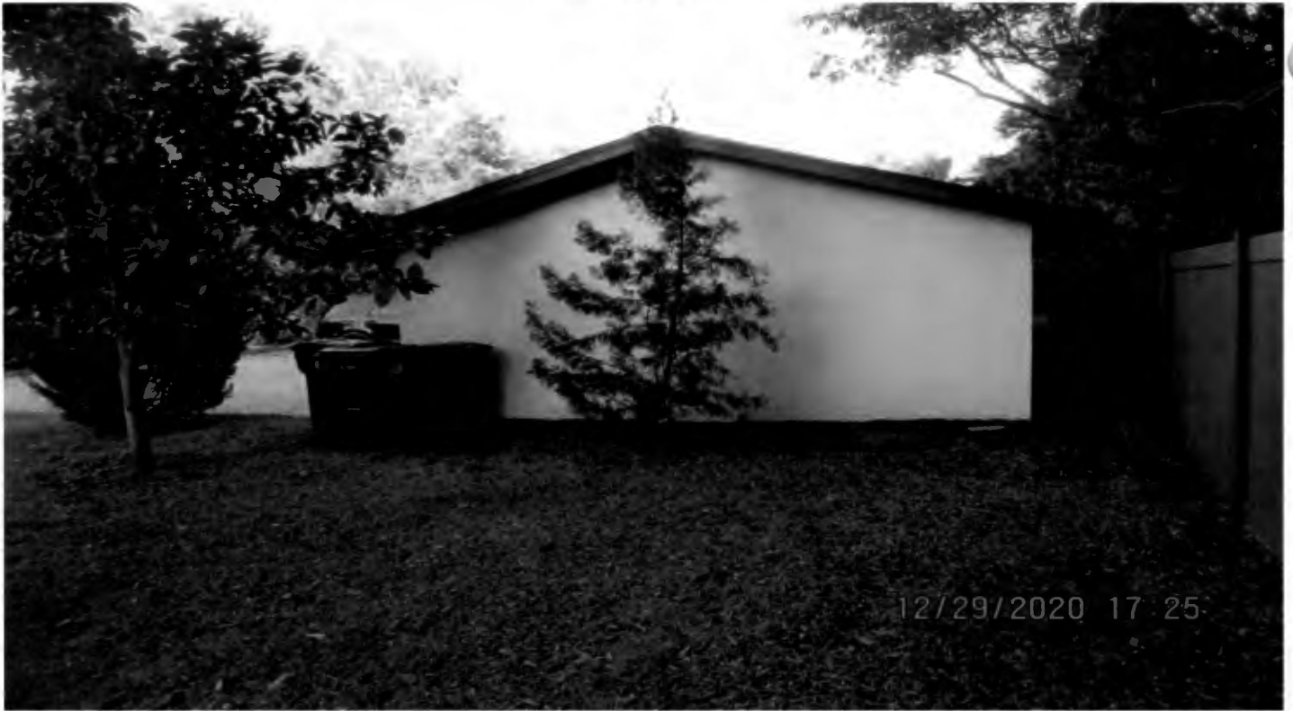
View of garage facing east, with 3.1 ft. setback on south side
