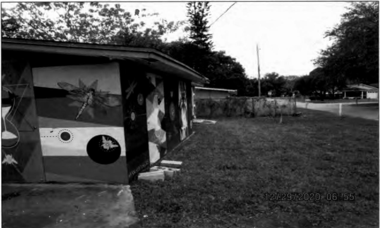
North side of existing structure requiring Variance #6, facing west
