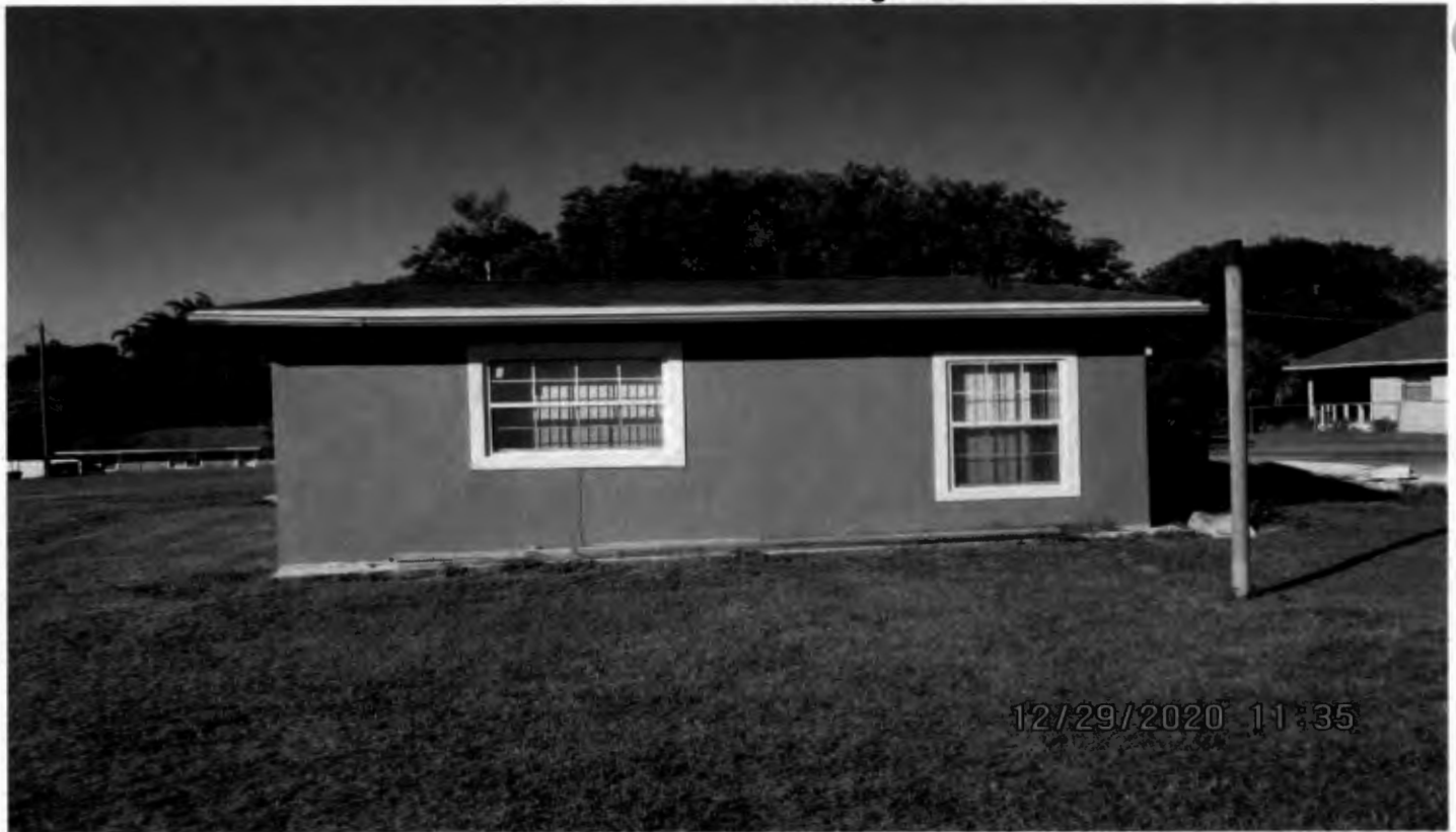
Rear of ADU looking west
