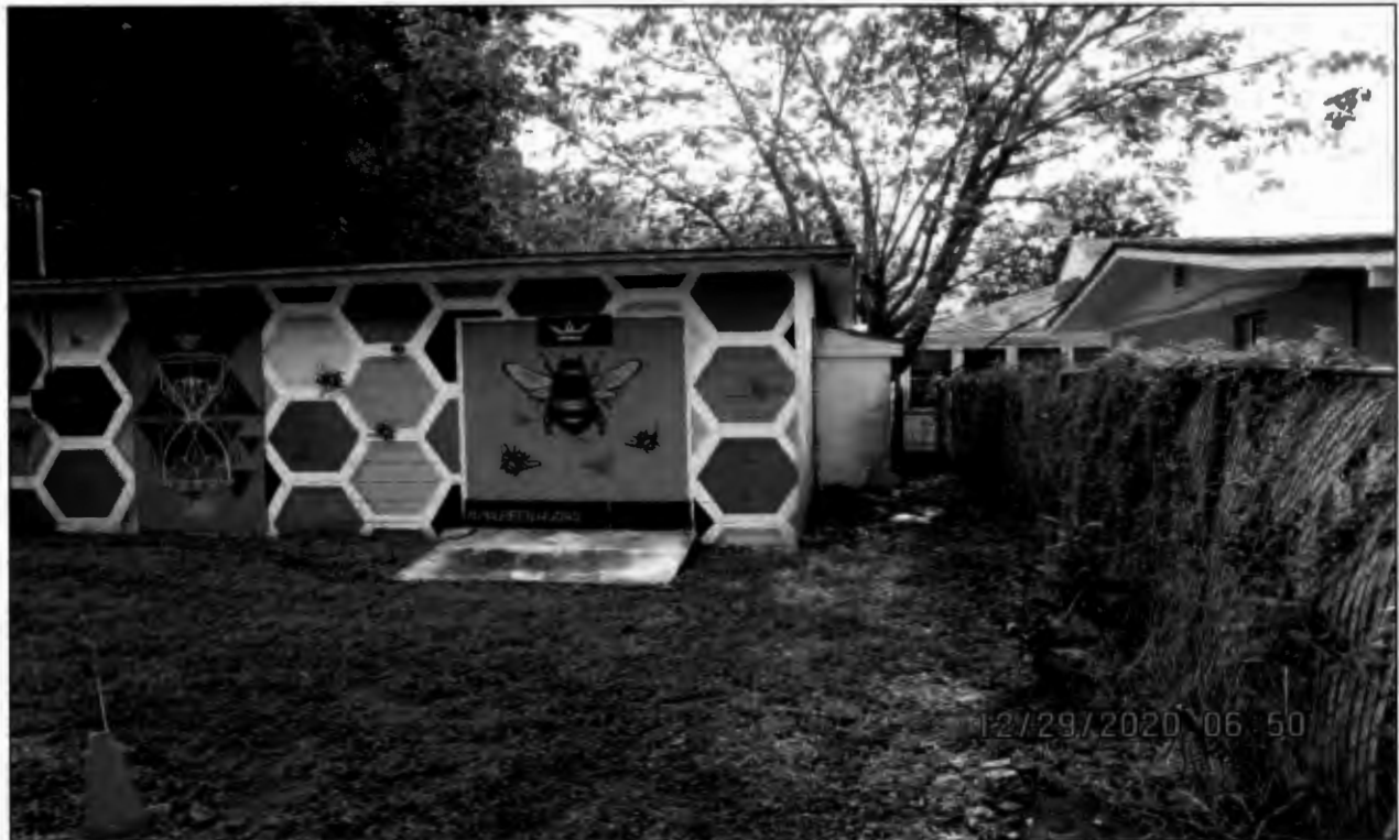
Facing south towards existing structure from Vine St.
