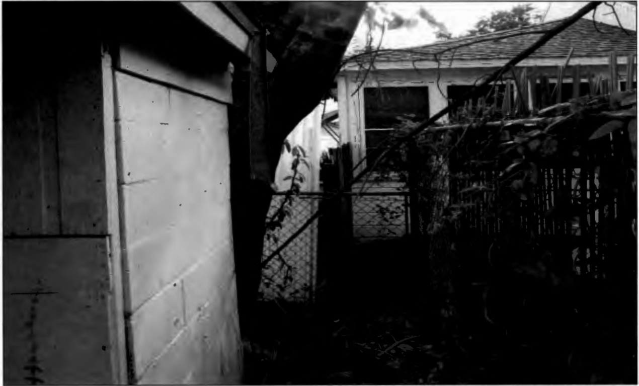
West side of existing structure requiring Variance #5, facing south
