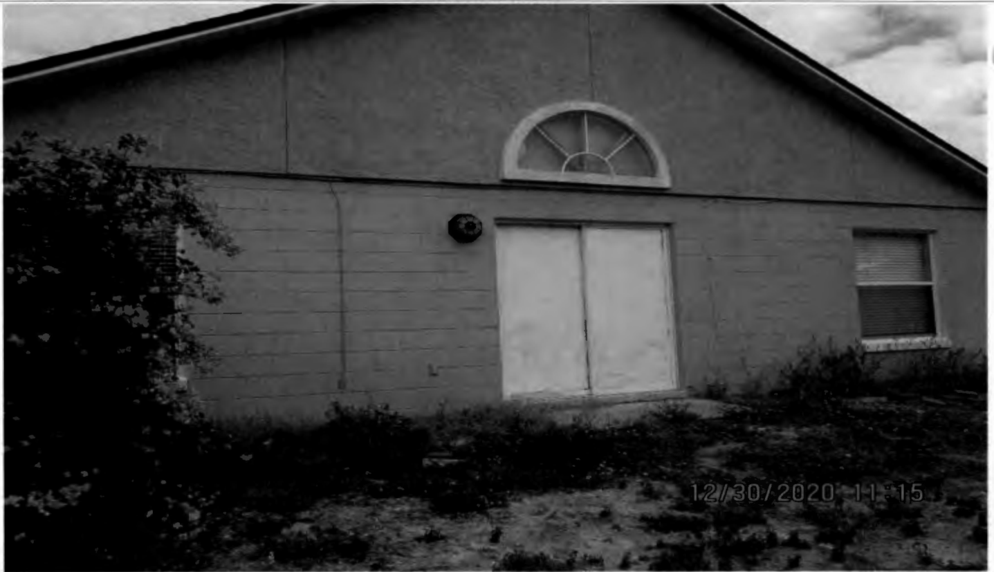
Proposed location of addition looking northeast
