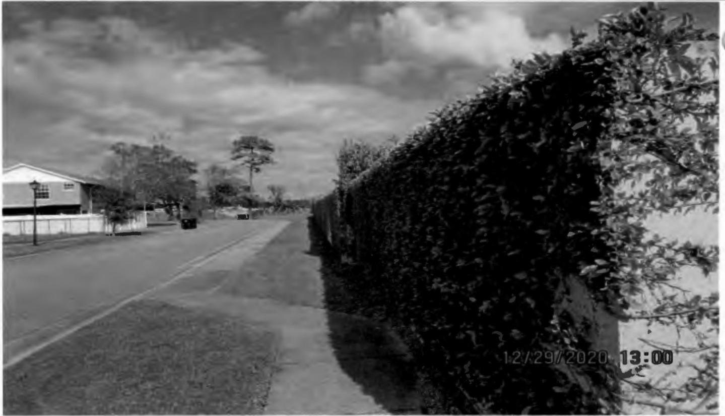
Existing wall looking north along Dearmont Ave.
