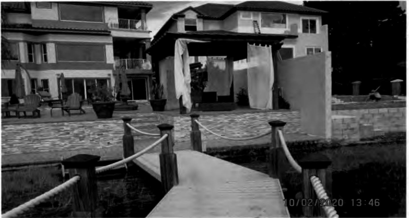
11/5/2020 BZA-10 ft. wall within NHWE setback, and pergola with 2 ft. east side setback, looking north
