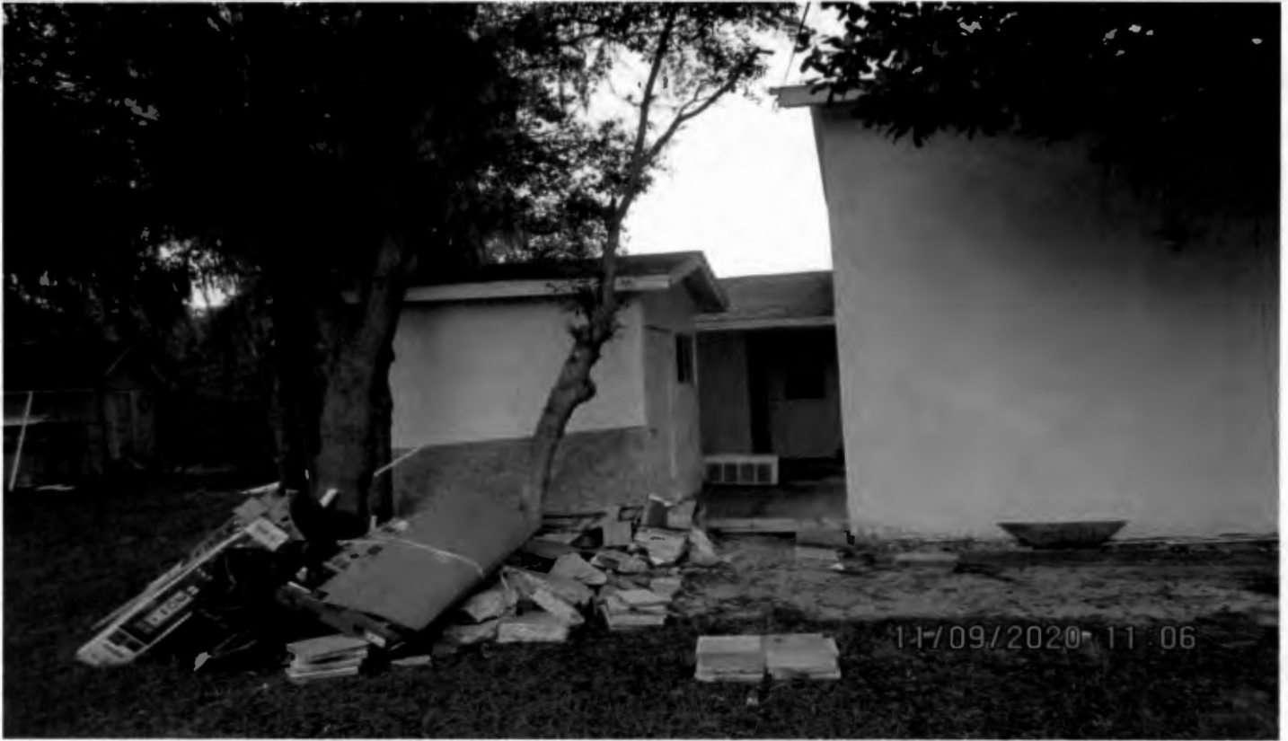
Small shed proposed to be attached to home looking west
