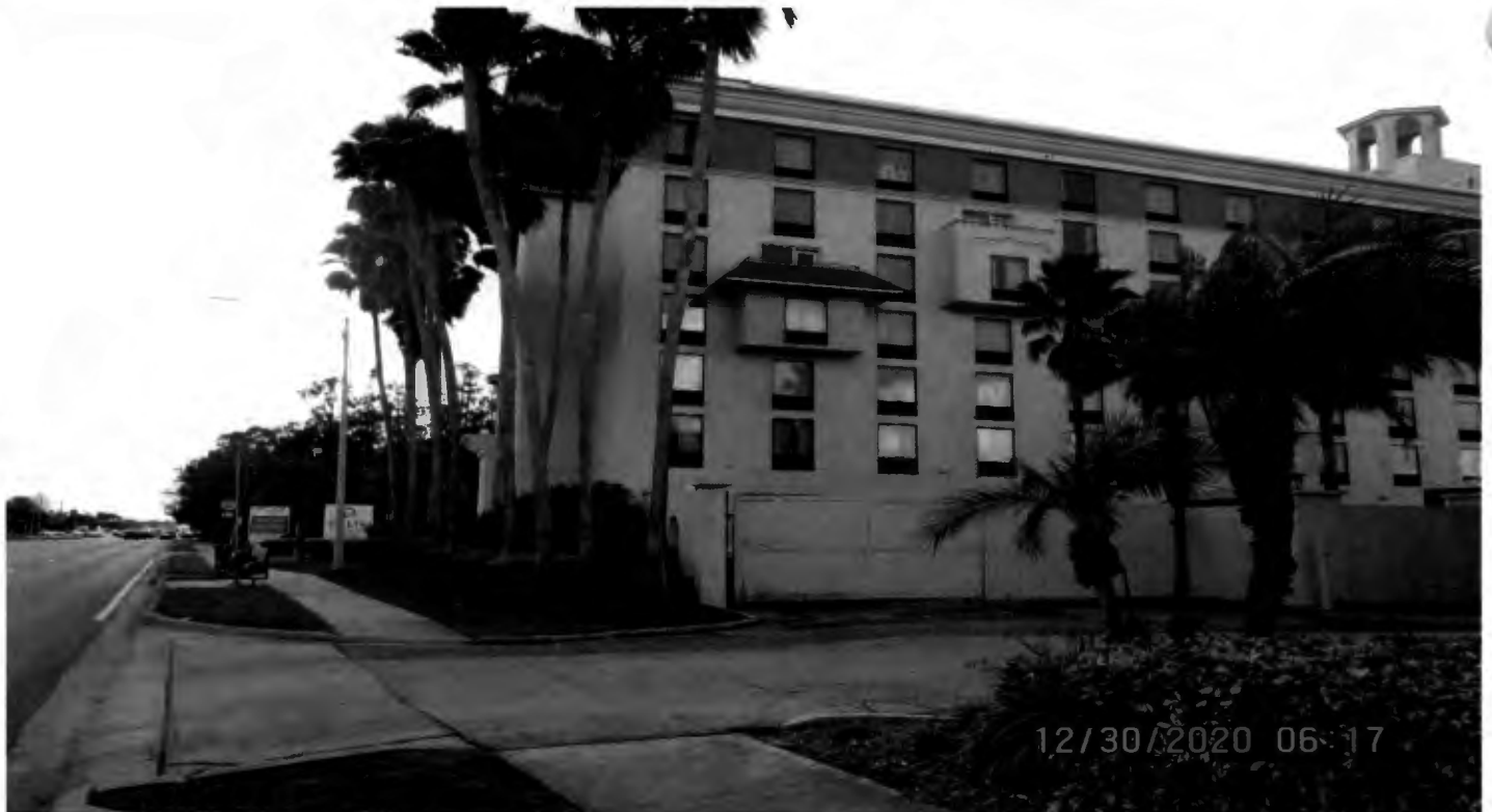
Proposed location of laundry room addition looking south
