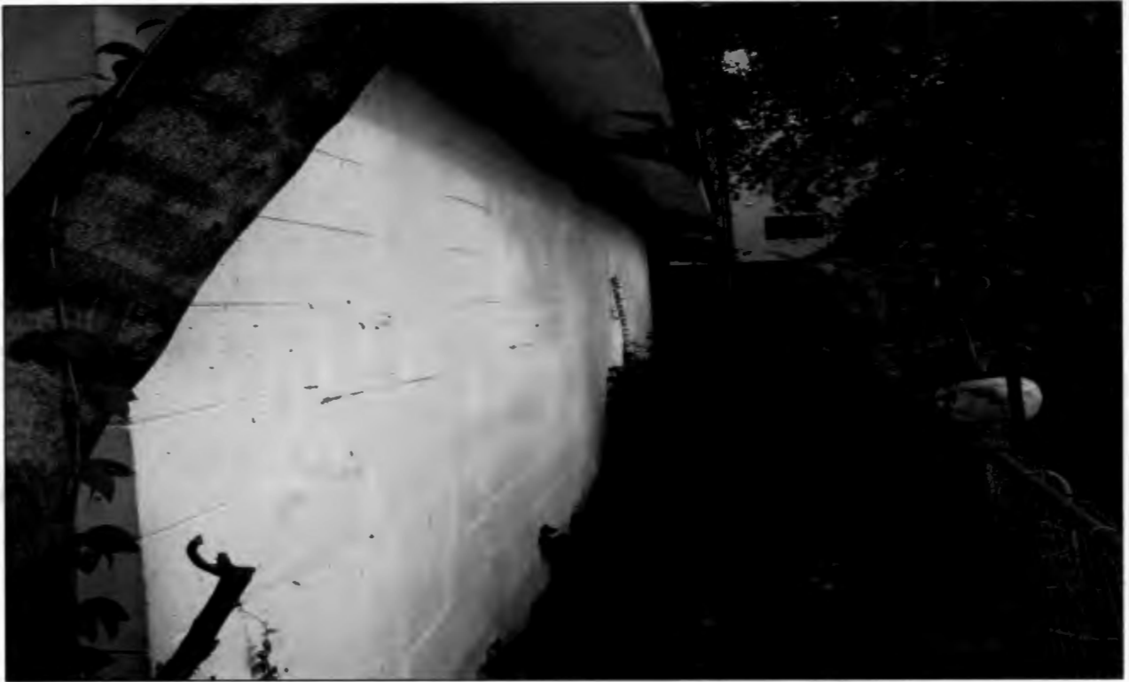
South side of existing structure requiring Variance #4, facing east
