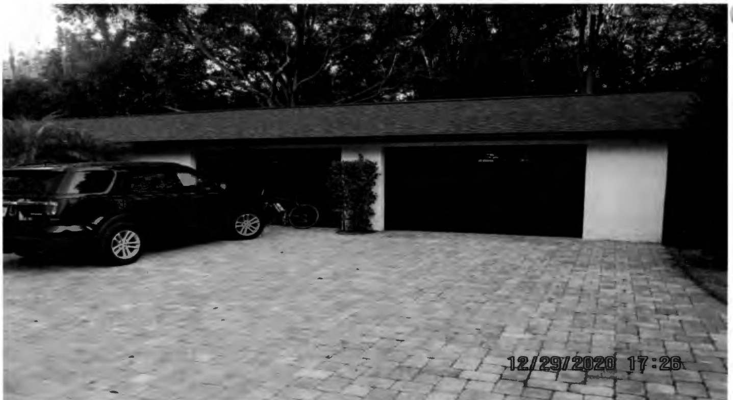
Garage facing south
