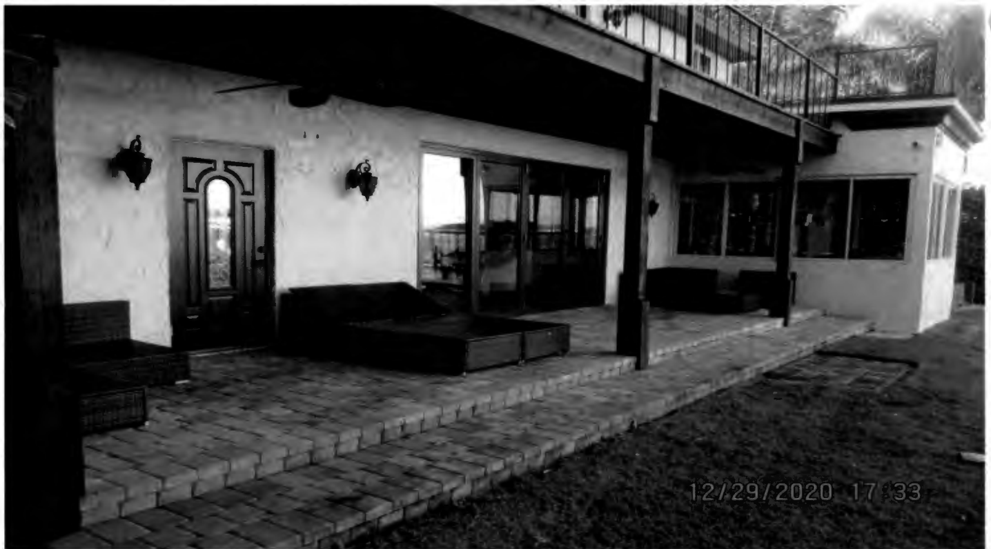
Covered rear deck facing north
