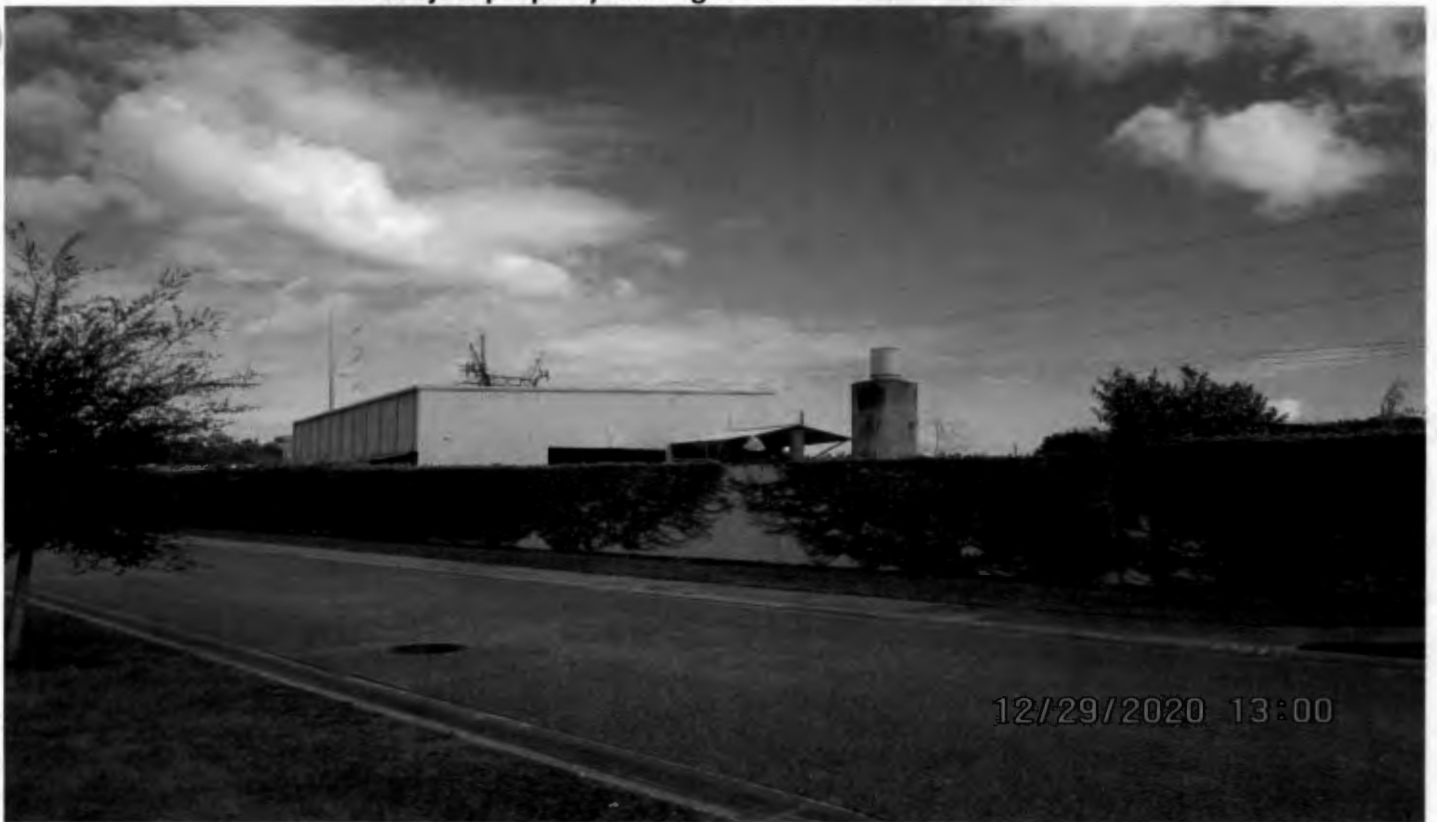
Adjacent commercial looking northeast from Dearmont Ave.
