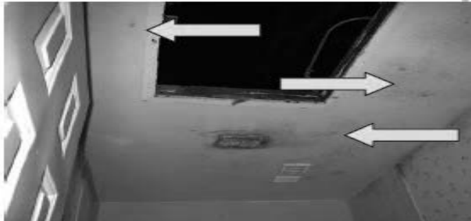
Photo #9 Unit 326: Fungus growth on the ceiling of the 2 nd floor bathroom.
