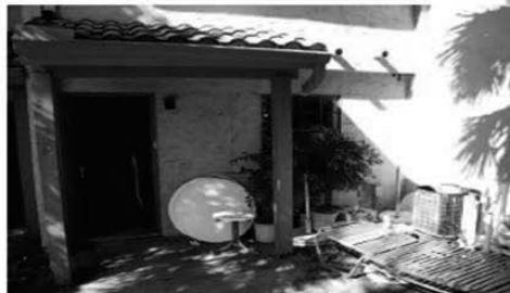
Photo #15 Unit 329: Front entrance. Missing gutter downspout. Broken front window. AC not useable.
