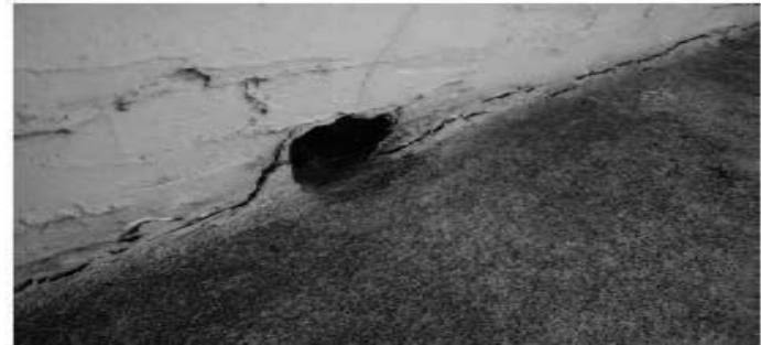
Photo #8 Unit 326: Evidence of cracking at the balcony deck-to-wall area.
