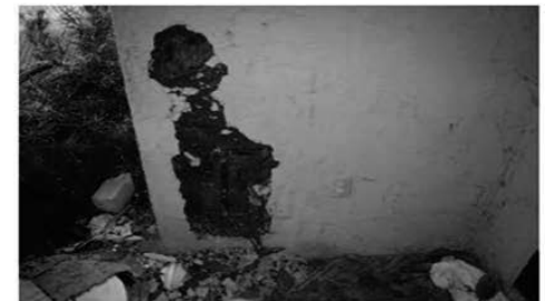
Photo #18 Unit 329: Probable repair at copper piping near hose bibb at rear patio. Damaged structural studs.
