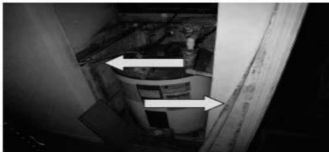
Photo #11 Unit 326: Typical water heater in typical AHU/WH closet. Notice mold on interior of closet and underneath wallpaper on exterior. Typical.
