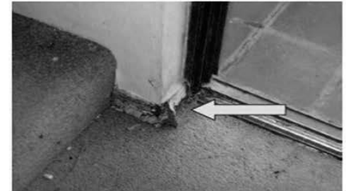
Photo #14 Unit 326: Damage to base of wall at rear sliding-glass door. Rust and fungus growth visible.
