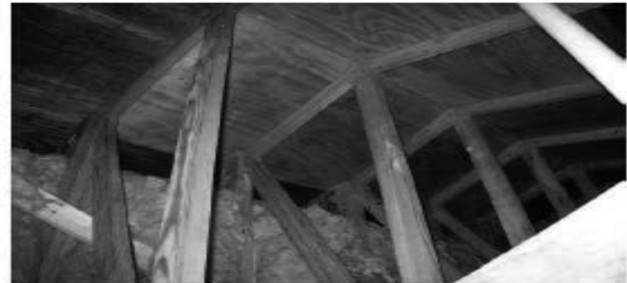
Photo #10 Unit 326: Typical attic construction. No ridge vent observed. Insulation typically covers soffit vents.
