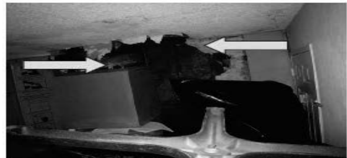
Photo #12 Unit 326: Evidence of wood rot and water infiltration into the first floor bedroom underneath the balcony. Unit used as storage. Typical.
