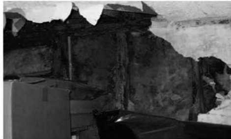
Photo #13 Unit 326: Close-up of previous photo showing extensive structure damage and fungus growth.
